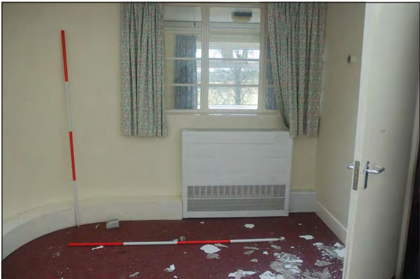
Plate 36: Short Stay Unit (Internal): View southwest of Room G12 detailing current use and original casement window fitting. Formerly a treatment room. Curved floor plan indicates former shape of the southwestern end of the building now disguised by the link corridor (visible through the casement window). Particleboard door in use rather than original panelled door seen elsewhere within the structure as room size was reduced and a new partition fitted. (Scales: 2 x 2.0m)
