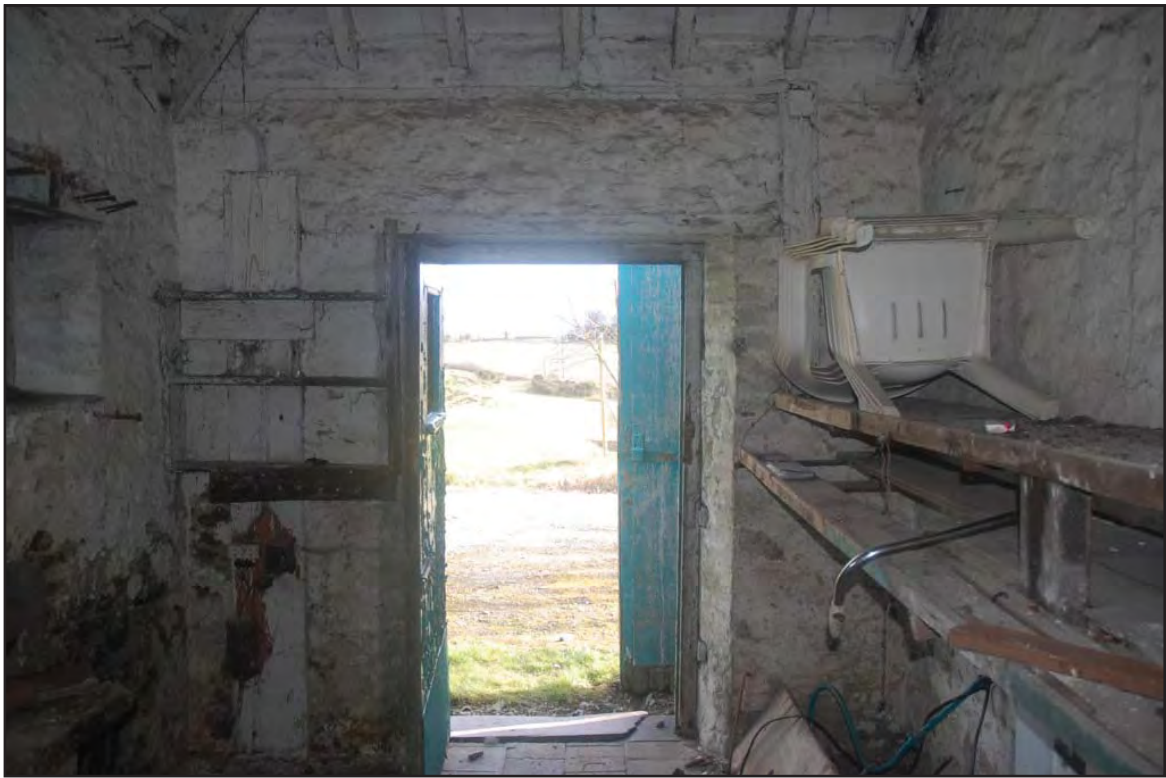
Plate 55: Garage (Internal): View south of side entrance room (cf. external view Plate 50) detailing interior finish and usage. Roughcast walls, whitewashed and exposed rafters visible. Various fittings also present facilitating it's use as a store.
