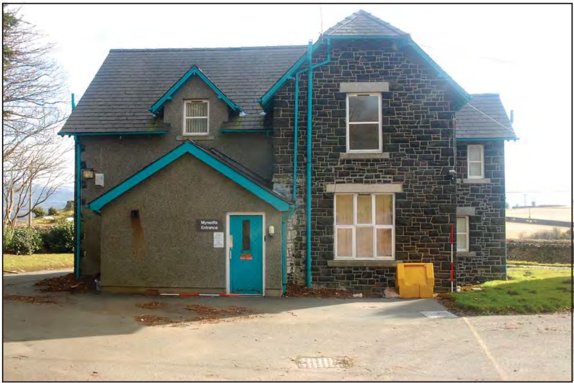
Plate 43: Administration Block: Northwest facing elevation detailing ground floor Room G04 and first floor Rooms F03 to F05. The rear of the property was altered c.1991, with the removal of a ground floor wing that included a kitchen, prep room and store. The kitchen was reduced in size to create the pebbledashed gabled main entrance/photocopy room visible in the image. Remnants of the alteration work can be seen where the main entrance is keyed into the original build. (Scales: 2 x 2.0m)
