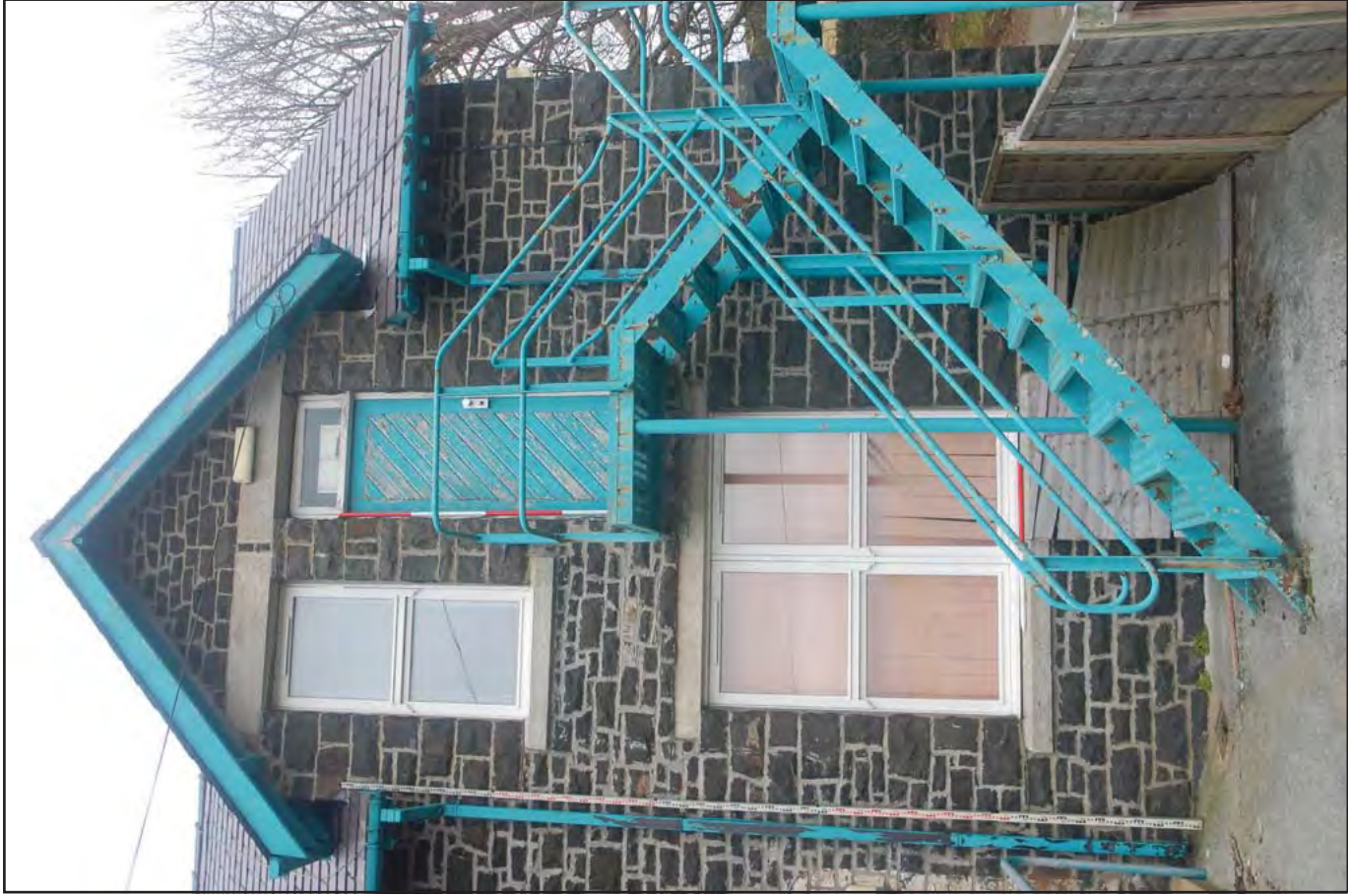
Plate 41: Administration Block: Southeast facing elevation. Ground floor Room G02 and first floor Room F04 are visible; Room F04 includes a fire exit, which is a converted window space. Stone voussoirs and sills in use. Original main entrance (cf. Plate 42) is to left of image (out of shot). Scales: 2 x 2.0m and 1 x 5.0m.
