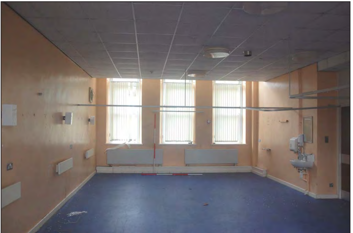
Plate 16: Long Stay Unit (Internal): Room G11 - view southeast of former female ward, detailing window fittings and bullnose skirtings. Original ceiling is disguised by a suspended ceiling (Scales: 2 x 2.0m)
