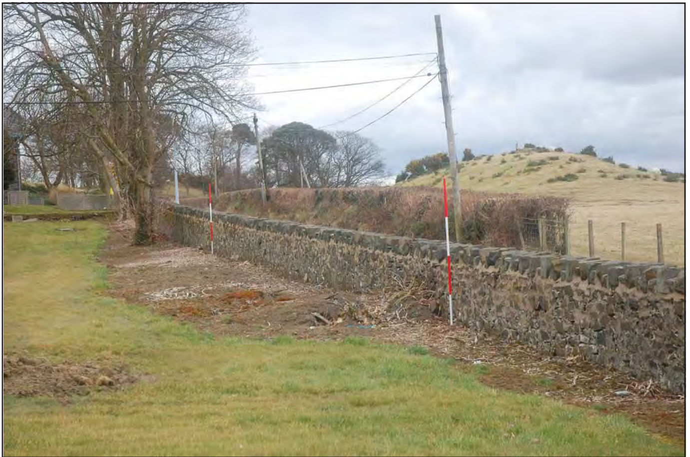
Plate 63: Boundary Wall - view south of portion running parallel to Hendrewen Road. Built from irregular shaped stone with a crenellated surmount. (Scale: 1 x 2.0m)
