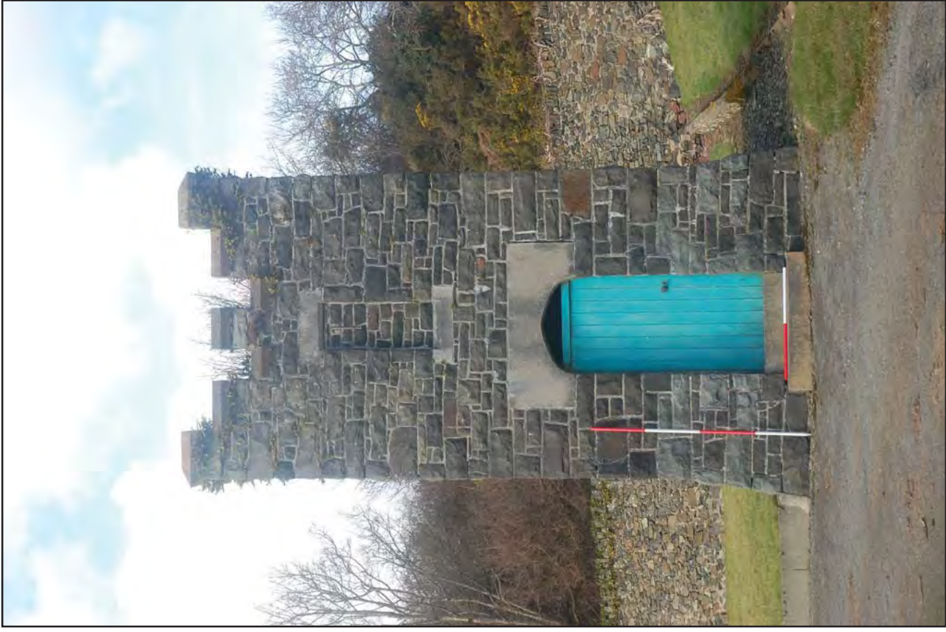
Plate 52: Water Tower - Southeast facing elevation detailing construction form, including crenellated capping, internal buttress and main entrance via pannelled door. Note the boundary wall at rear of image (Scales: 2 x 2.0m).
