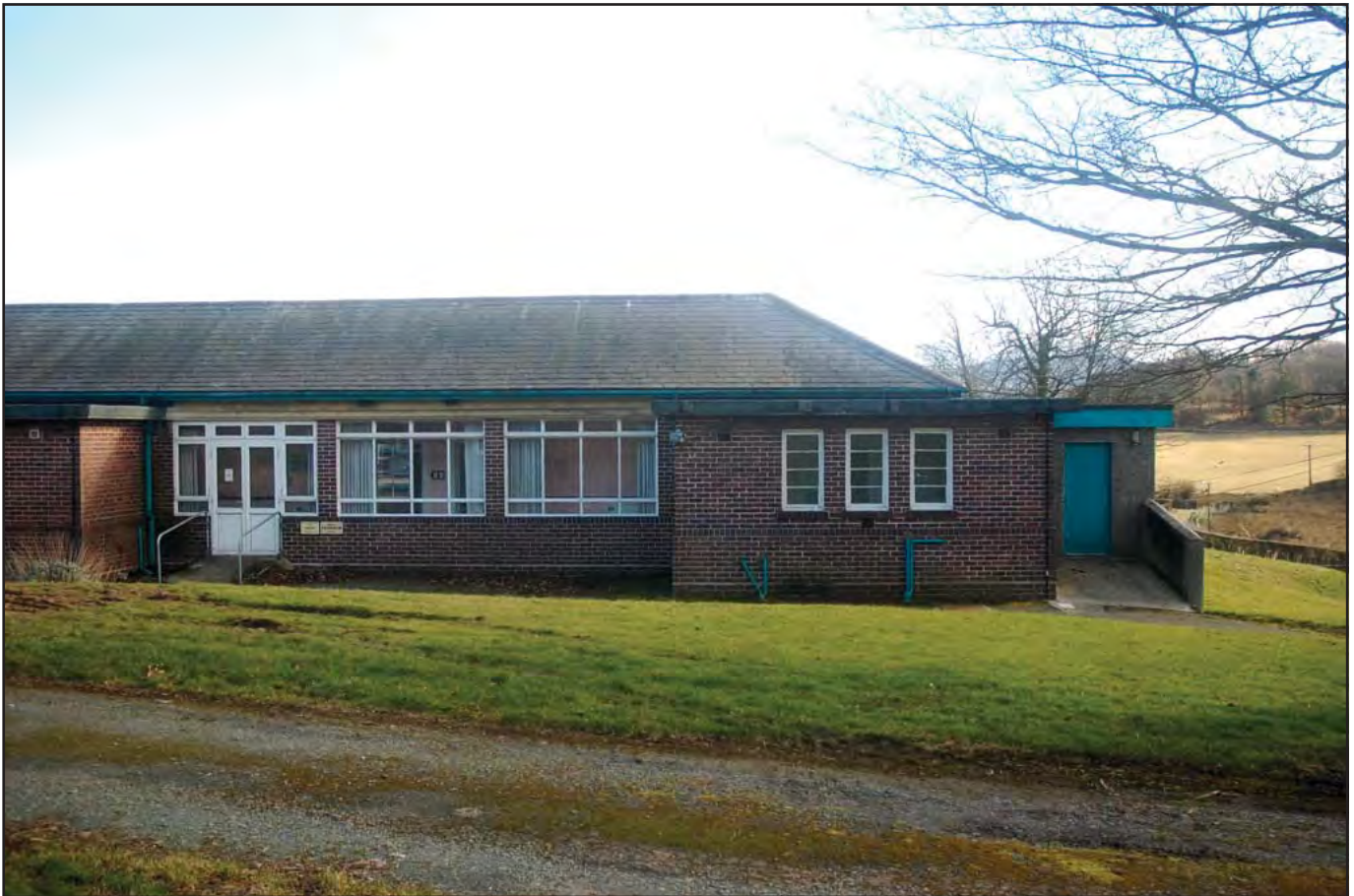
Plate 24: Short Stay Unit: Northwest facing elevation - main entrance and Room G11 (Kitchen); detailing English Garden Wall bond brick style and casement windows. Note the link corridor attached to the southwest facing elevation towards right of image
