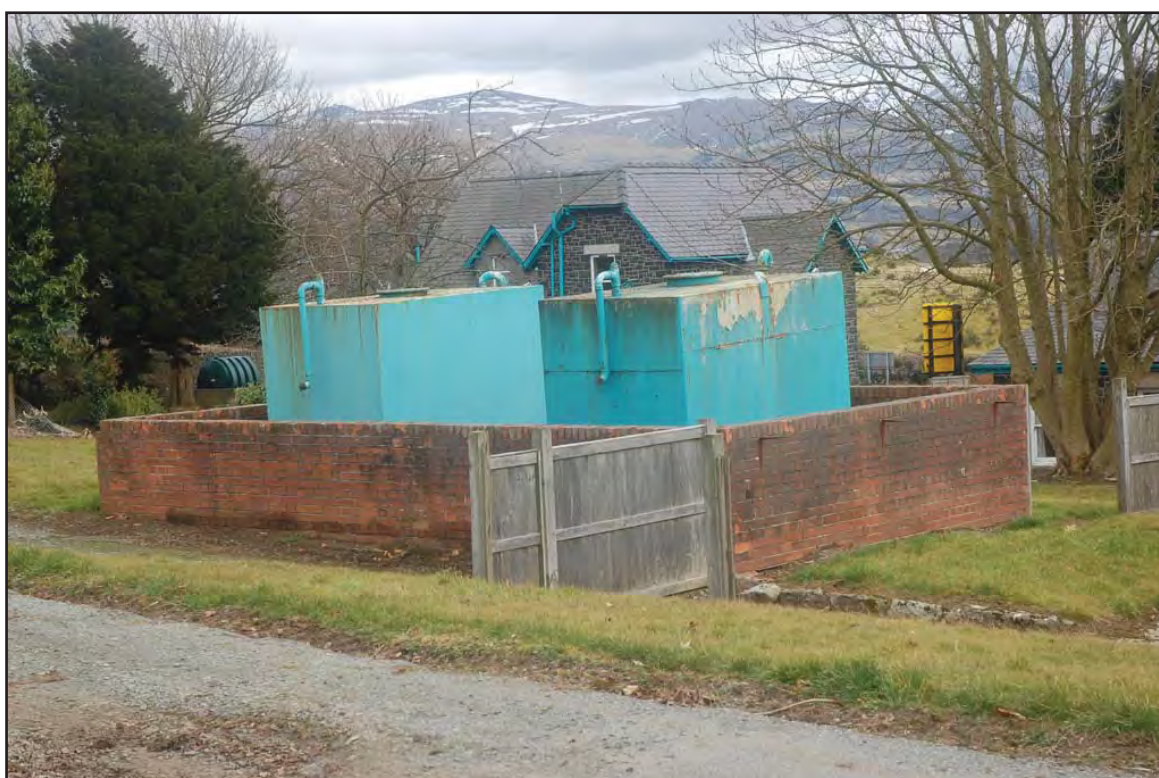
Plate 62: Oil Tanks: View southeast of oil tanks located towards rear of property. Enclosed by a low brick wall (Dearnies/Rat trap Bond). Accessed via site road that links all buildings within complex. Note administration block towards centre of image and views from the hospital site towards Snowdownia.
