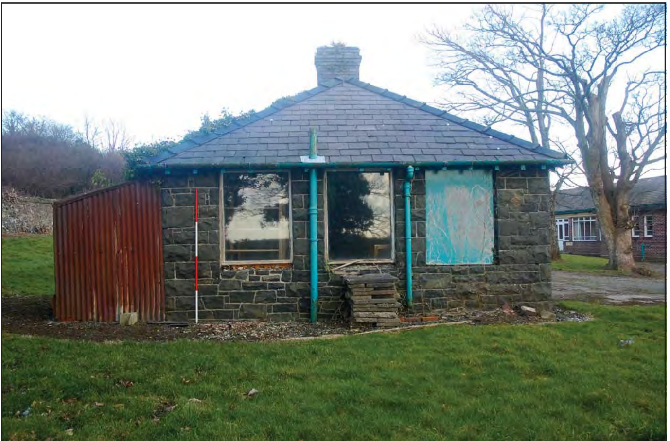
Plate 54: Garage - Southwest facing elevation detailing three fixed windows, hip gable roof and brick built chimney. The corrugated lean to is a later addition (Scale 1 x 2.0m)
