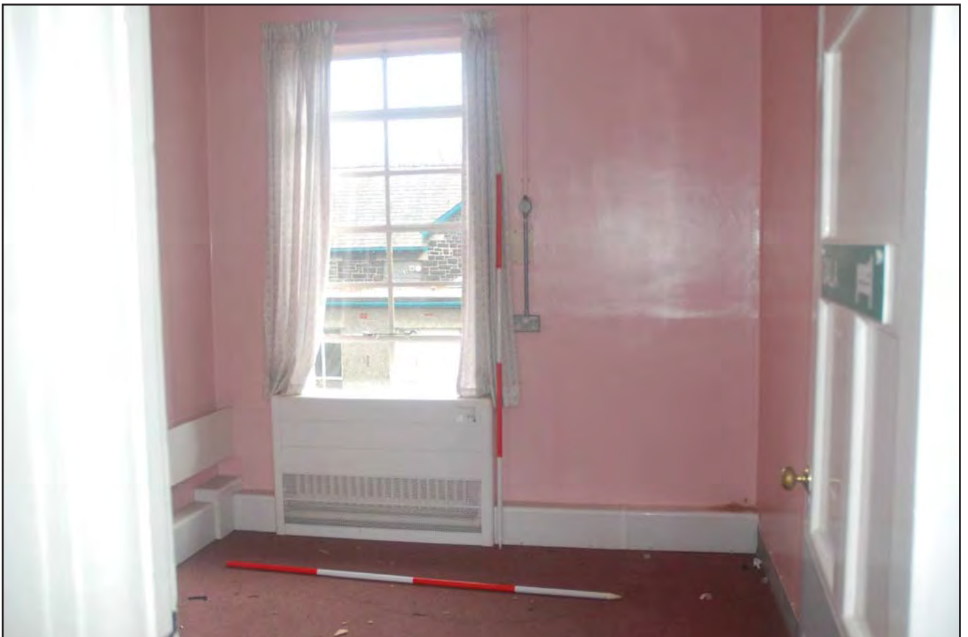
Plate 32: Short Stay Unit (Internal): View southeast of Room G08 detailing current use as a ward. Storage heater visible below original casement window, with boxed in plumbing. Panelled and moulded entrance door visible in image foreground. Rear of Long Stay Unit through window (Scales: 2 x 2.0m)
