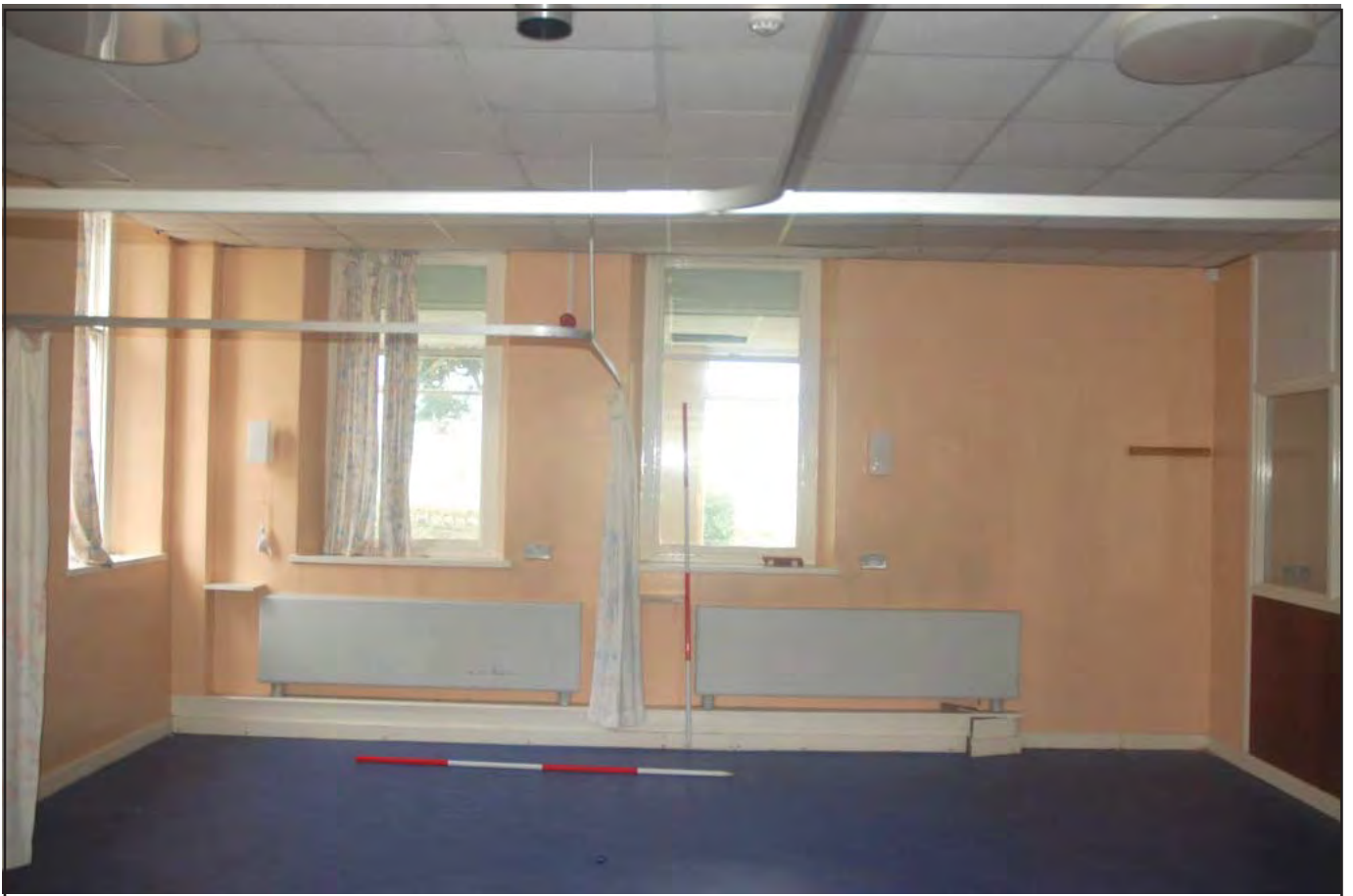
Plate 17: Long Stay Unit (Internal): Room G12 - view southeast of former female ward annexe. This room was created from the conversion and alteration of the former sewing, treatment and linen rooms into one room; therefore, most of the original internal structural elements have been altered and/or disguised. A suspended ceiling is in place and the screen separating Rooms G12 & G11 can be seen to the right of the image (Scales: 2 x 2.0m)
