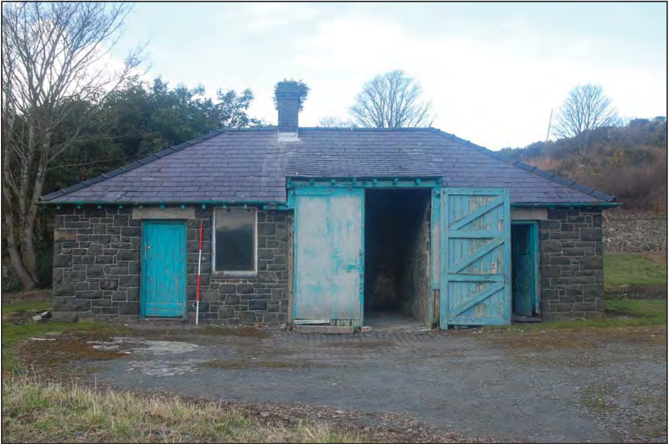
Plate 53: Garage - Southeast facing elevation; detailing main entrance via large panel and brace doors and two side entrances. Part of the original construction phase along with Long Stay Unit, Water Tower and Administration Block, with similar building detail including sub-rectangular stonework, stone lintel and quoin edging. (Scale: 1 x 2.0m)
