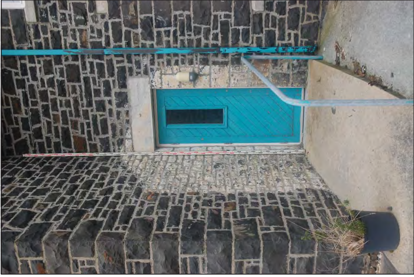
Plate 42: Administration Block: Southeast facing elevation. Ground floor former main entrance (now a fire exit) with a panelled door. Original porch has been removed, but outline is still visible. (Scale 1 x 5.0m).
