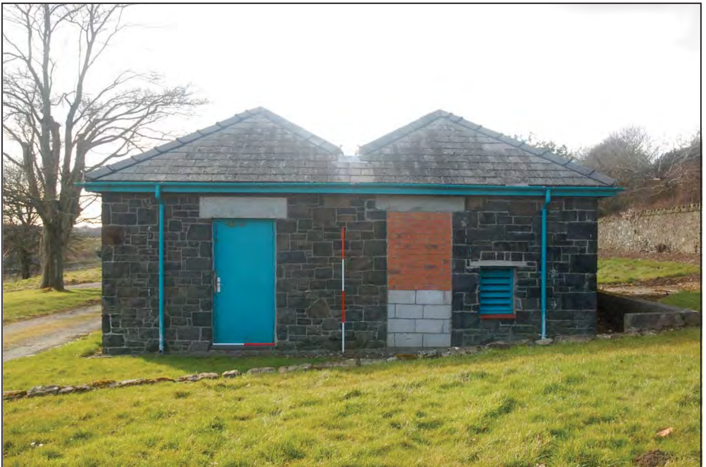
Plate 58: Generator Room: Southeast facing elevation detailing side entrance (blue door) and blocked entrance next to louvered vent. Double hip gable roof. The generator room was built between 1900 and 1914. The extension is indicated where the gables meet in the middle. (Scale: 1 x 2.0m; 1 x 1.0m)
