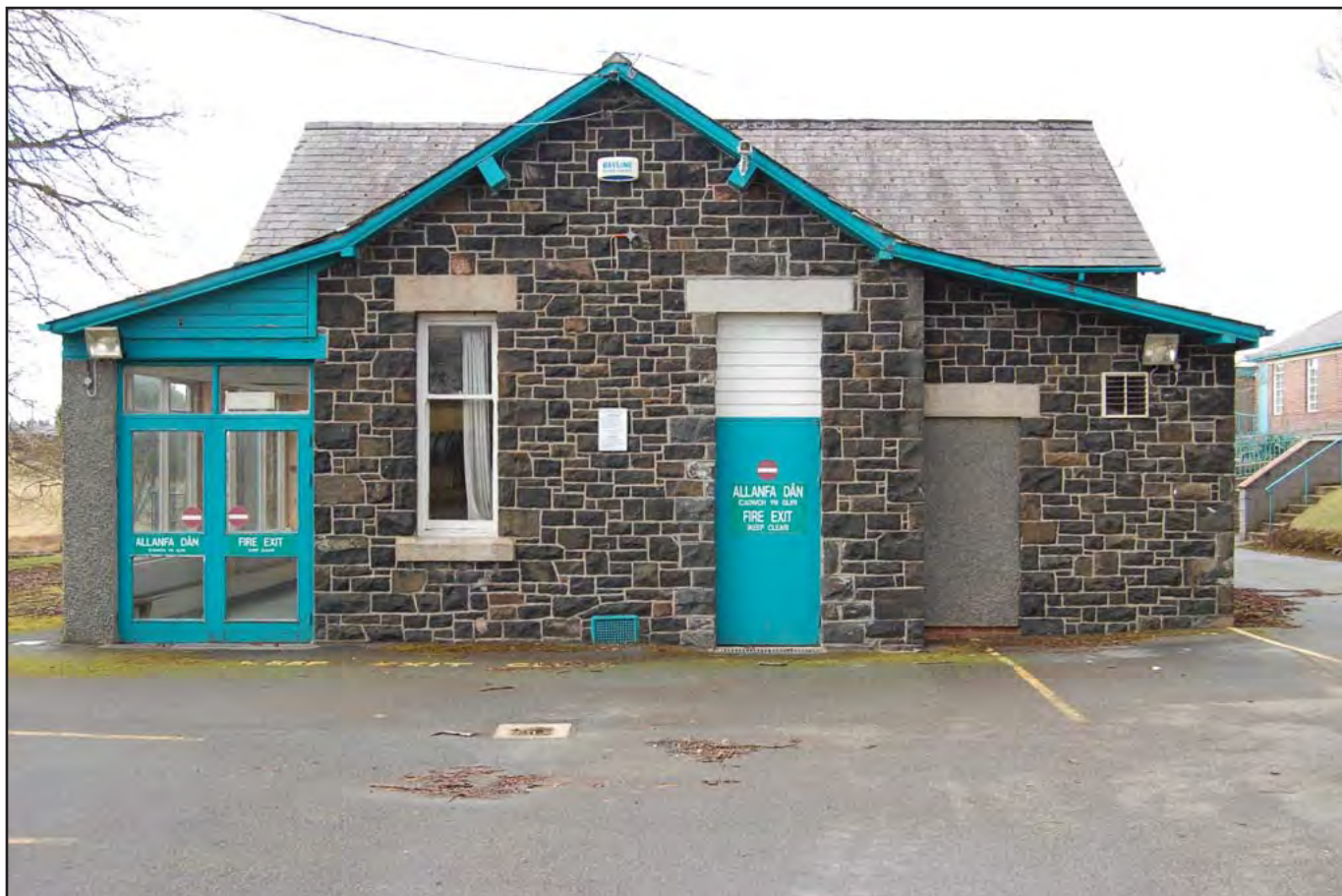
Plate 07: Long Stay Unit (External): Northeast facing elevation of early twentieth extension (Room G12), detailing the use of sub-rectangular stonework and quoin edging. The roof of the female wing (Room G11) is in the background.
