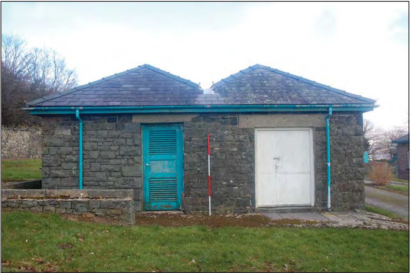
Plate 57: Generator Room: Northwest facing elevation detailing main entrance (large door) and louvered entrance. Double hip gable roof. The generator room was built between 1900 and 1914. An extension was later added, indicated by where the gables meet in the middle. The stonework on the left side of image is slightly different in appearance to the right side, indicating the extended portion. (Scale: 1 x 2.0m)
