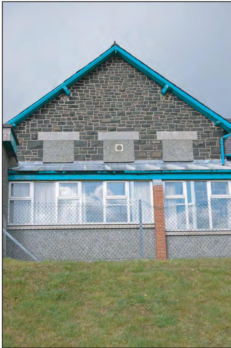
Plate 05: Long Stay Unit (External): Southeast facing elevation detailing late twentieth century veranda extension to the original structure (Rooms G03 and G07). The gable end of the male wing (Room G01) is also visible, detailing original structural style and blocked windows.
