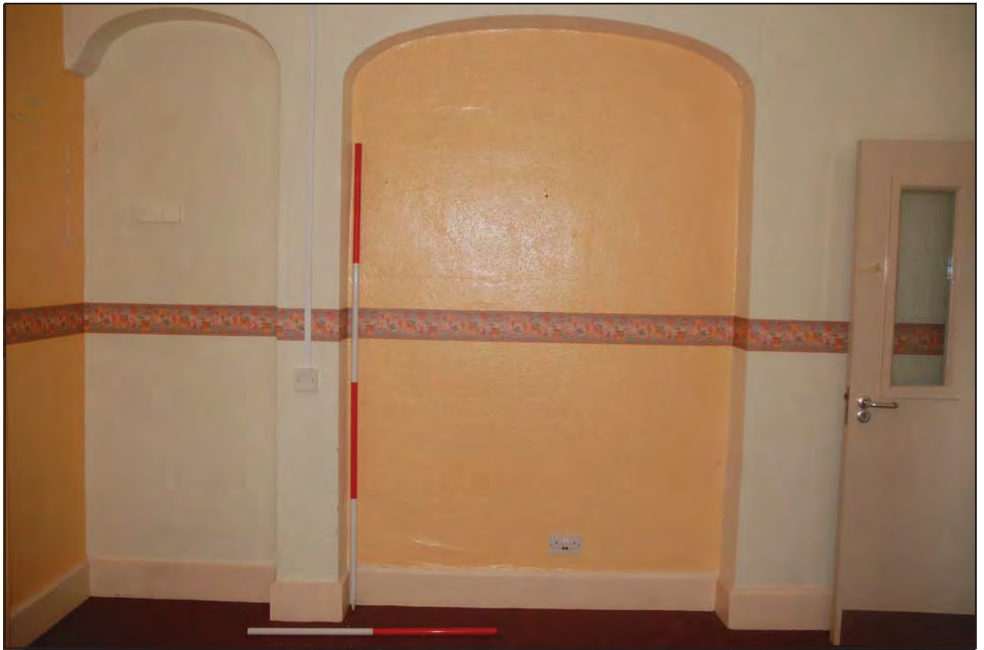
Plate 47: Administration Block (Internal): View northeast of former matron's office (Room G03) detailing redundant archways and modern fire door. Scales: 1 x 2.0m and 1 x 1.0m.
