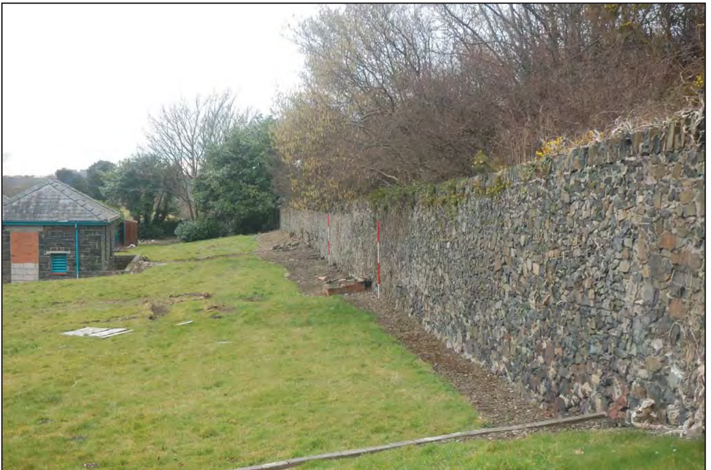
Plate 66: Boundary Wall - View west of rear portion, detailing construction (irregular stones and crenellated surmount) and height (2.50m max). Note the generator in image left and gravel path running along the base of the wall. (Scale: 2 x 2.0m)
