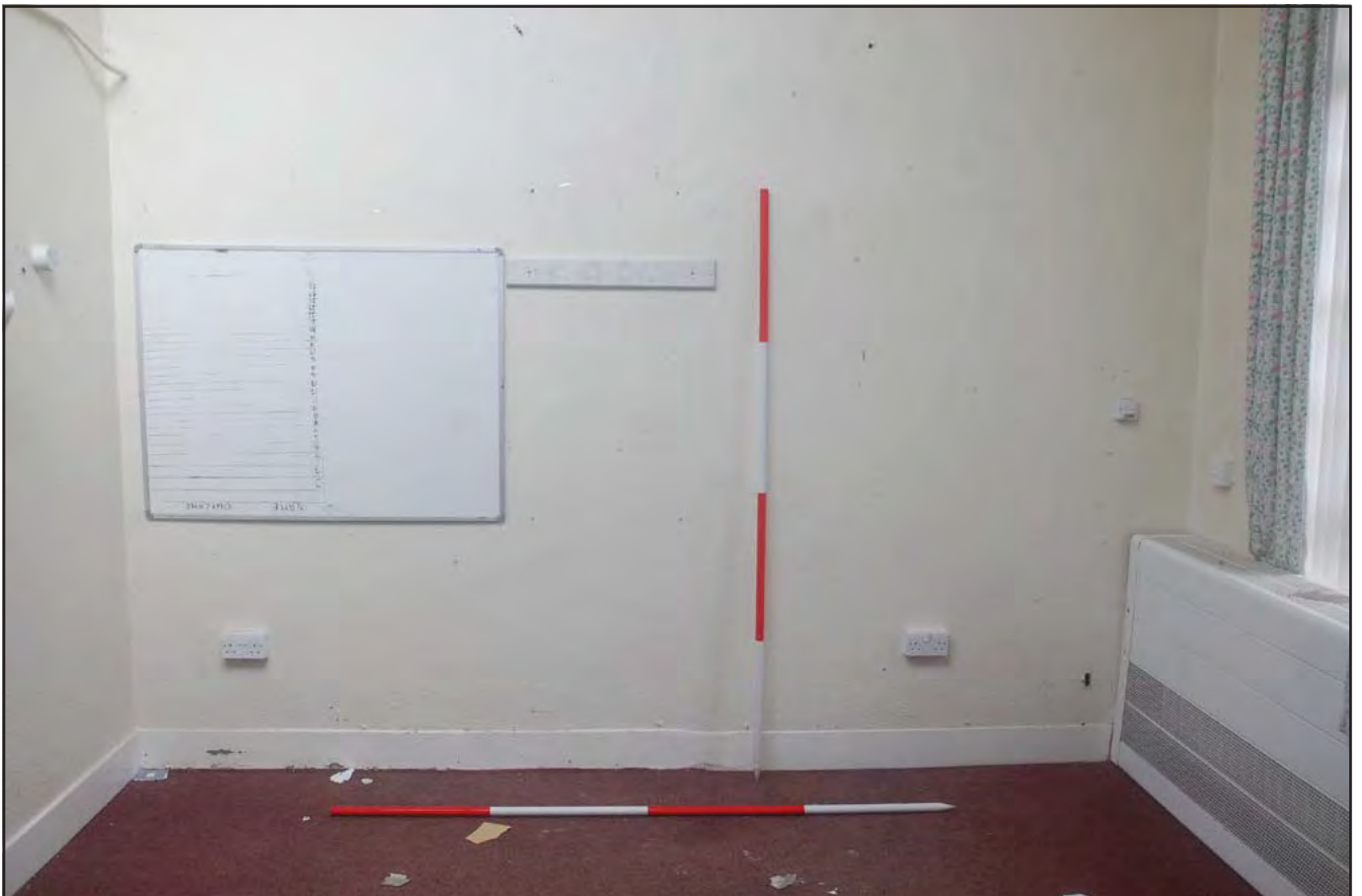
Plate 34: Short Stay Unit (Internal): View east of Room G10 detailing current use. Storage heater visible below original casement window, bullnose skirtings extant. (Scales: 2 x 2.0m)
