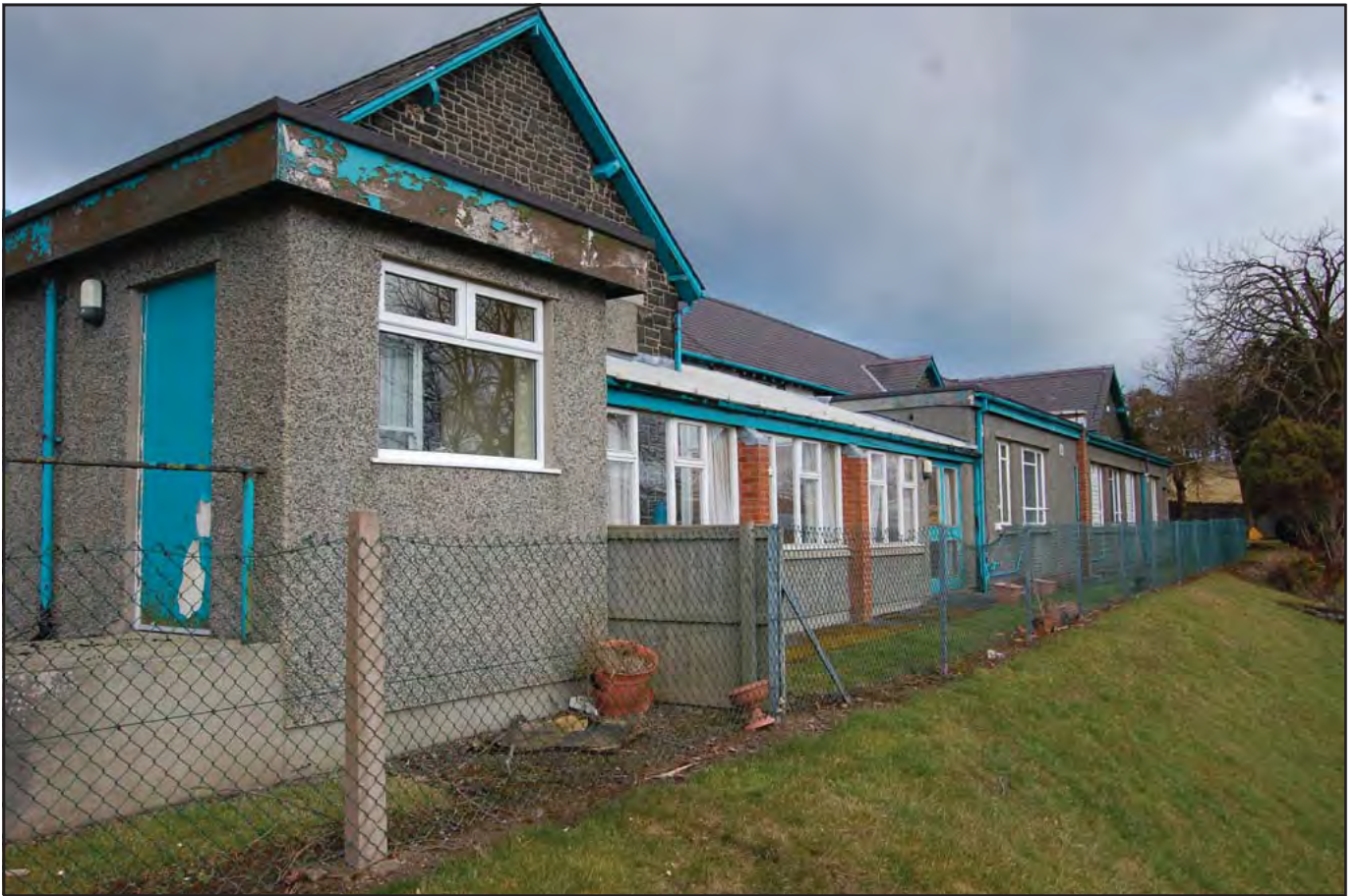
Plate 03: Long Stay Unit (External): Southeast facing elevation detailing late twentieth century veranda extension and flat roof extensions to the original structure. The Link Corridor is in the left foreground of image. The gable end of the male wing is also visible in the foreground, detailing original structural style.
