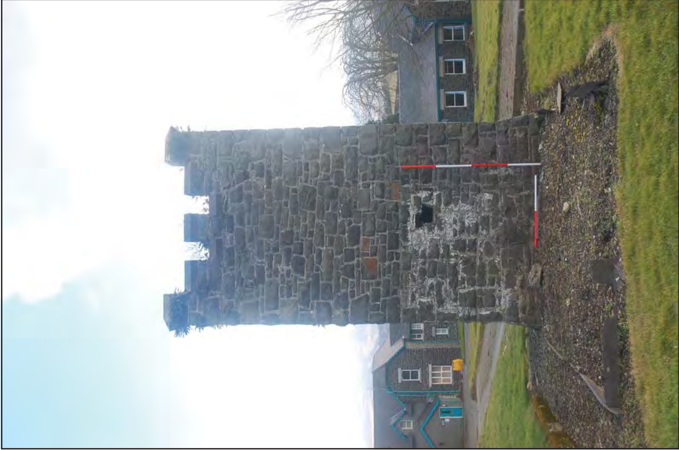
Plate 51: Water Tower - Northwest facing elevation detailing construction form, including crenellated capping and an internal buttress. Note the external slate defined area that appears to have functioned as a possible small garden area; note also the administration block in the left background and the Long Stay Unit in the right background (Scales: 2 x 2.0m).
