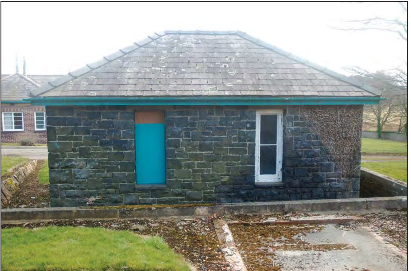
Plate 60: Generator Room: Northwest facing elevation detailing rear. This elevation represents the post-1914 extension, which has been benched into the slope. A later external platform has been built (bottom right of image), with brick surround that may have supported an upstanding piece of equipment. Note the rear of the Short Stay Unit to centre left of image.
