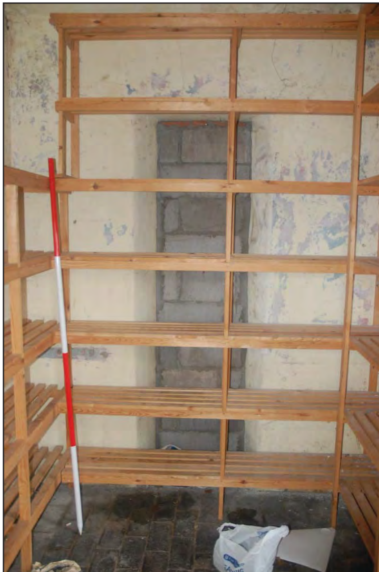
Plate 61: Generator Room (Internal) - View northeast of interior room, detailing decor and usage. Interior view of extension room. Note blocked window, visible from the outside in Plate 59. The floors are quarry tiles; the walls are rendered. Wooden shelving throughout room. (Scale: 1 x 2.0m)
