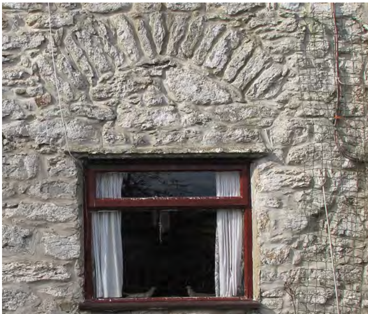
window of main room, south side, with relieving arch
