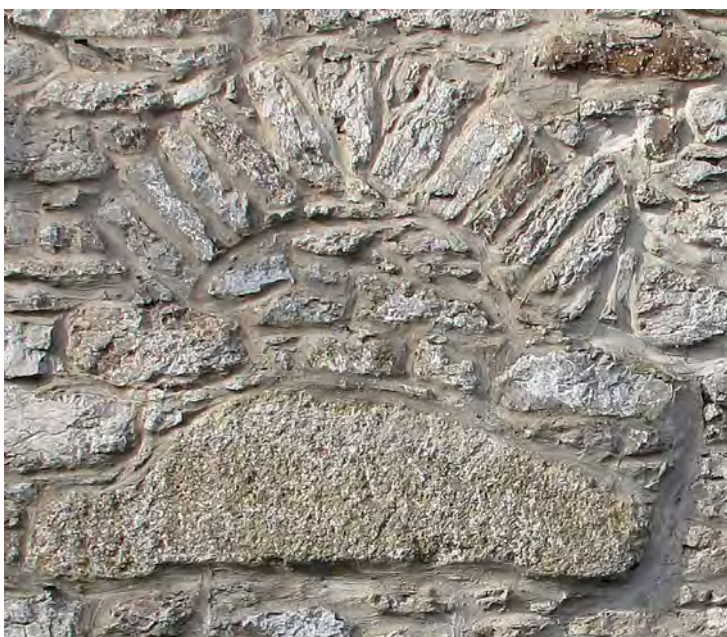
Lintel of blocked window, south side, west end, with relieving arch
