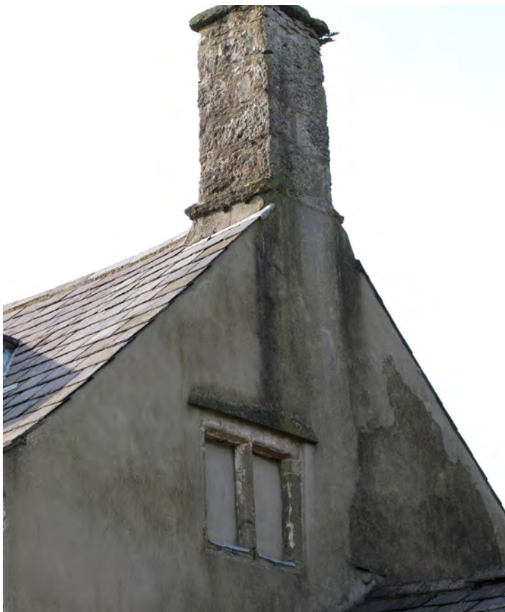
First floor blocked original gable window
