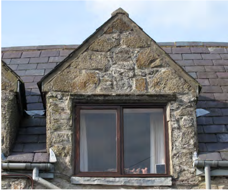
Middle dormer showing fragmentary jambs and cavetto moulding
