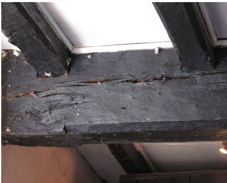
Beam in main room, chamfer stop; joists in beam sockets, chamfered with run-out stops
