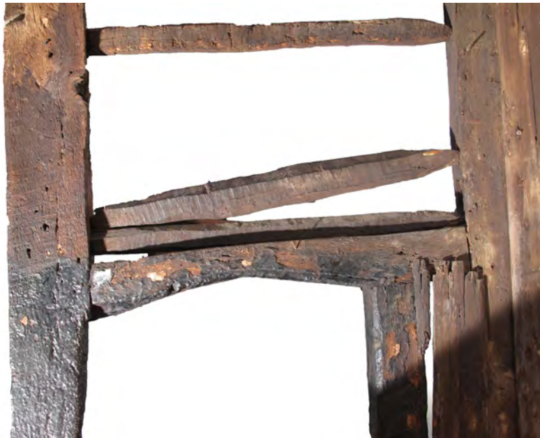
ground floor partition; false four-centred door head; staves for wattle and daub
