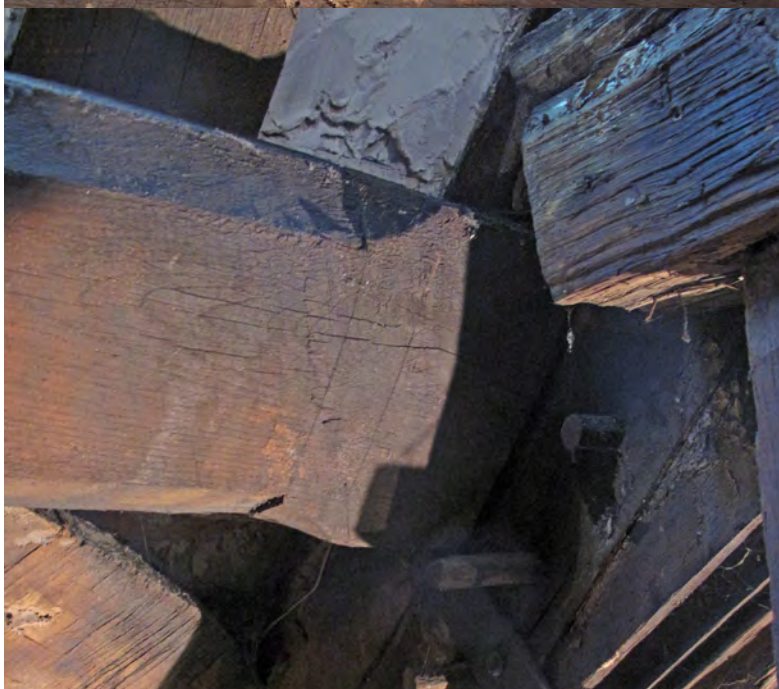
chamfered purlin at truss 3: carpenter's marks
