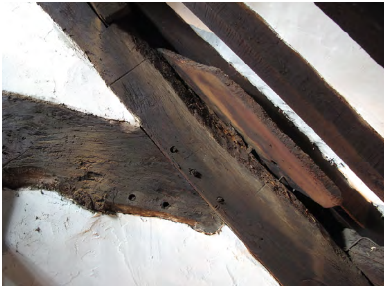
Truss 4: carpenter's marks on principal
