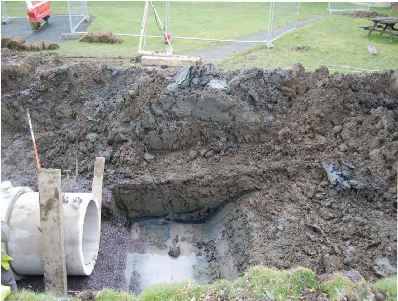
Plate 10 , Section of Pipe Trench in Park
