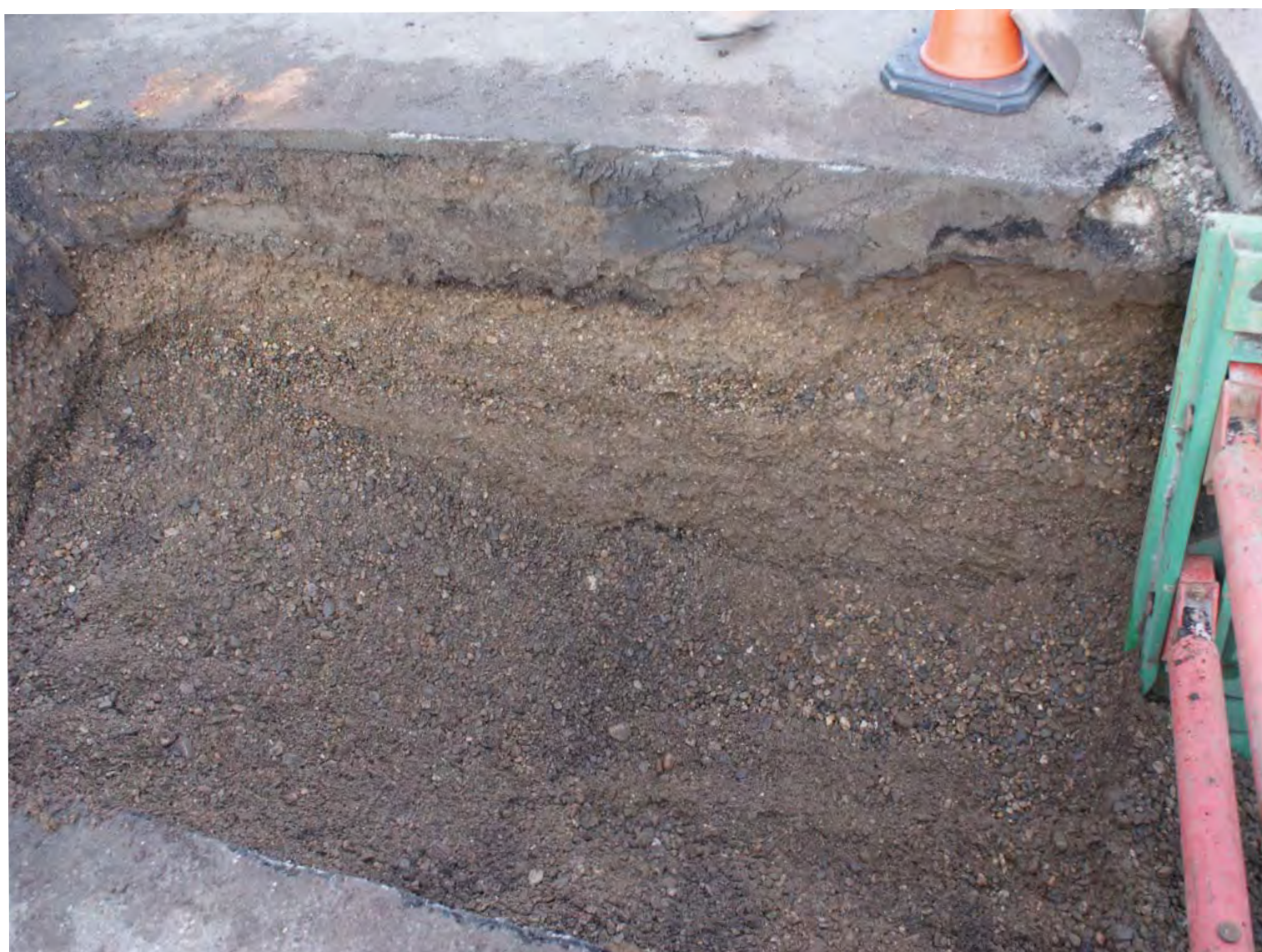
Plate 4, SE Trench edgeshowing Sand & Gravel
