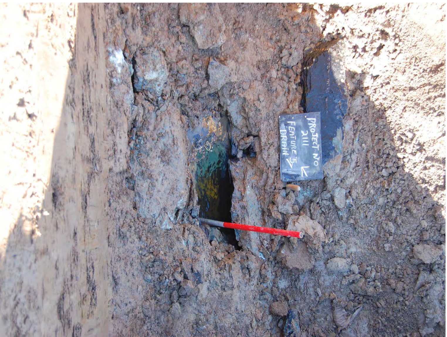
Plate 13, Stone Built Culvert
