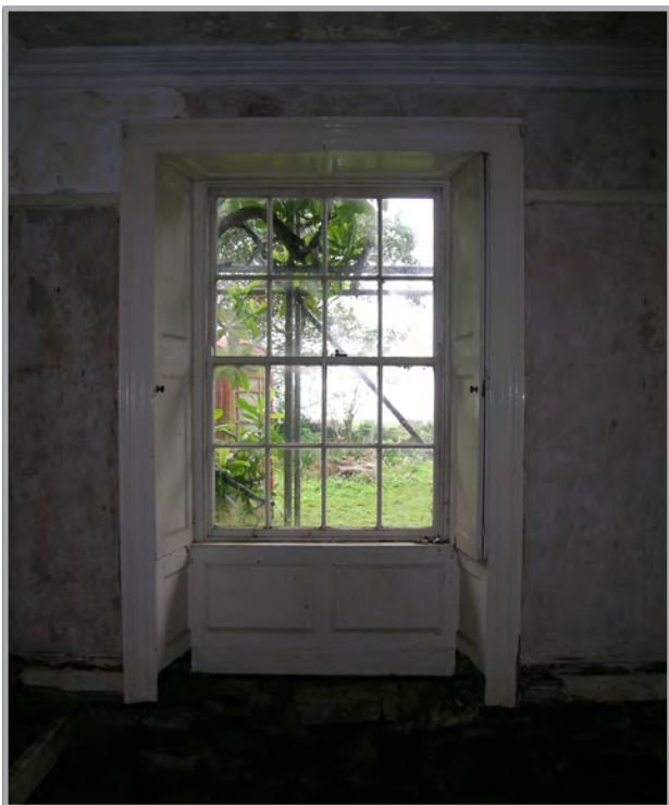
Plate 15: Sash windows and panelled shutters in the parlour wing
