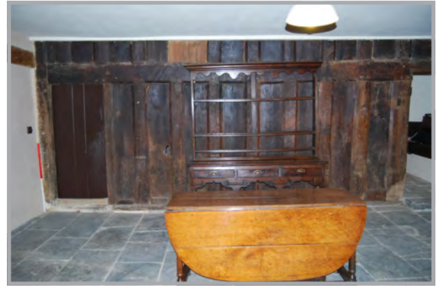
Plate 25: The dais partition on the ground floor facing the hall
