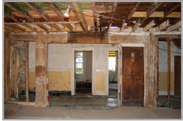
Plate 21: The aisle truss ground floor looking west. The two aisle posts are linked by a later horizontal timber at ceiling height
