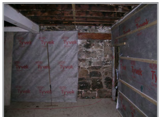
Plate 38: Blocked window in north wall of hall
