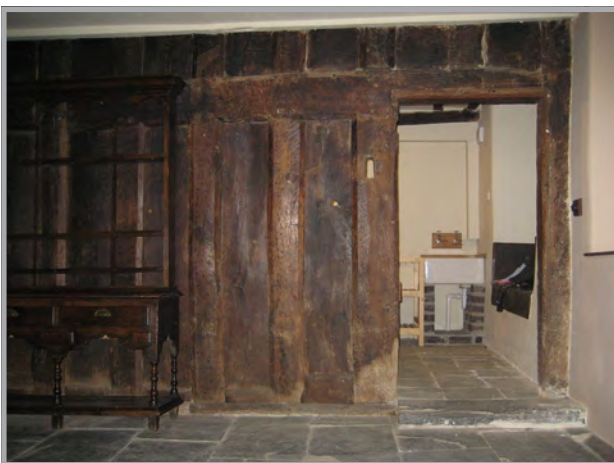
Plate 30: The dais partition ground floor south door
