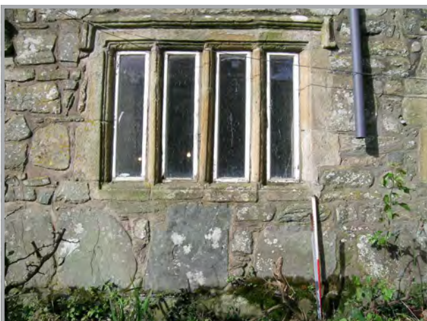
Plate 5: Ovolo moulded windows on the south side of the hall
