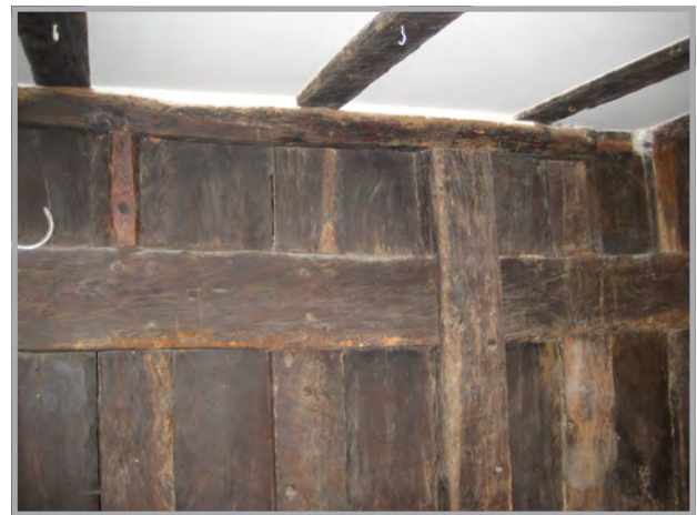
Plate 31: The dais partition ground floor inner room. The vertical upright supports the plate for the joists
