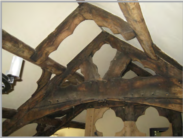
Plate 34: The louvre truss and arch-braced collar beam truss with decorative cusping
