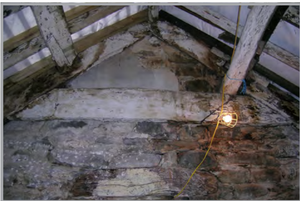
Plate 36: Simple collar beam truss at the east end of the inner room
