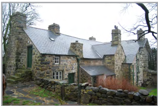
Plate 8: The north elevation
