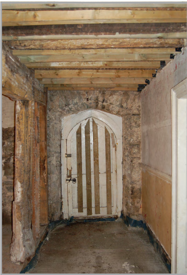
Plate 12: The cross-passage during renovation
