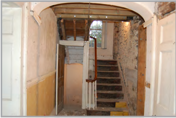
Plate 14: The stairs at the north end of the cross-assage
