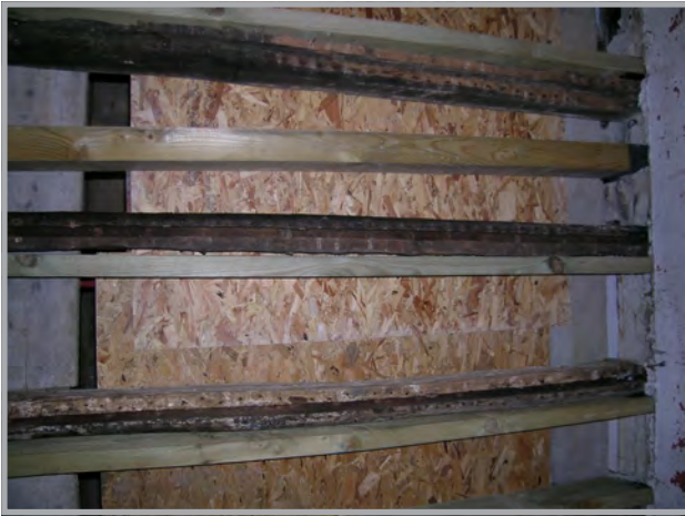
Plate 11: Re-used timbers used as ceiling joists in the cross-passage
