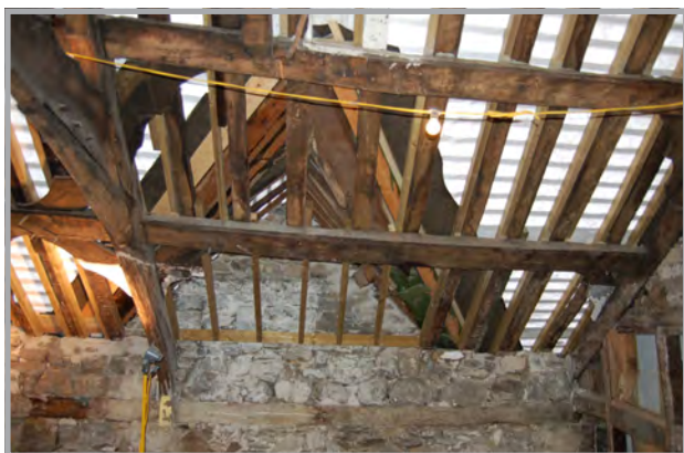
Plate 39: Straight joint in masonry of inner gable of lateral chimney
