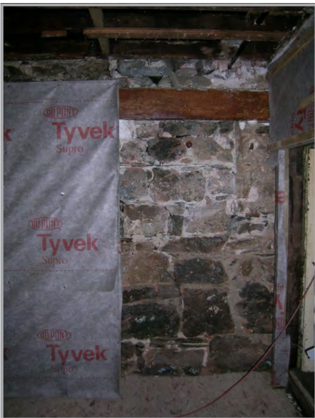
Plate 20: Blocked window in the north wall of the hall
