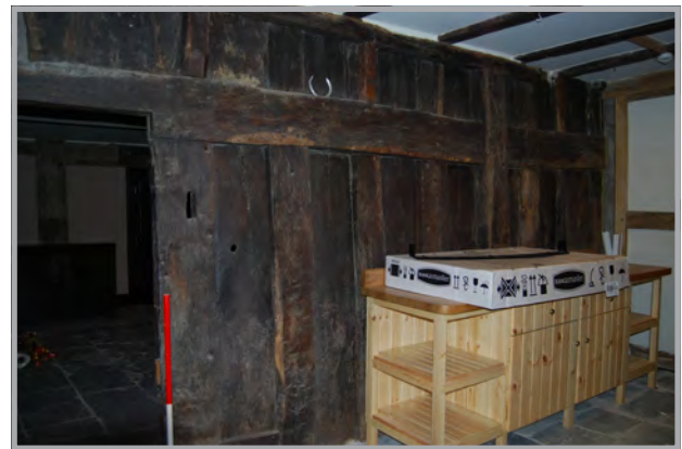
Plate 26: The dais partition ground floor inner room.
