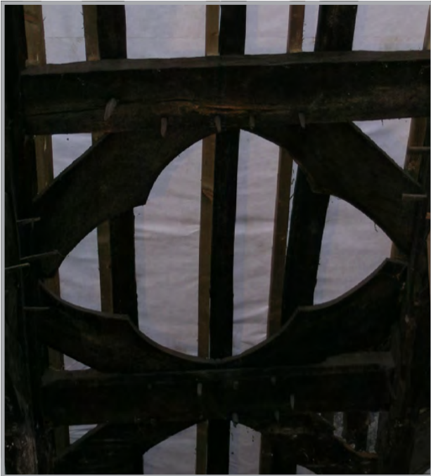
Plate 35: Decorative cusped windbraces
