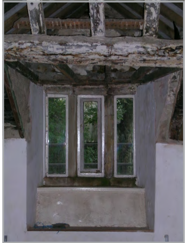
Plate 37: Dormer window in first floor inner room
