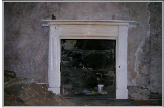
Plate 16: Slate fireplace in the parlour wing
