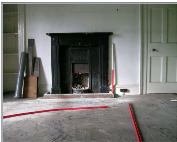
Plate 32: Fireplace with flanking cupboards first floor parlour wing
