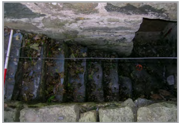
Plate 9: Steps down to basement
