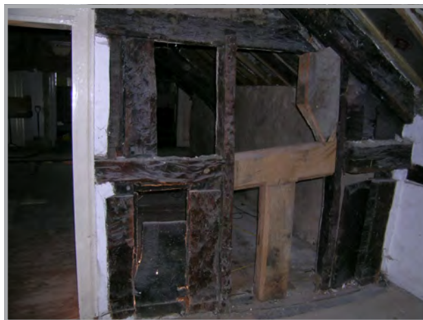
Plate 41: Dais partition first floor inner room. The upper rail and one post has been removed
