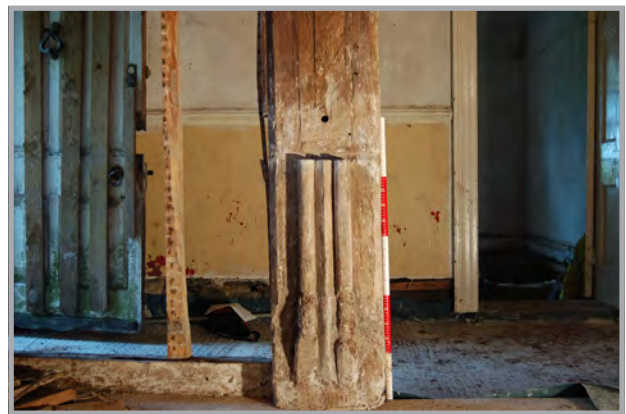
Plate 22: The moulding on the hall side of the south aisle post
