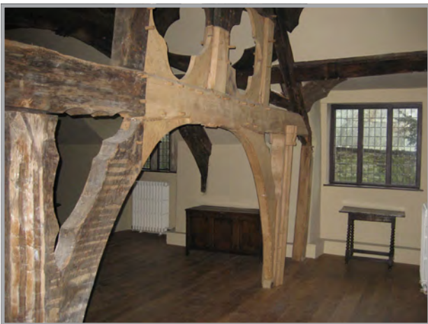
Plate 24: The aisle truss after renovation
