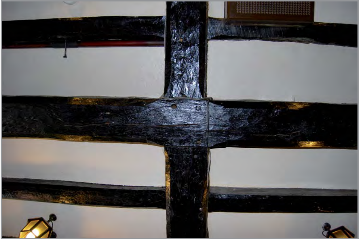
Plate 11: Image showing axial beam and transverse beam
