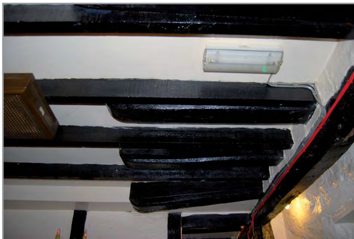
Plate 14: Jetty beams
