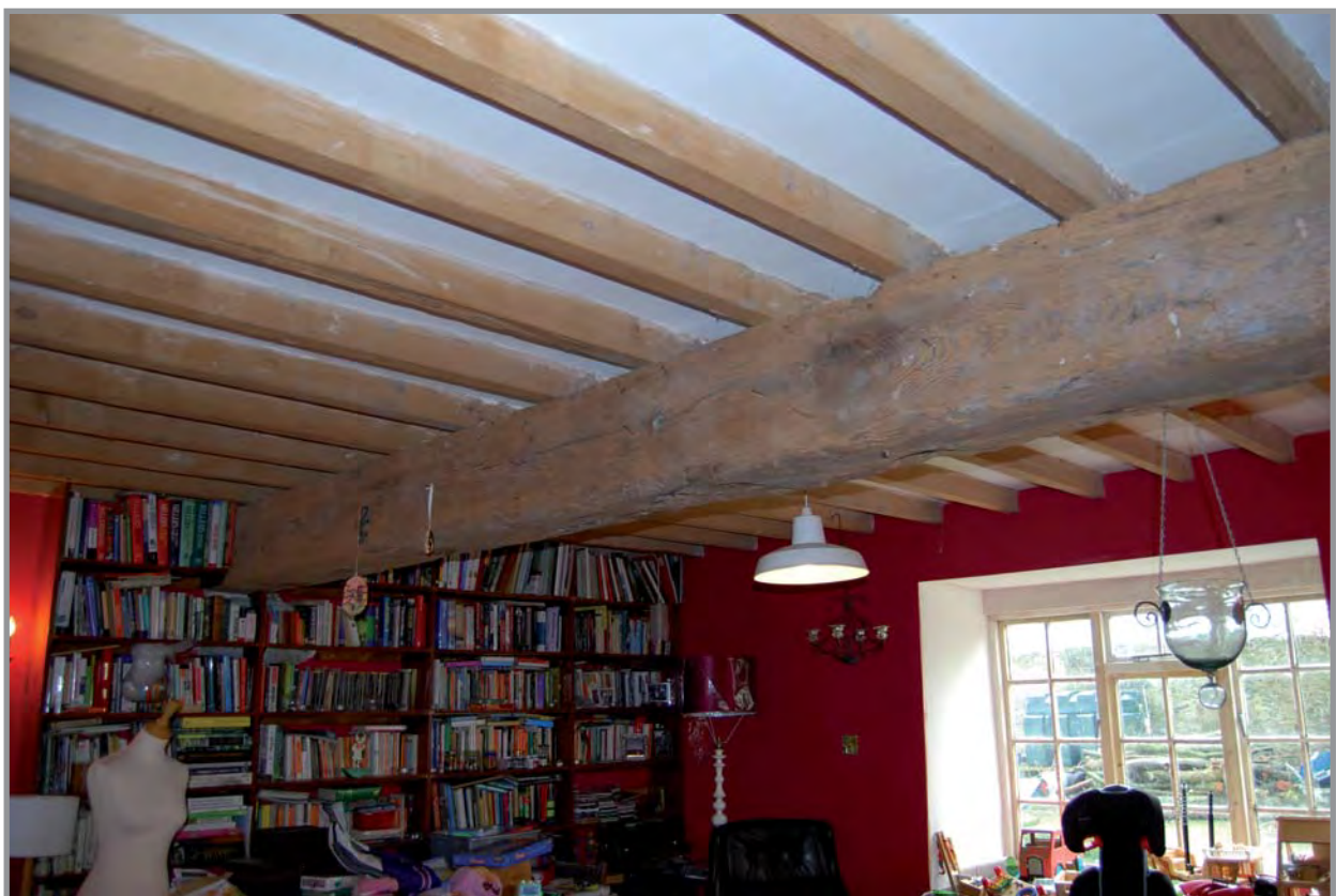
Plate 14: Gronant building B living room facing south west showing the large square axial beam which runs east to west across the entire of building B
