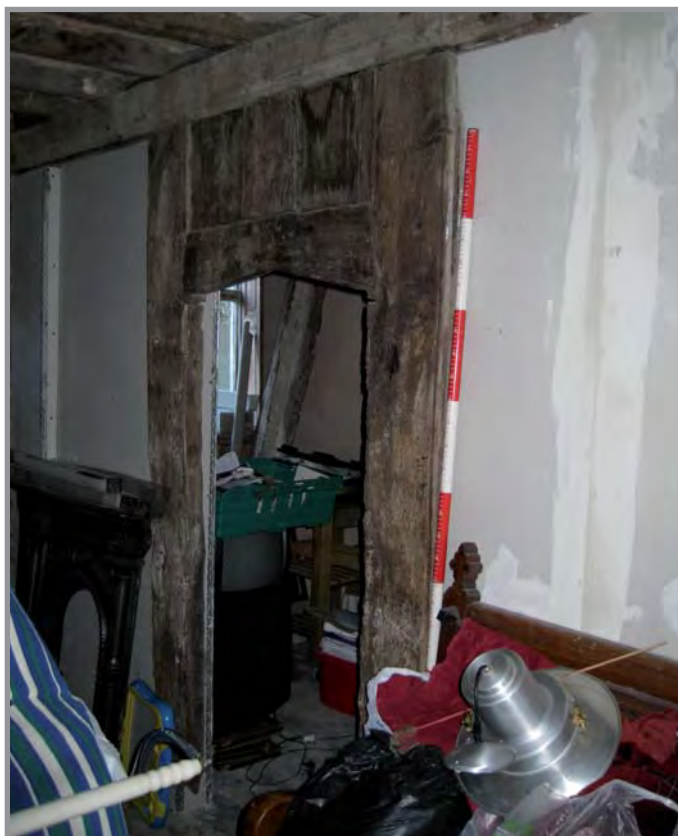
Plate 19: Gronant building A. Post and panel screen
