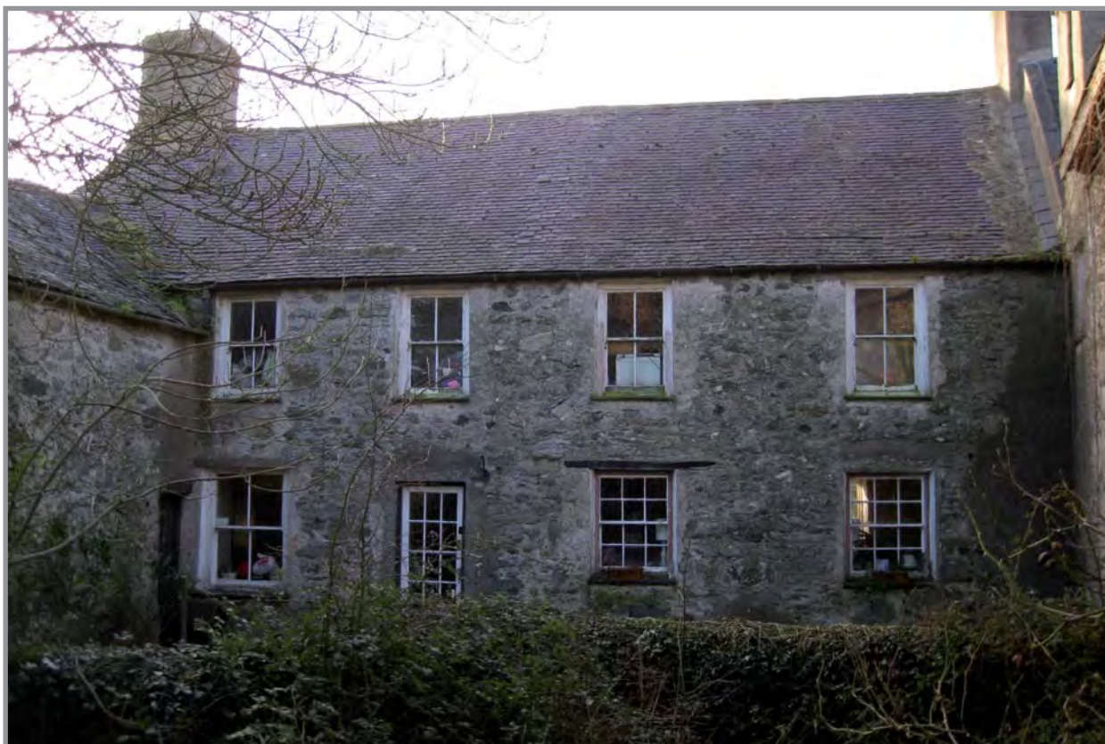
Plate 9: Gronant north facing elevation showing building B with four sash windows on the first floor, two 12-pane windows to the east and a four pane to the west. The change in masonry shows that the window east of the door was once a door
