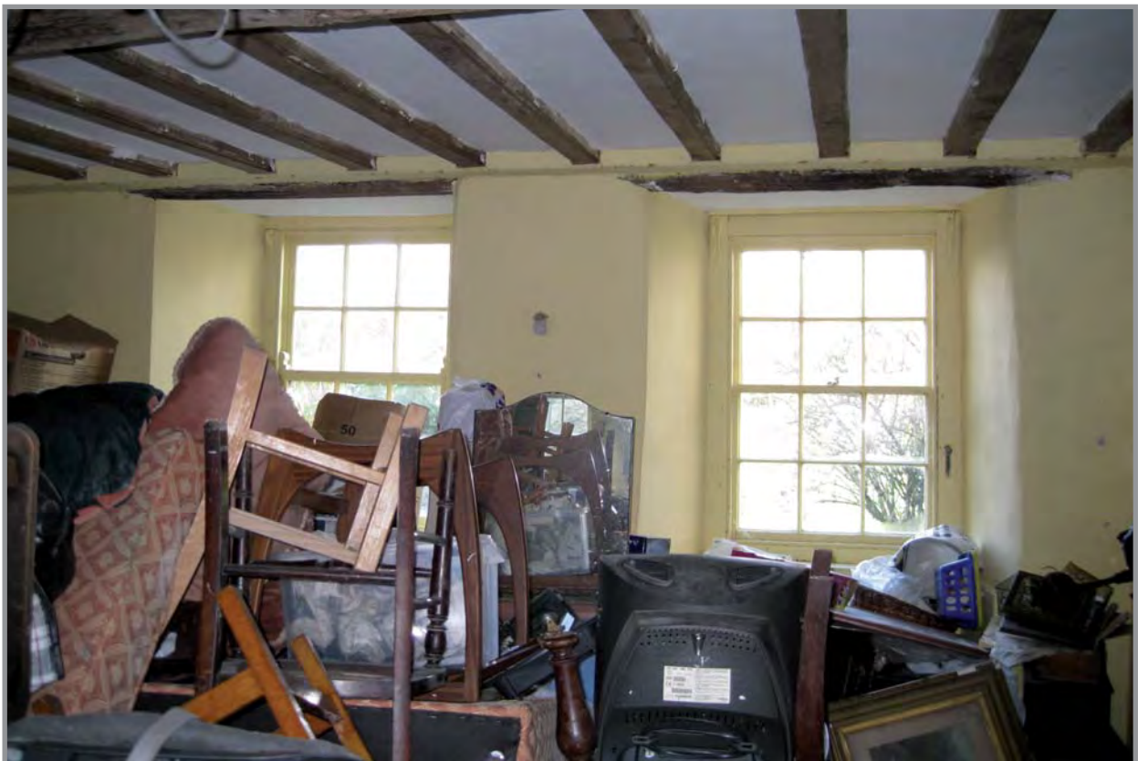
Plate 22: Gronant building A, ground floor 12-pane sash windows facing east
