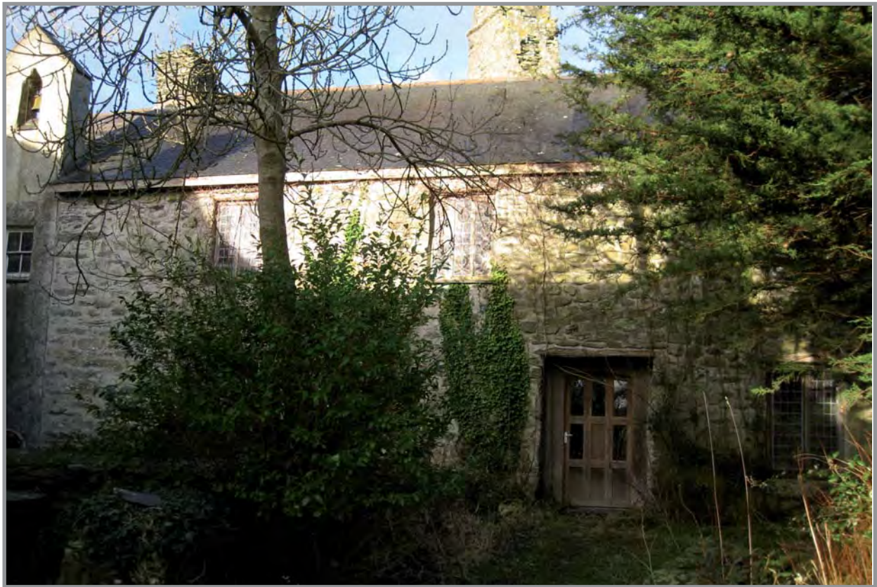
Plate 11: Gronant east facing elevation of building A
