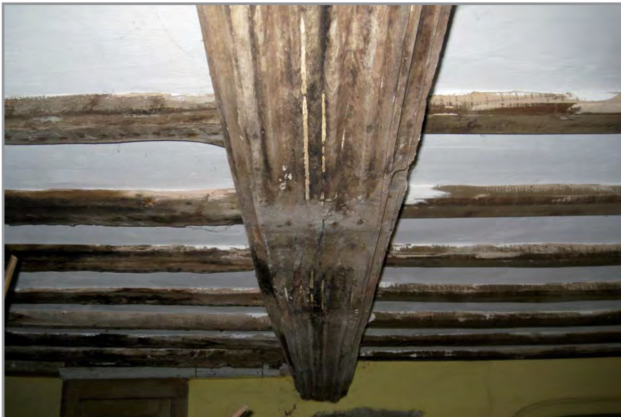
Plate 23: Gronant building A. Heavily moulded beam
