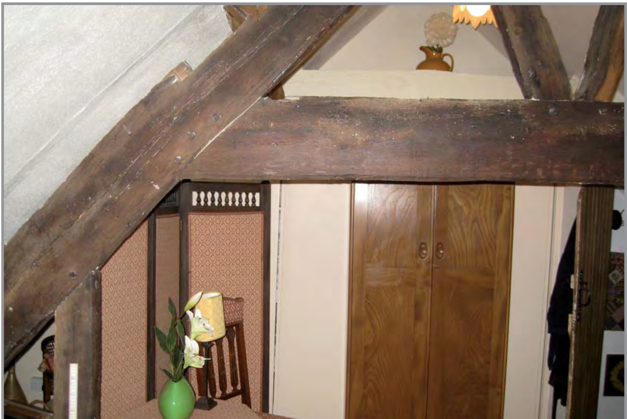
Plate 20: Truss 1 detail in second floor front room. Facing east
