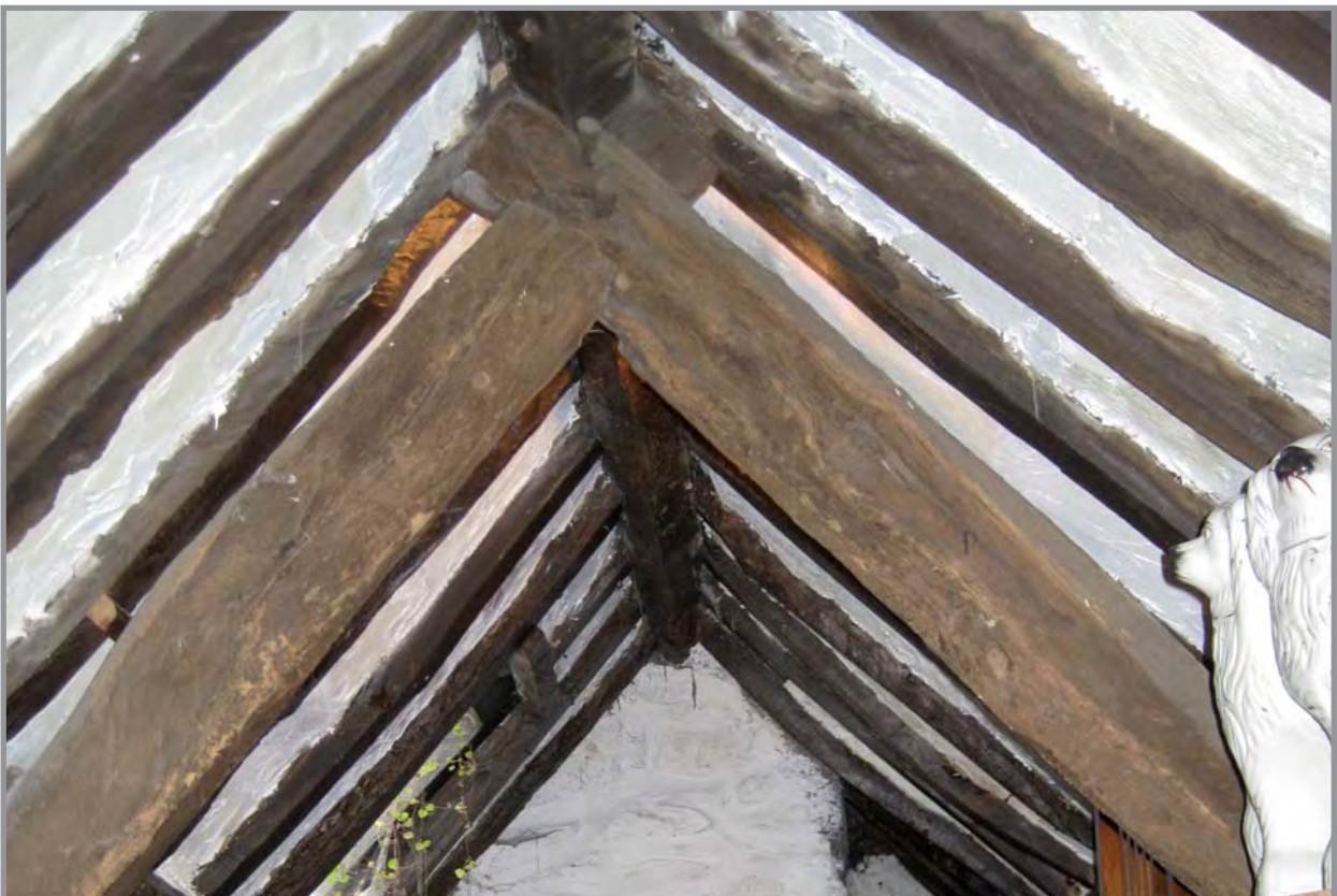
Plate 22: Truss 2 in attic room. Facing south-west
