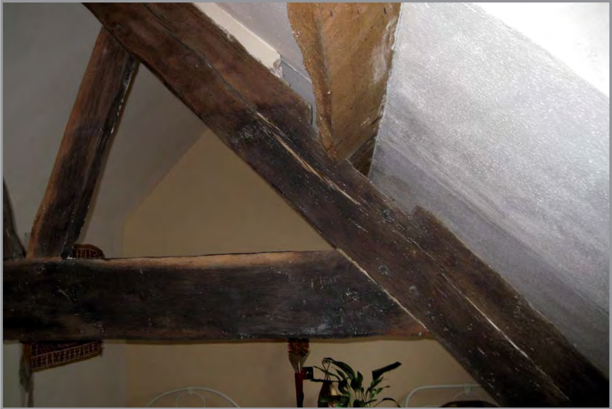
Plate 21: Truss 1 detail in second floor front room. Facing west
