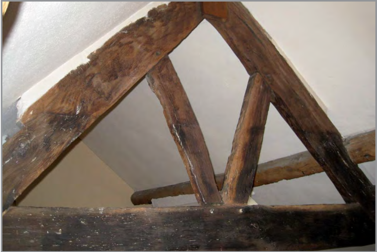
Plate 19: Truss 1 in second floor front room. Facing east
