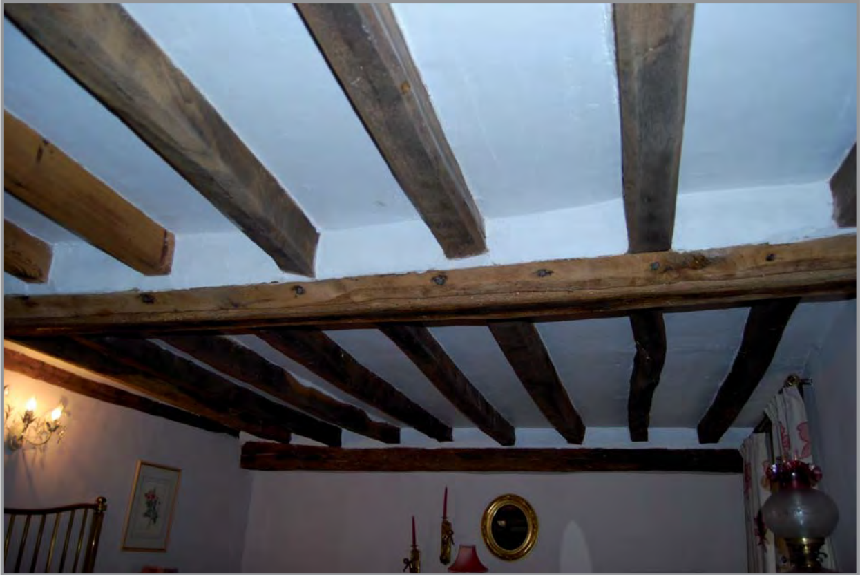
Plate 15: Front bedroom, showing ceiling timbers. Facing North-east
