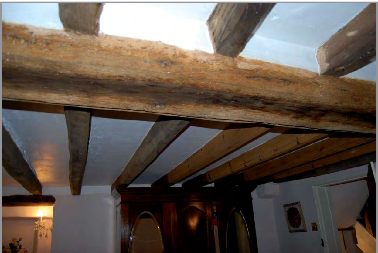
Plate 16: Front bedroom, showing chamfered beam. Facing south
