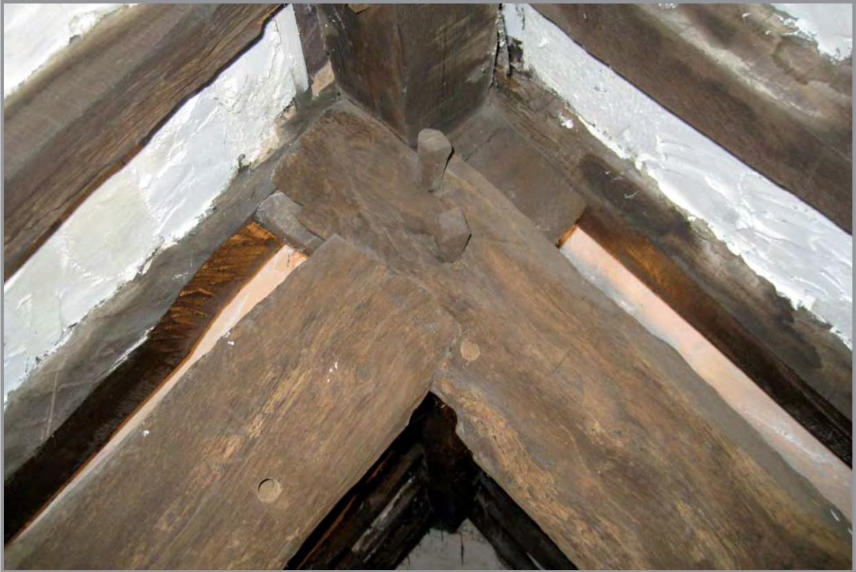
Plate 23: Truss 2 detail of the collar beam truss ridge beam, Facing north-west
