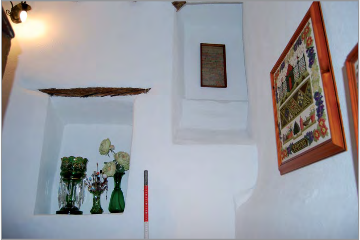
Plate 9: Stairway, showing blocked window. Facing south-west
