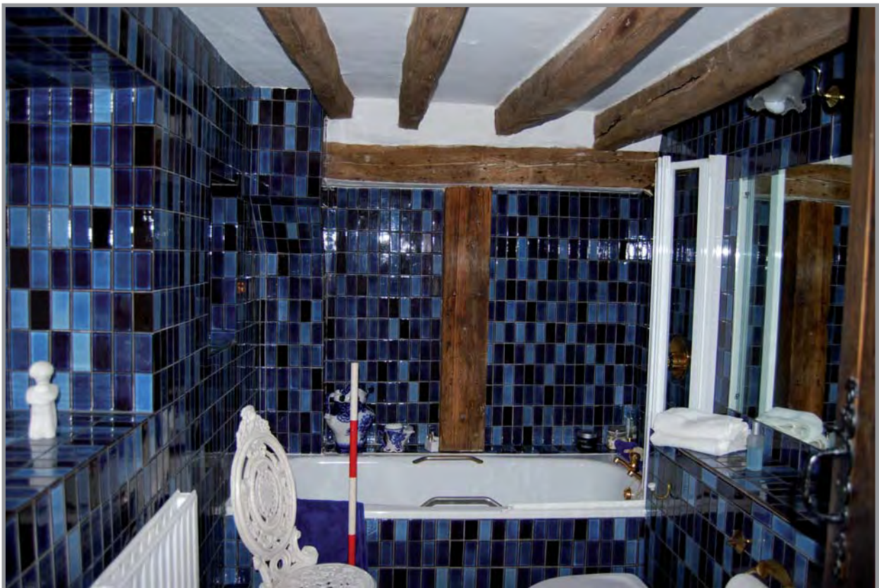
Plate 12: Bathroom, showing timbers. Facing north-west
