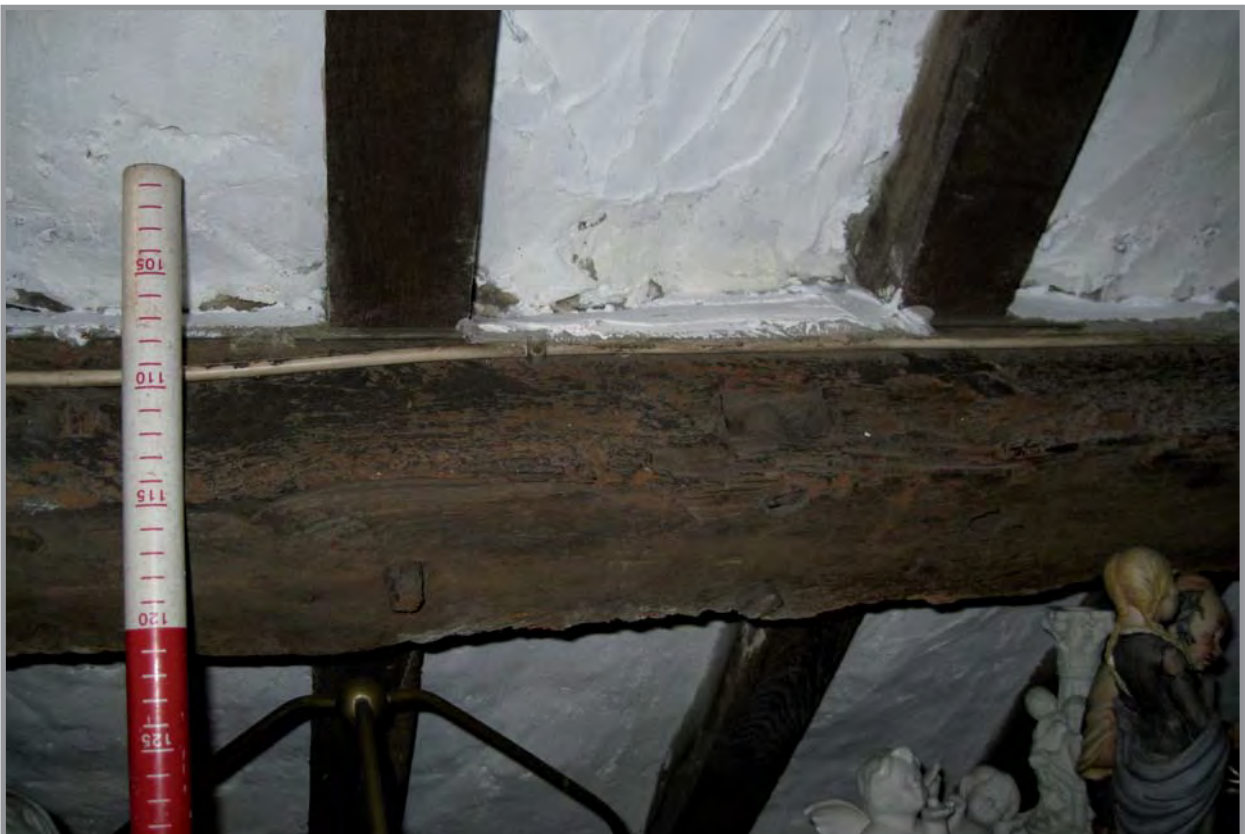
Plate 24: Attic room, showing timber detail. Facing north-west
