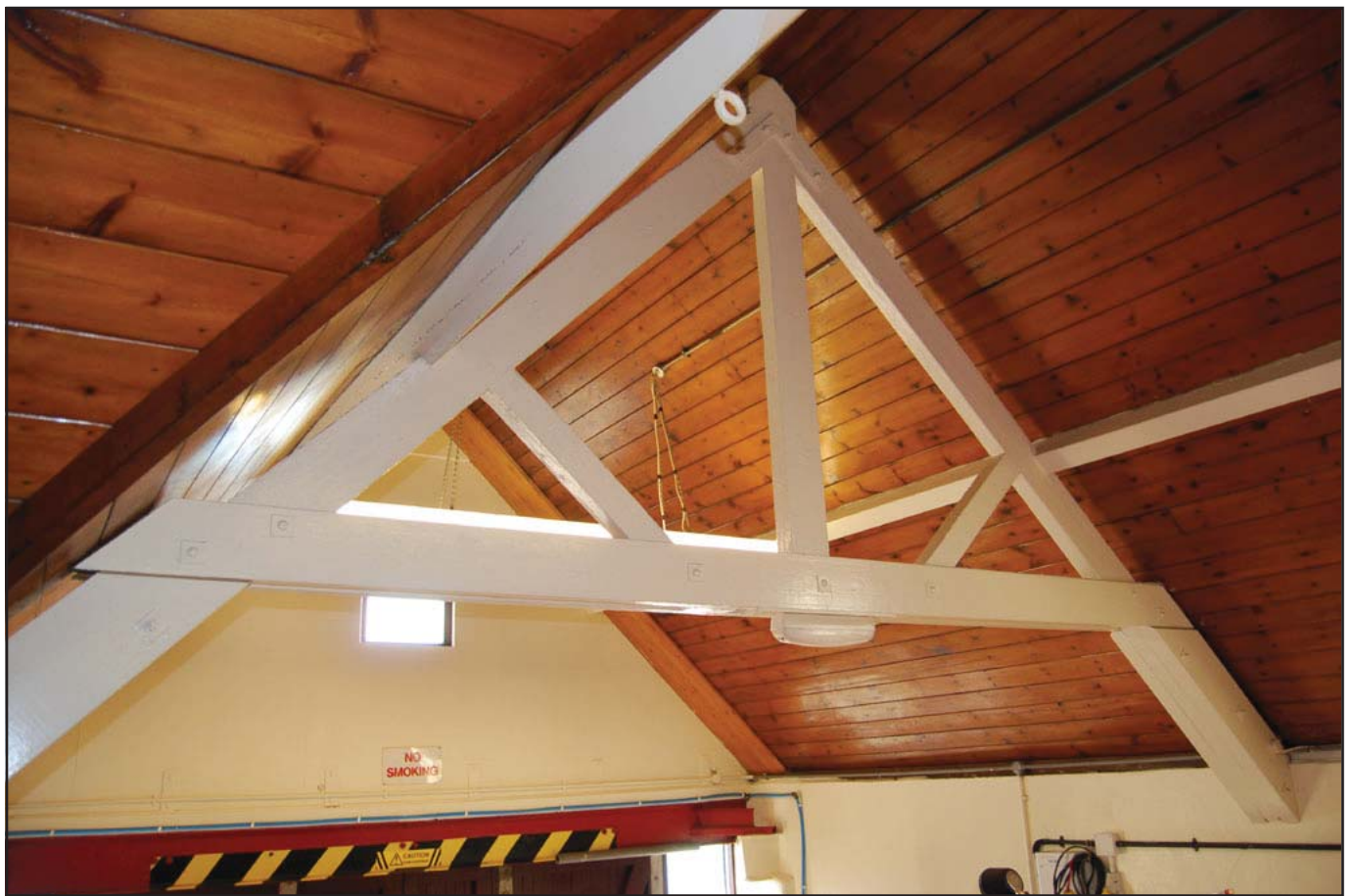
Plate 19 – Detail of A frame truss; view from northeast
