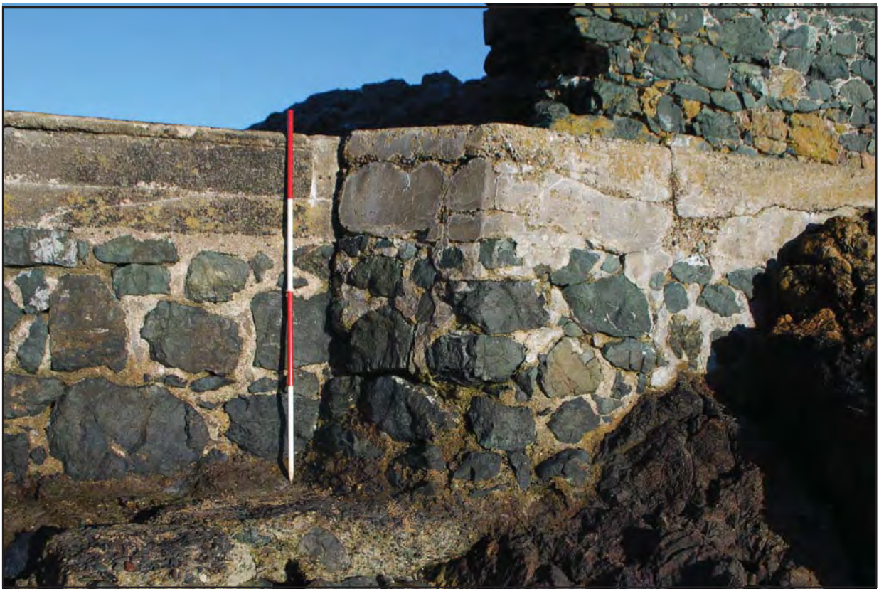
Plate 09 – Detail showing breakwater built around remnants of stub wall (Scale: 2.0m with 0.50m divisions)
