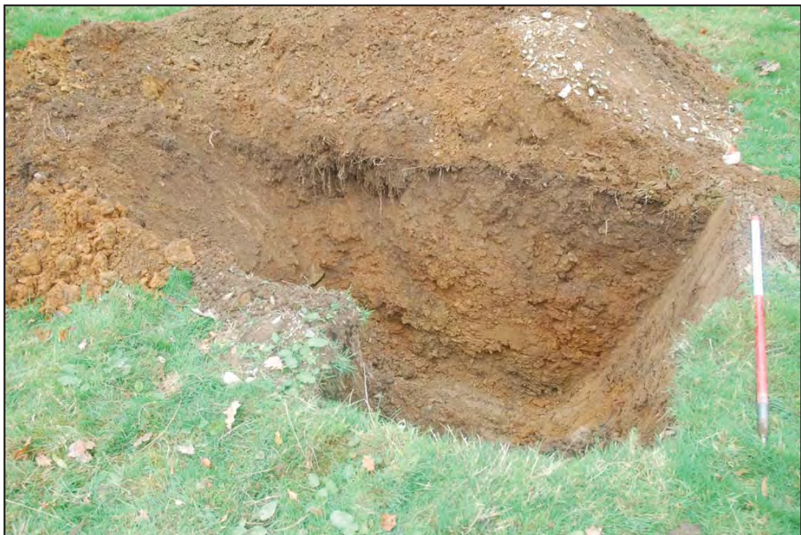
Plate 07: east-facing section of soakaway detailing limit of excavation and exposed sections/stratigraphy. The topsoil was extant to a depth of 0.26m followed by an orange clay-silt; followed by a mid-brown gravel-clay to limit of excavation (ranging pole: 1.0m)
