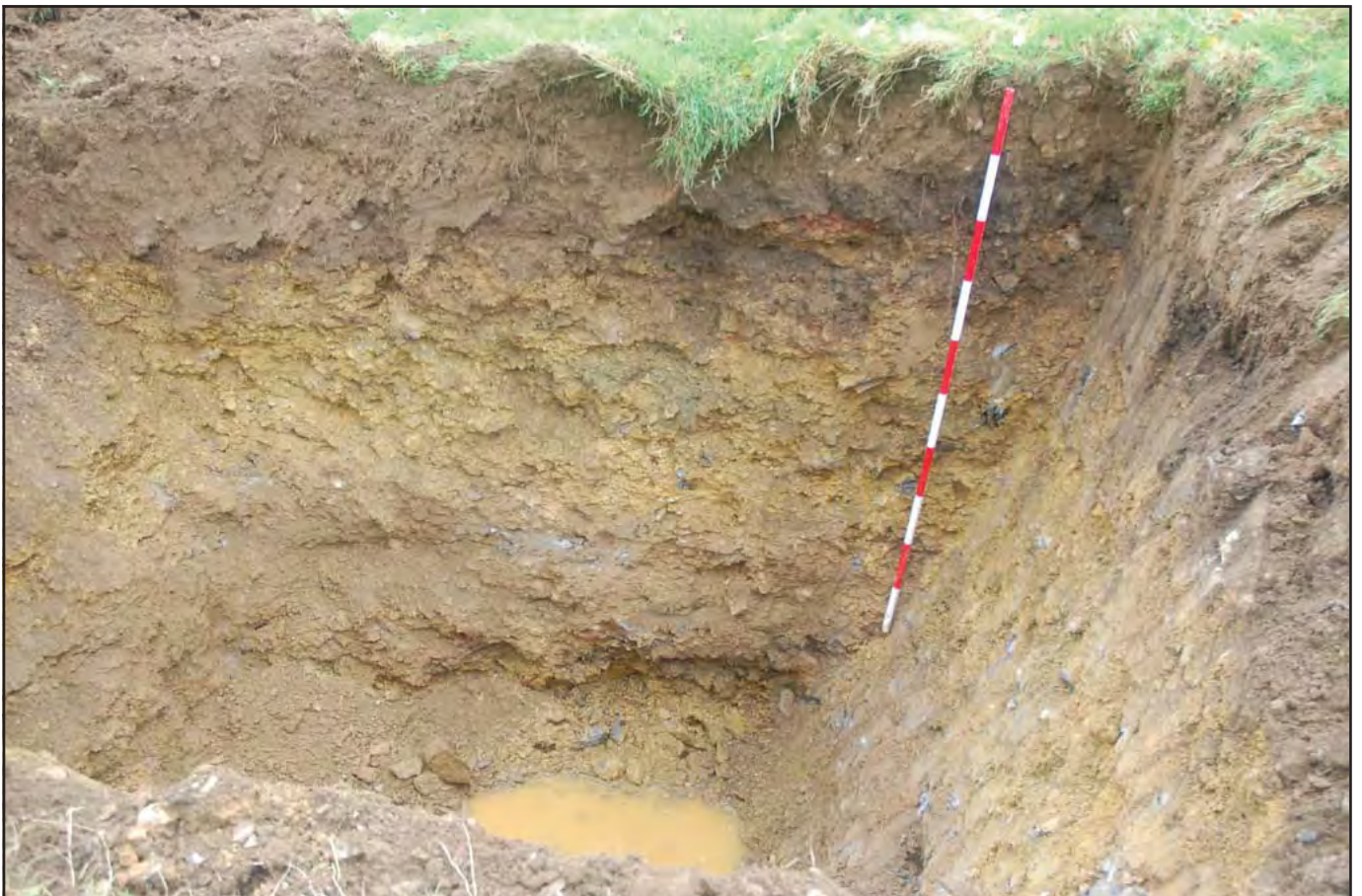
Plate 05: view west of the septic tank excavation detailing limit of excavation. The pit was excavated into a slope and comprised topsoil of varying thickness followed by two distinct glacial deposits (ranging pole: 2.0m)
