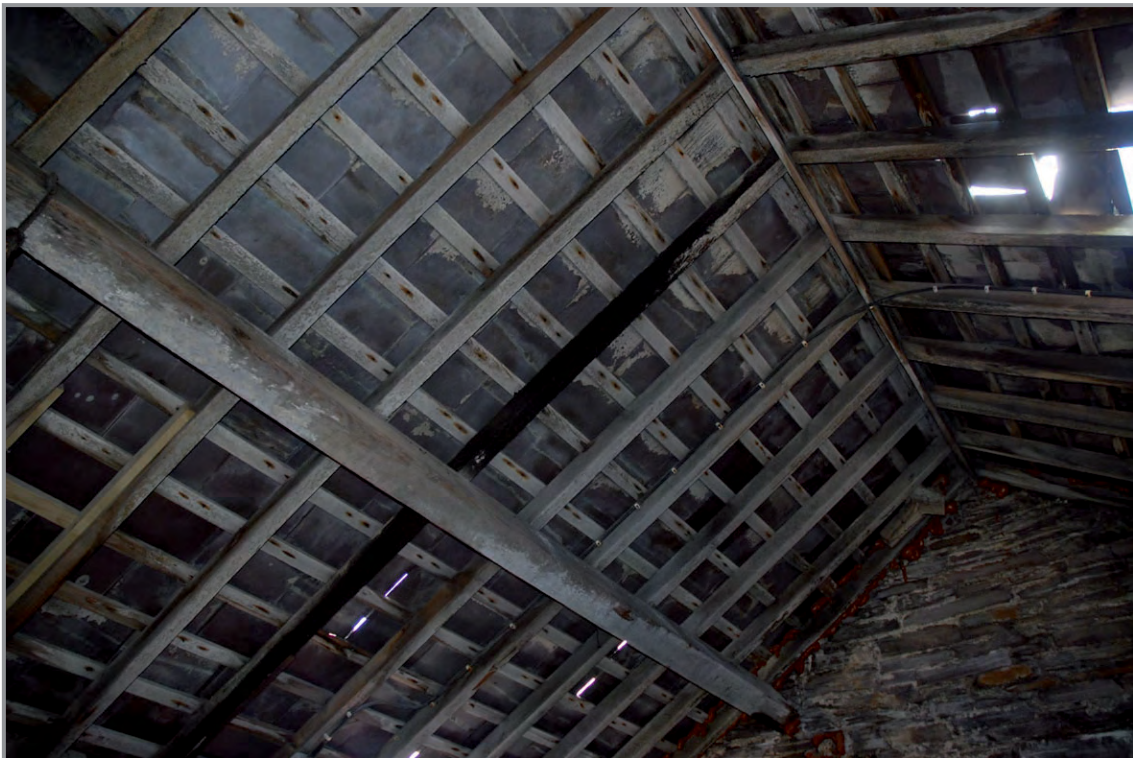
Plate 17: Building 54. Internal view taken from the south. Showing the replacement roof.
