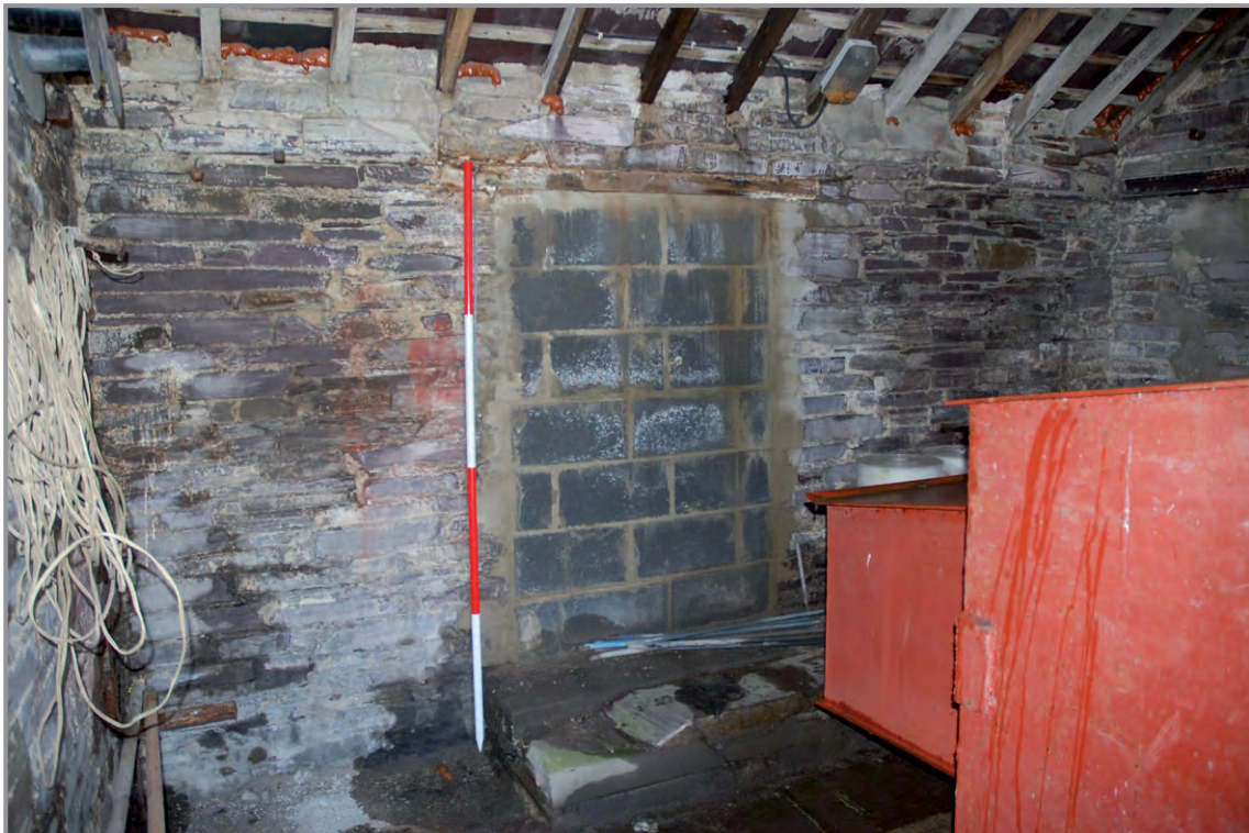
Plate 11: Building 54. South-east elevation internal. Showing the blocked doorway in the north-west facing elevation.
