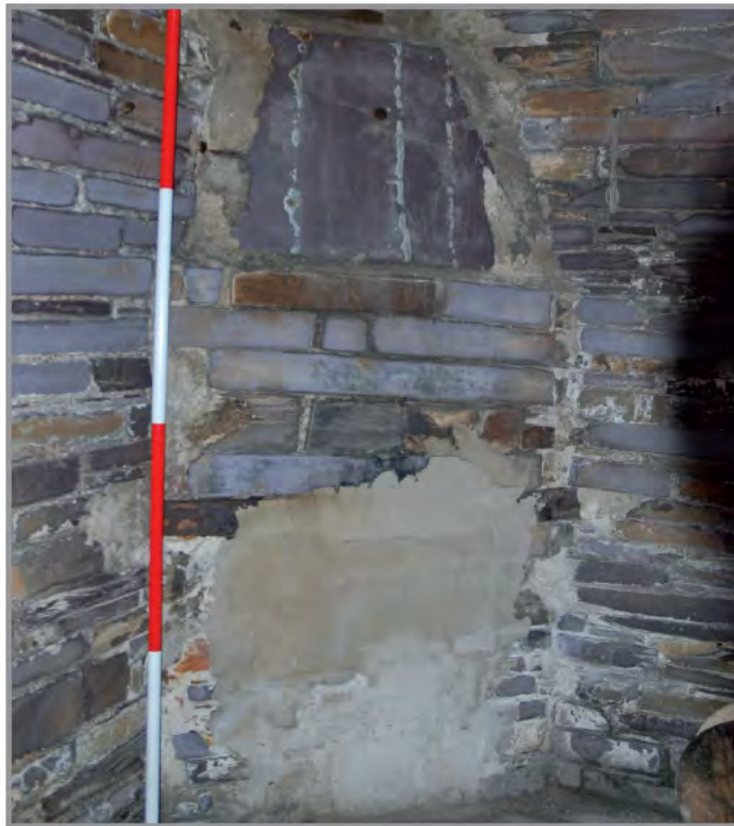
Plate 8: Building 54. Internal view taken from the east. Showing the blocked fireplace.
