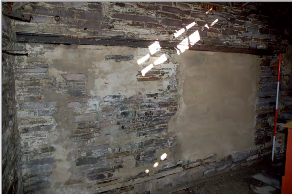
Plate 9: Building 54. South-west elevation internal. Showing the two phases of blocking of the original winding house opening.
