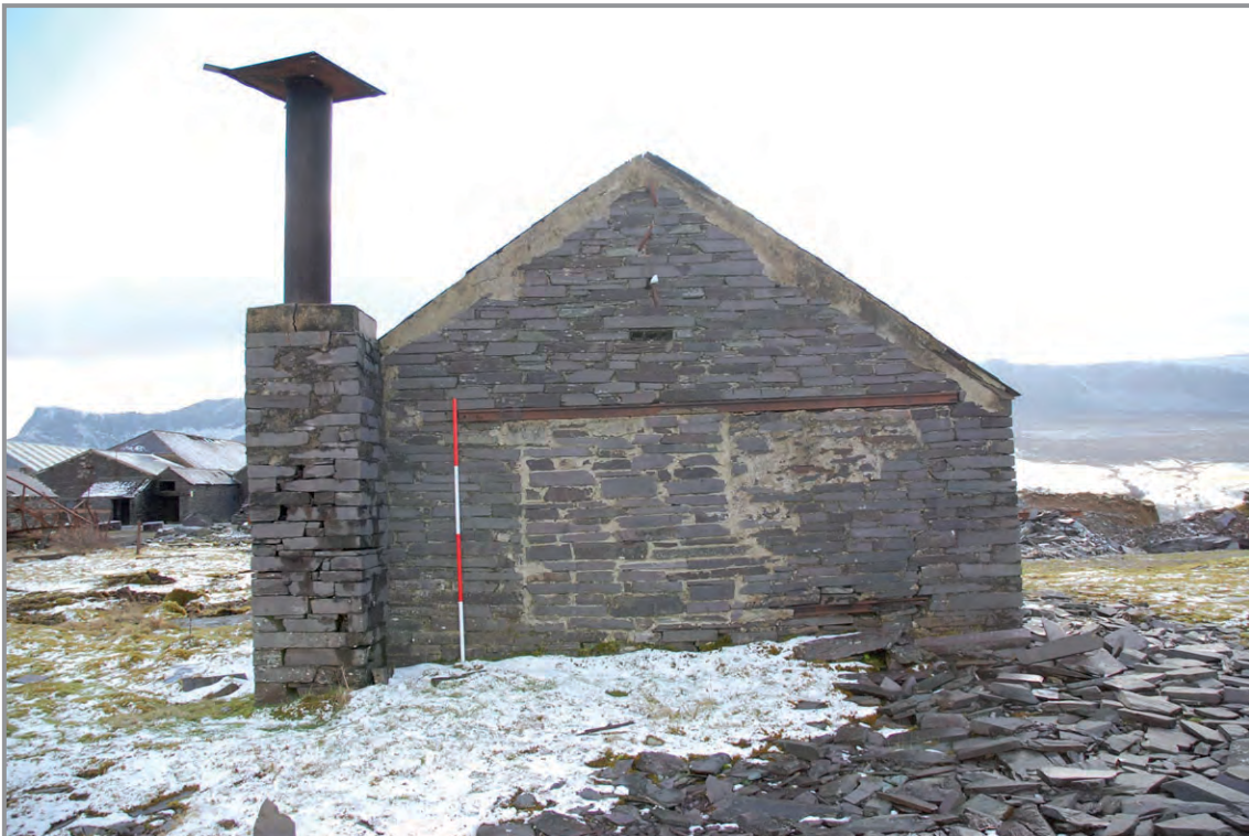
Plate 7: Building 54. View of the south-west elevation. Showing the two phases of the blocked opening and chimney, which was added at a later date. With the Eureka mill in the background
