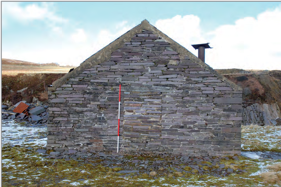
Plate 5: Building 54. View of the north-east facing elevation. Showing the blocked window.
