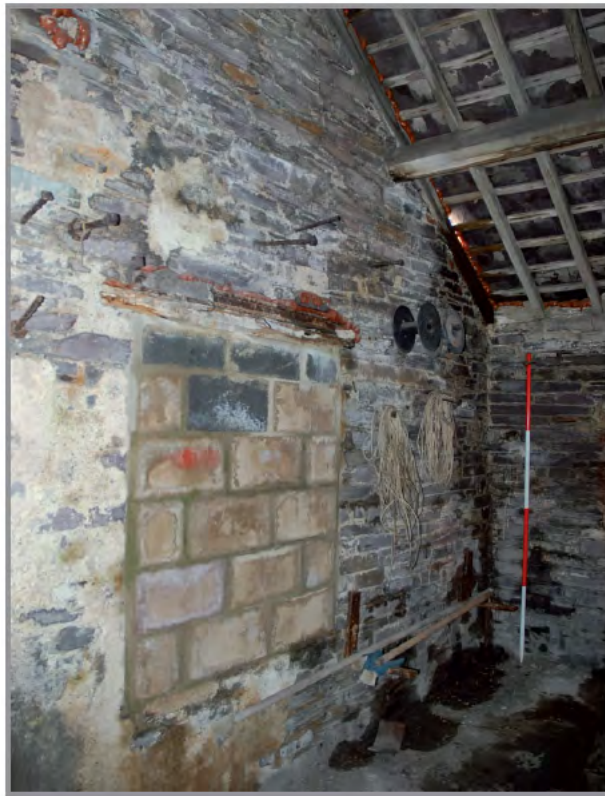
Plate 12: Building 54. North-east elevation internal. Showing the blocked window.
