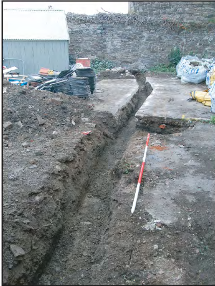
Plate 01: Zone 1/YARD 1 (PRN 30451): view southeast of service trench excavation (14.0m in length, 0.70m in width and 0.50m depth). Note enclosure wall A in the background, which defined the original quay layout and was retained as part of the redevelopment programme and concrete pad at former location of Building 18 (PRN 30453). (Ranging pole: 2.0m)
