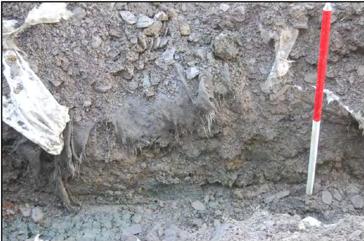
Plate 08: Zone 2/Yard 4 (PRN 30463): service trench excavation - detail of full excavation depth and contaminated soil associated with former garage
