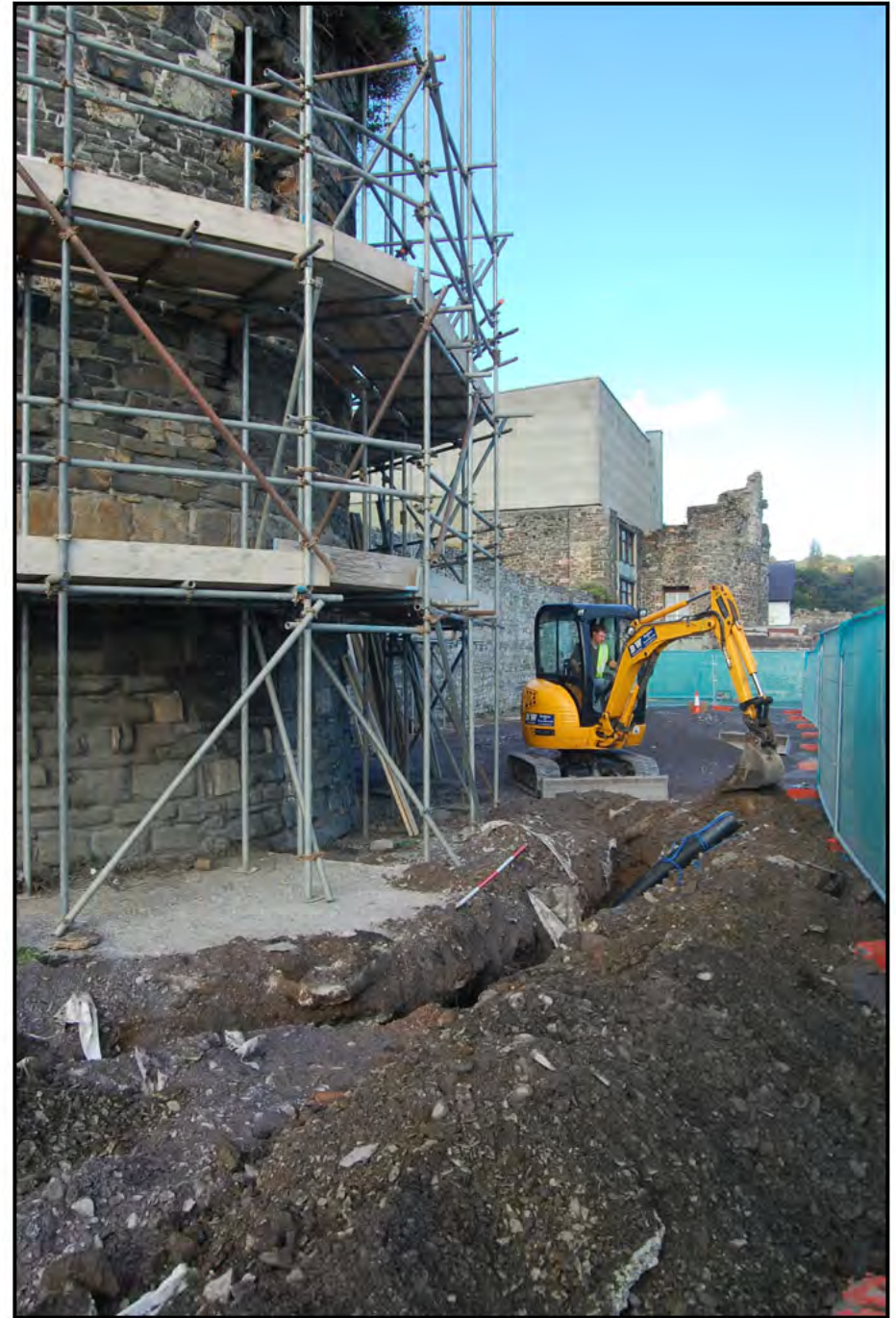
Plate 06: Zone 2/Yard 3 (PRN 30457): service trench excavation - detail of excavation surrounding Tower 3 with concrete pad associated with Building 12 (PRN 30461) towards left of image (Ranging pole: 2.0m)
