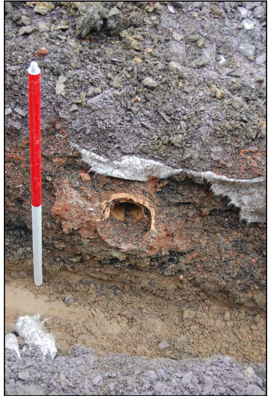
Plate 04: Zone 2: service trench excavation - detail of disused water pipe held in a red brick and concrete mixed covering (Ranging pole: 1.0m).
