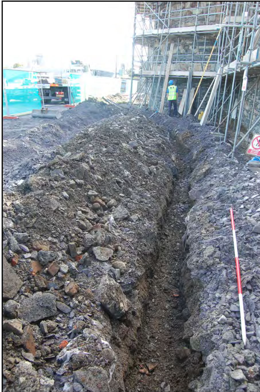
Plate 09: Zone 2/Yard 4 (PRN 30463) to Yard 5 (PRN 30468): service trench excavation - completed length with Tower 3 in the background. (Ranging pole: 2.0m)
