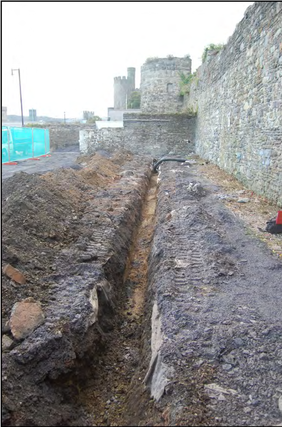
Plate 05: Zone 2: service trench excavation - detail of full excavation depth
