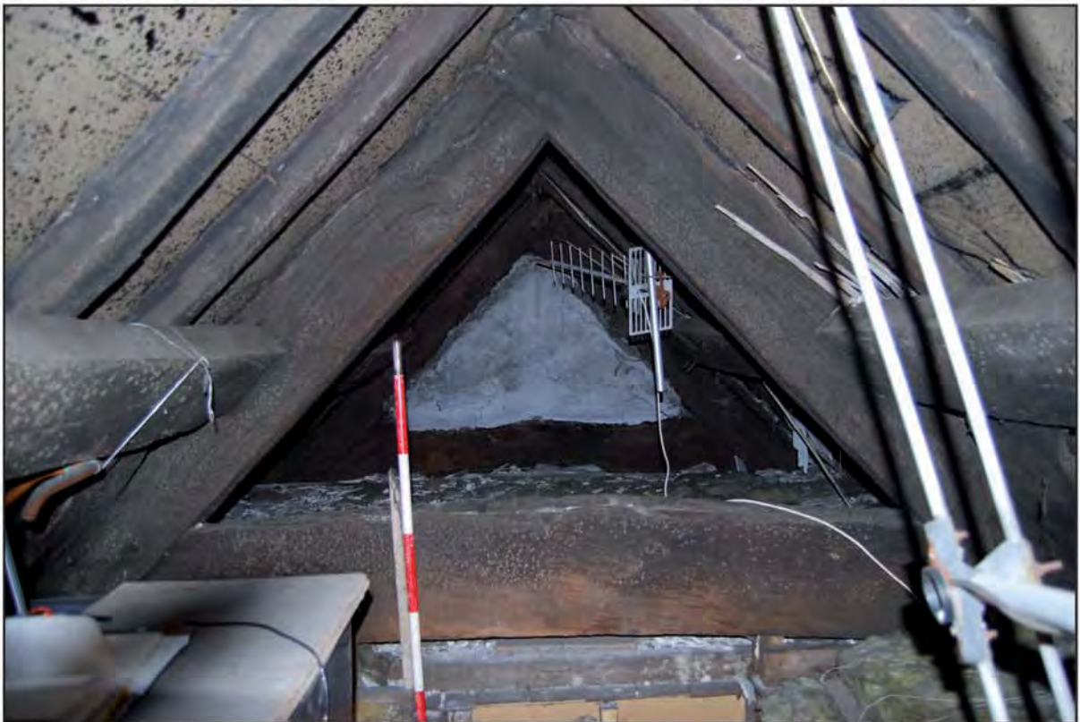
Plate 4: North facing image of truss 2 & 3.
