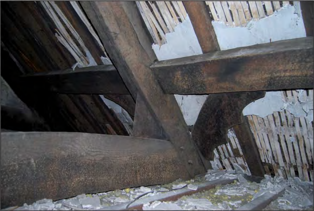
Plate 5: North-west facing image of the wind brace attached to truss 4.
