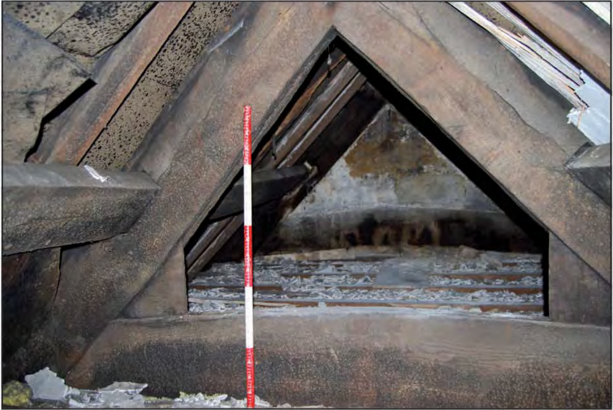
Plate 3: South facing image of truss 4.
