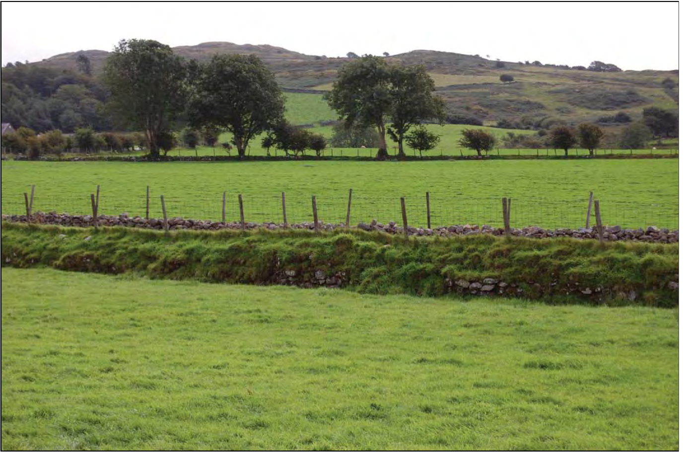
Plate 7: Field boundary wall feature 15 from the north
