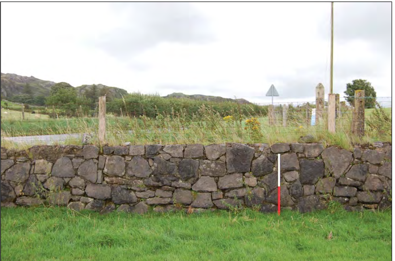
Plate 6: Field boundary wall feature 10 from the west
