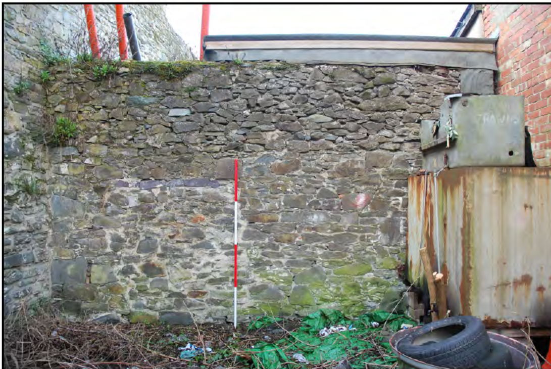
Plate 1: YARD 1 (PRN 30452): Cross Wall A: south-facing elevation of rubble-built mortared stone wall 3.0m high that defined the northern boundary of Yard 1; the topmost metre is a later addition. A blocked entrance is visible to the left of the ranging pole. (Ranging pole: 2.0m)
