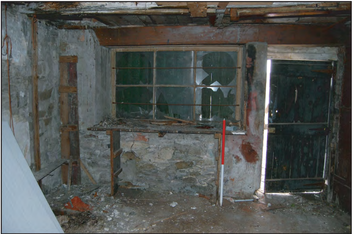
Plate 10: Yard 01 (PRN 30451)/Building 01 (PRN 30452): internal view of east wall: ledged door and window. (Ranging pole: 1.0m)
