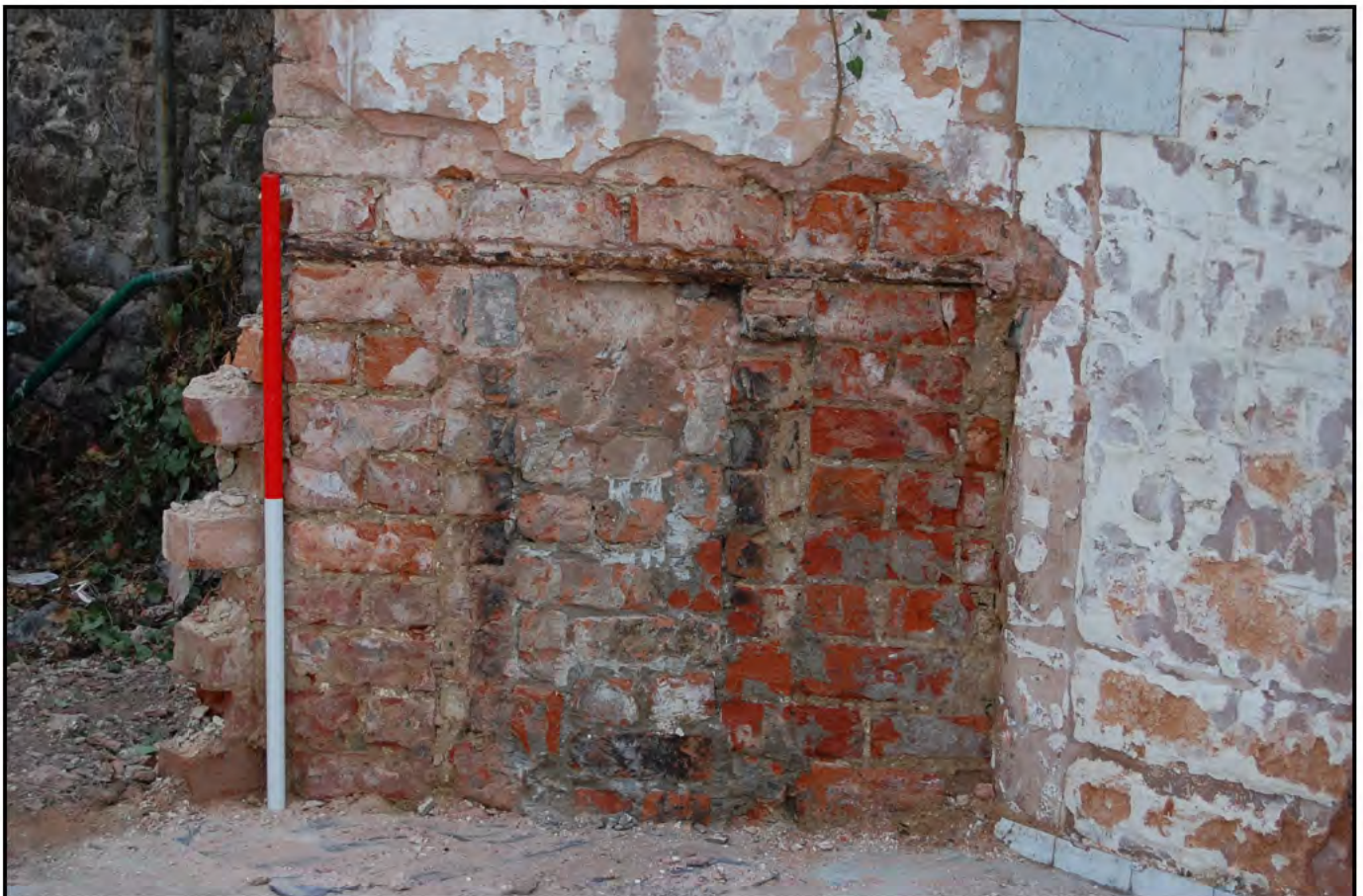
Plate 27: YARD 3 (PRN 30457): Building 13 (PRN 30462): internal fireplace associated with chimney (plate 26), identified during demolition phase (Ranging pole: 2.0m).
