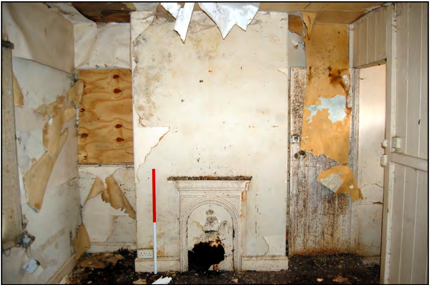
Plate 46: YARD 5 (PRN 30468): Building 05 (PRN 30469) (internal): The first floor comprised a single room , with three single-hung sash windows. A small cast iron Victorian arched fireplace remained in situ.
