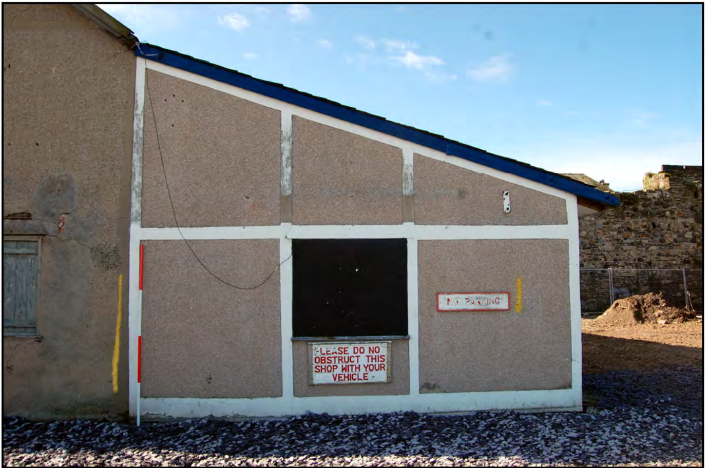
Plate 16: YARD 02 (PRN 30454): Building 02 (PRN 30455): east elevation (quay side) prior to demolition. The east elevation measured 5.30m in width and 3.95m in height, with pebbledash render. A blocked window was extant towards the centre of the elevation, c.1.00m above ground level (window measurements: 1.00m in height and width). (Ranging pole: 2.0m)
