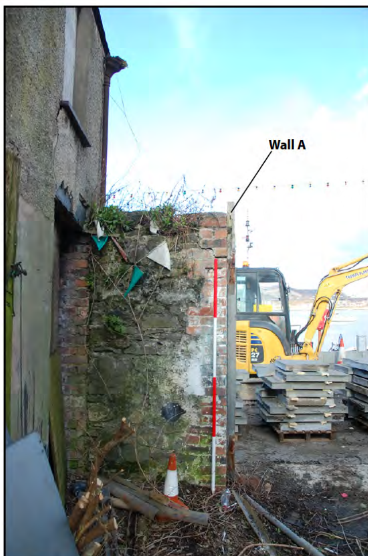
Plate 2: YARD 1 (PRN 30452): Wall A: view east of enclosure wall (Wall A) that initially surrounded the entire quay but was subsequently altered to accommodate new entrances/structures. Entrance through Wall A into Yard 1 visible in this example (Ranging pole: 2.0m)
