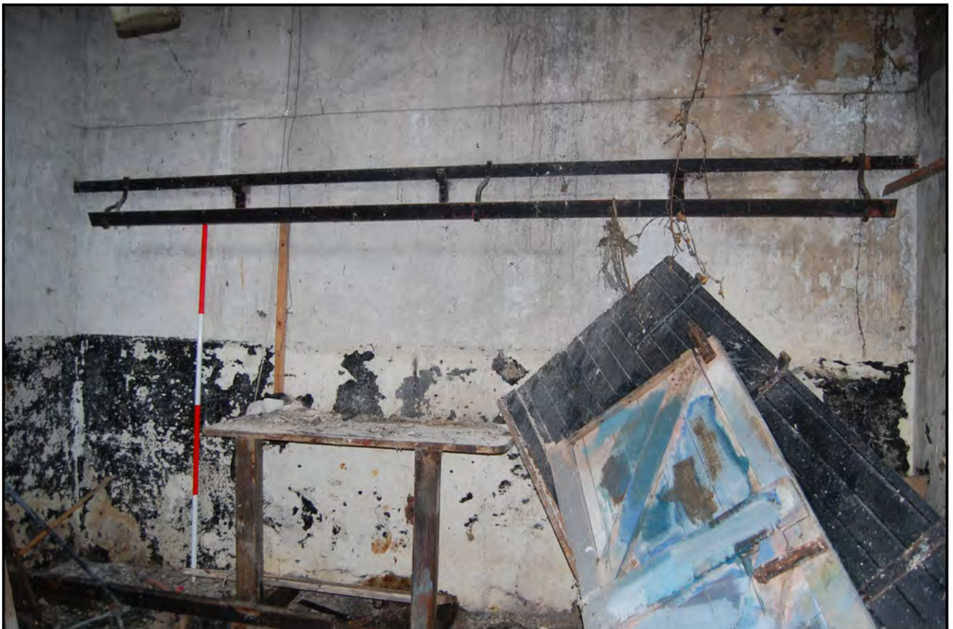
Plate 59: YARD 6 (PRN 30474): Building 08 (PRN 30476): internal view of former slaughterhouse, a range of metal rails with sliding hooks that were extant on all elevations except the front entrance. (Ranging pole: 2.0m)
