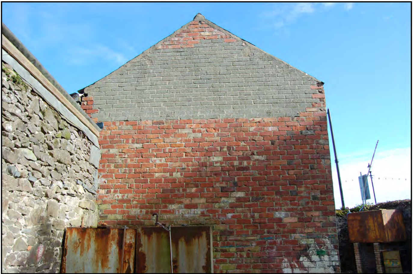
Plate 06: YARD 1 (30451): Building 01 (30452): west elevation, built largely of red brick using a stretcher bond with first floor grey brick repair. Note Cross Wall A at left of image.
