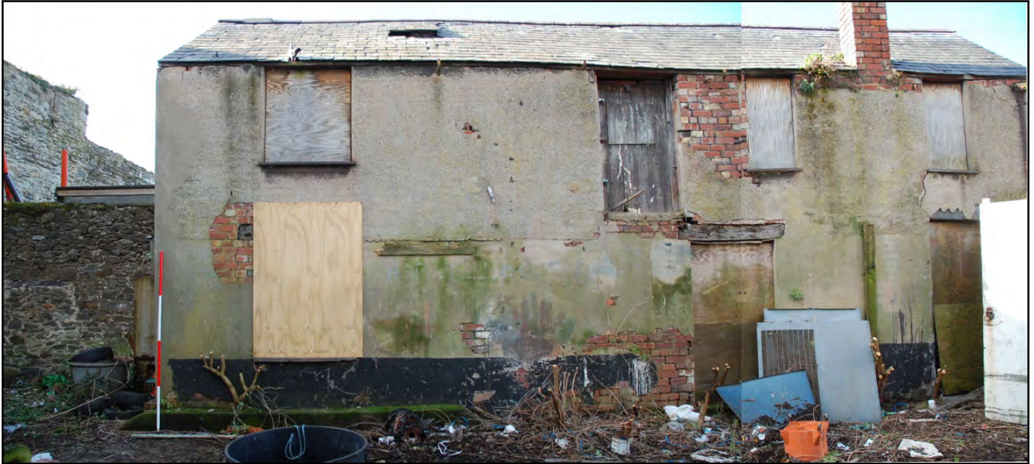
Plate 05: YARD 1 (PRN 30451): Building 01 (PRN 30452): south elevation: measured 10.84m in length and 3.95m in height. This elevation was in red brick (stretcher bond) partly covered by roughcast render. On the ground floor were two doors and one window, whilst on the first floor were three windows and a door. A single stack brick-built chimney rises from this wall, between the two windows, surmounted by a bishop-style chimney pot. Cross Wall A is visible to left of Building 01 (cf. plate 01) (Ranging pole: 2.0m)
