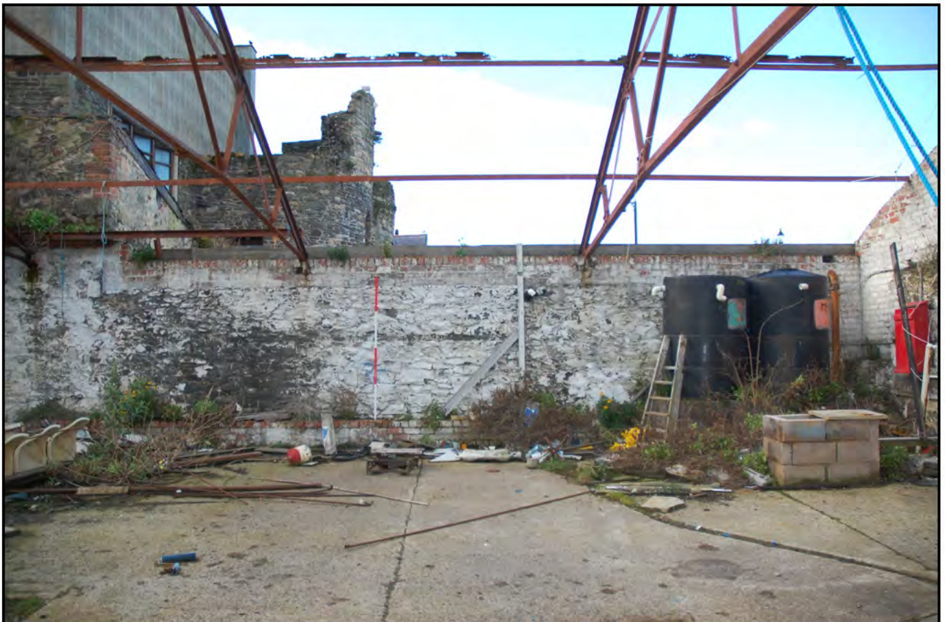
Plate 51: YARD 5 (PRN 30468): Cross Wall D: view north of elevation, which formed the northern boundary of YARD 5. The wall reached a total height of 2.6m including a 0.4m brick rebuild on the top that held the roof supports. Steel girders had also been inserted into the town wall as part of the roof structure. There was also a 0.40 m high dwarf brick wall built against the bottom of Cross Wall D but the function was unknown. Cross Wall D had been partly repaired in brick at the east end plate 51.
