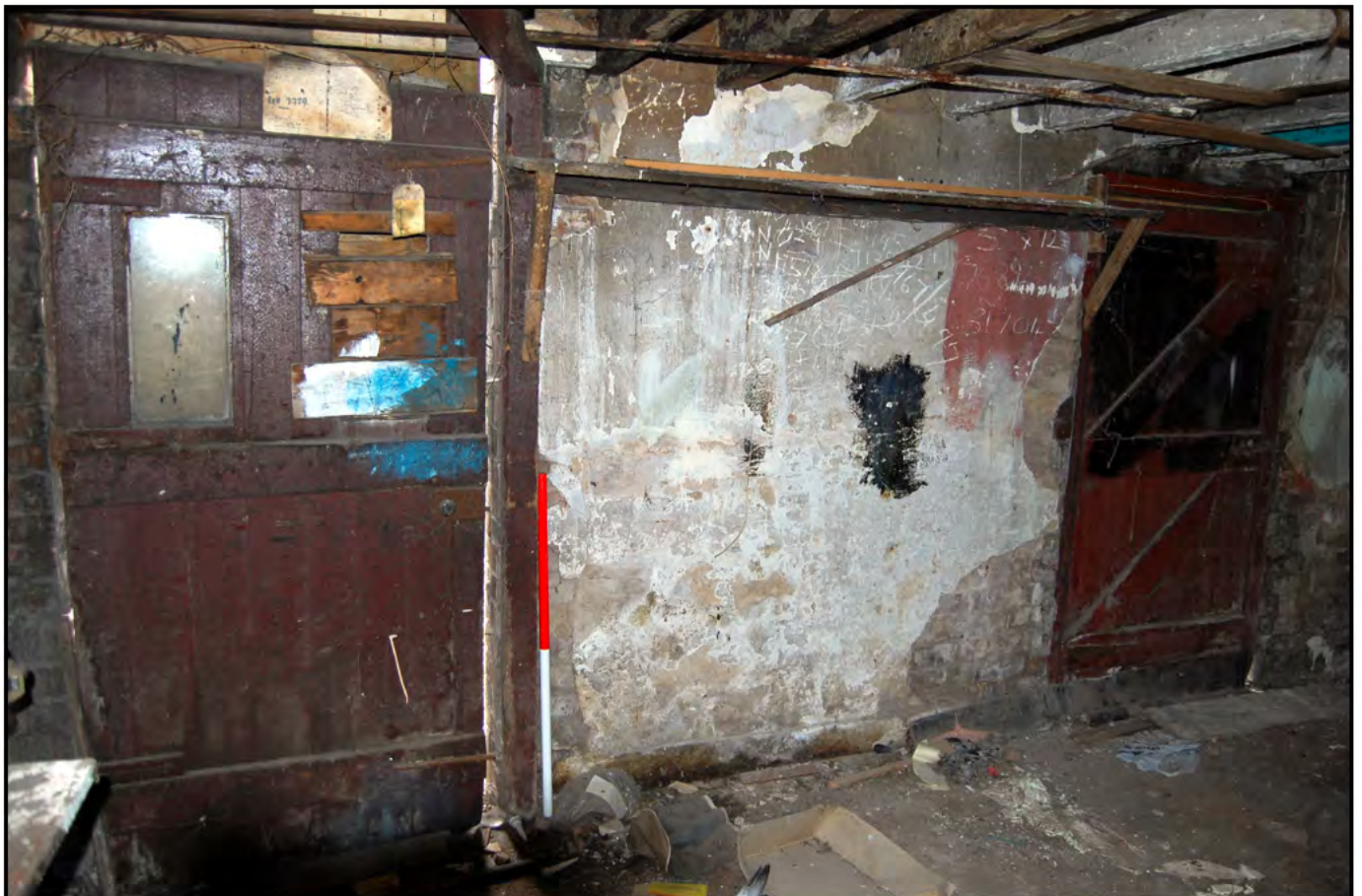
Plate 09: Yard 01 (PRN 30451)/Building 01 (PRN 30452): internal view detailing ground floor (south wall). one ledged and braced door and one ledged door surviving in the south wall. (Ranging pole: 1.0m)
