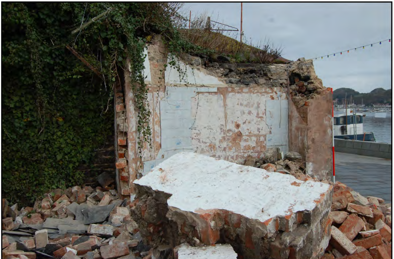
Plate 25: YARD 3 (PRN 30457): Building 13 (PRN 30430462): removal of south-facing elevation during demolition phase, detailing rendered and tiled internal elevations. (Ranging pole: 2.0m)
