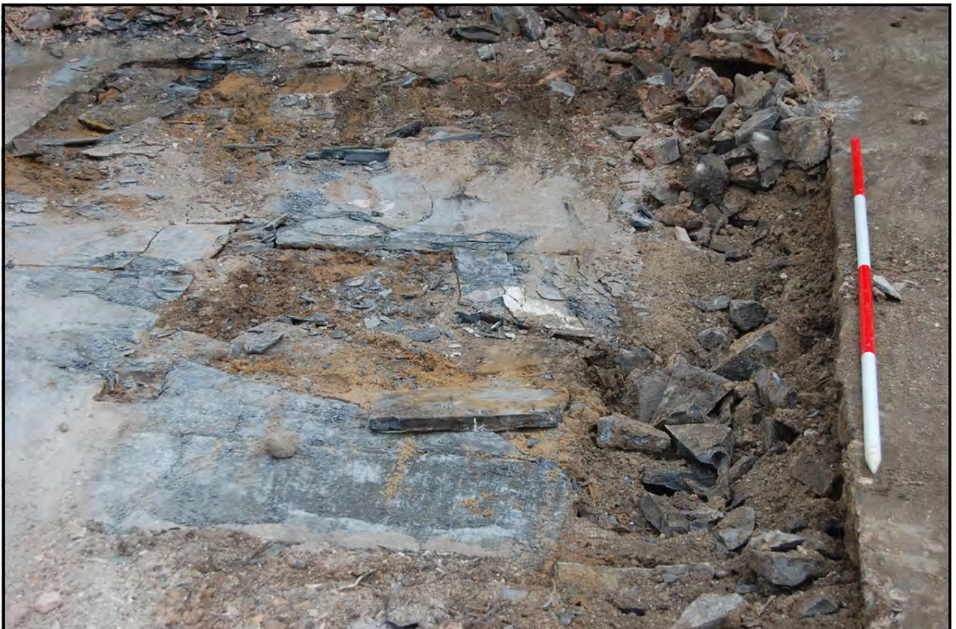
Plate 37: YARD 4 (PRN 30463): Building 14 (PRN 30465): during demolition: the floor was made of large (up to 1.0m 2 ) slate slabs plate 36 laid on yellow sand. The floor level within Building 14 was some 0.25m lower than the modern concrete floors of Building 04 (PRN 30464) and probably represented the original floor/yard levels.
