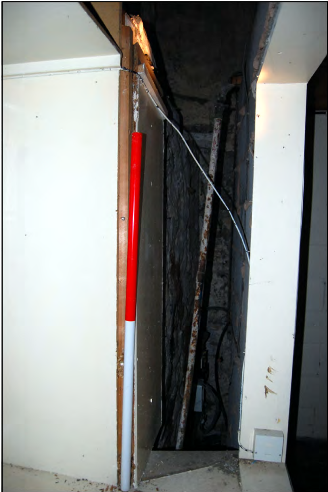
Plate 18: YARD 2 (PRN 30454): Building 02 (PRN 30455) (Internal): The east elevation window was identified internally as a recessed bay window. An inspection of this feature revealed that a thermal block wall had been built as a false wall parallel to the original elevation. The latter was partially visible where drywall from the bay window had been removed, exposing whitewashed stone walling . (Ranging pole: 1.0m)
