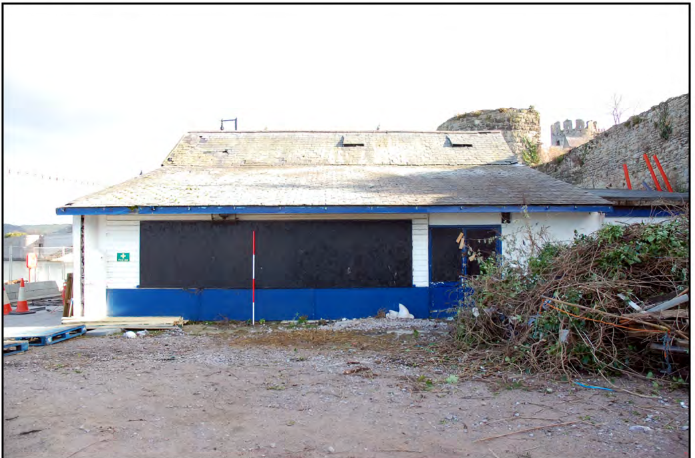
Plate 15: Yard 2 (PRN 30454): Building 02 (PRN 30455): a single storey lean-to located against the south wall of Yard 2, opposite Building 01 (PRN 30452), with which it shared a common wall (Cross Wall A). A modern extension had been constructed onto the western end of the building. (Ranging pole: 1.0m)
