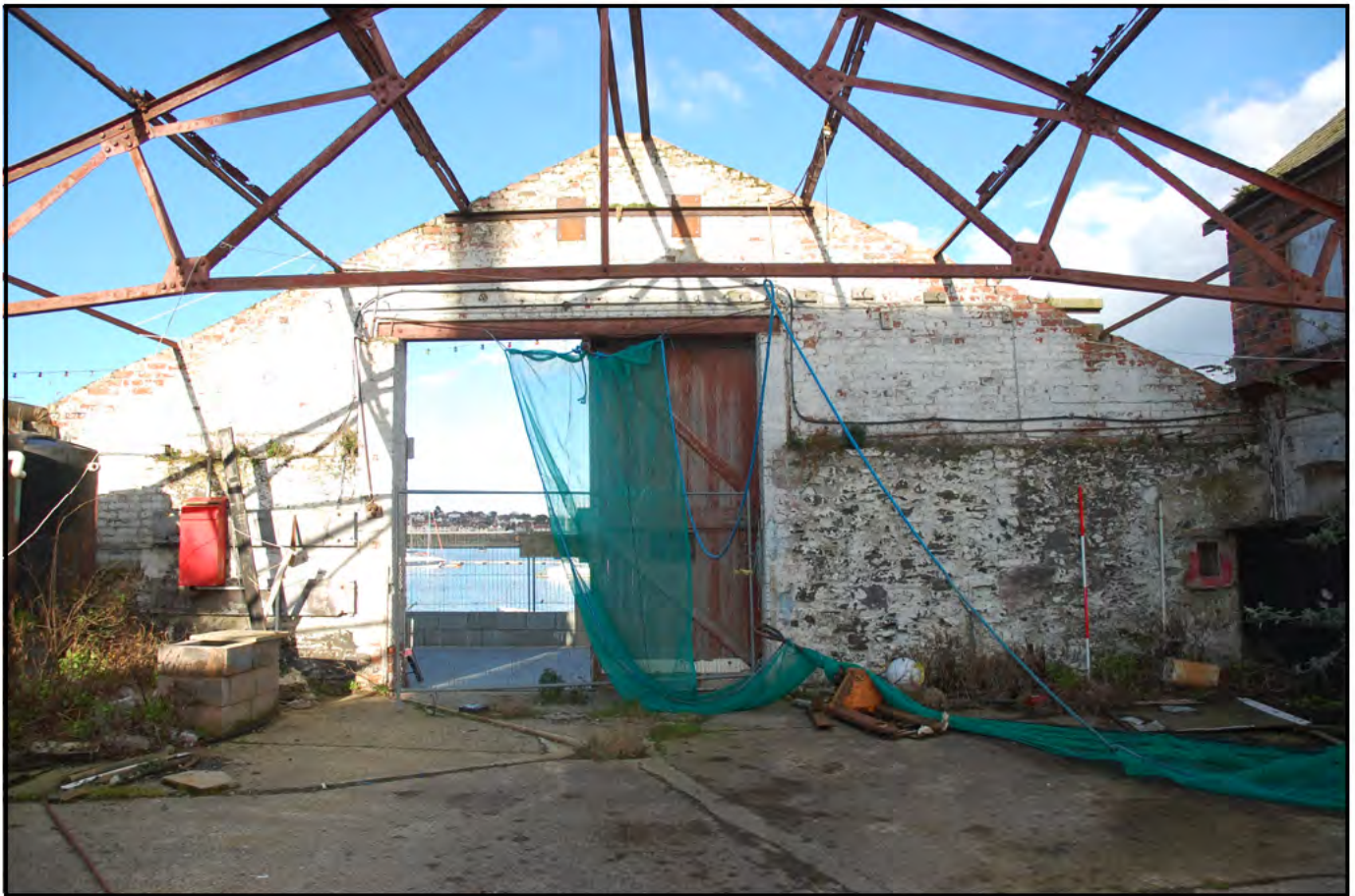
Plate 48: YARD 5 (PRN 30468): Building 06 (PRN 30470): this building was, in effect, Yard 5 with a roof on. The building/yard measured 16.4m x 16.0m (l x w), but excluded the south-east corner occupied by Building 05. Wall A (quay enclosure wall) is visible forming part of the east (quay) wall surmounted by brick. (Ranging pole: 2.0m)
