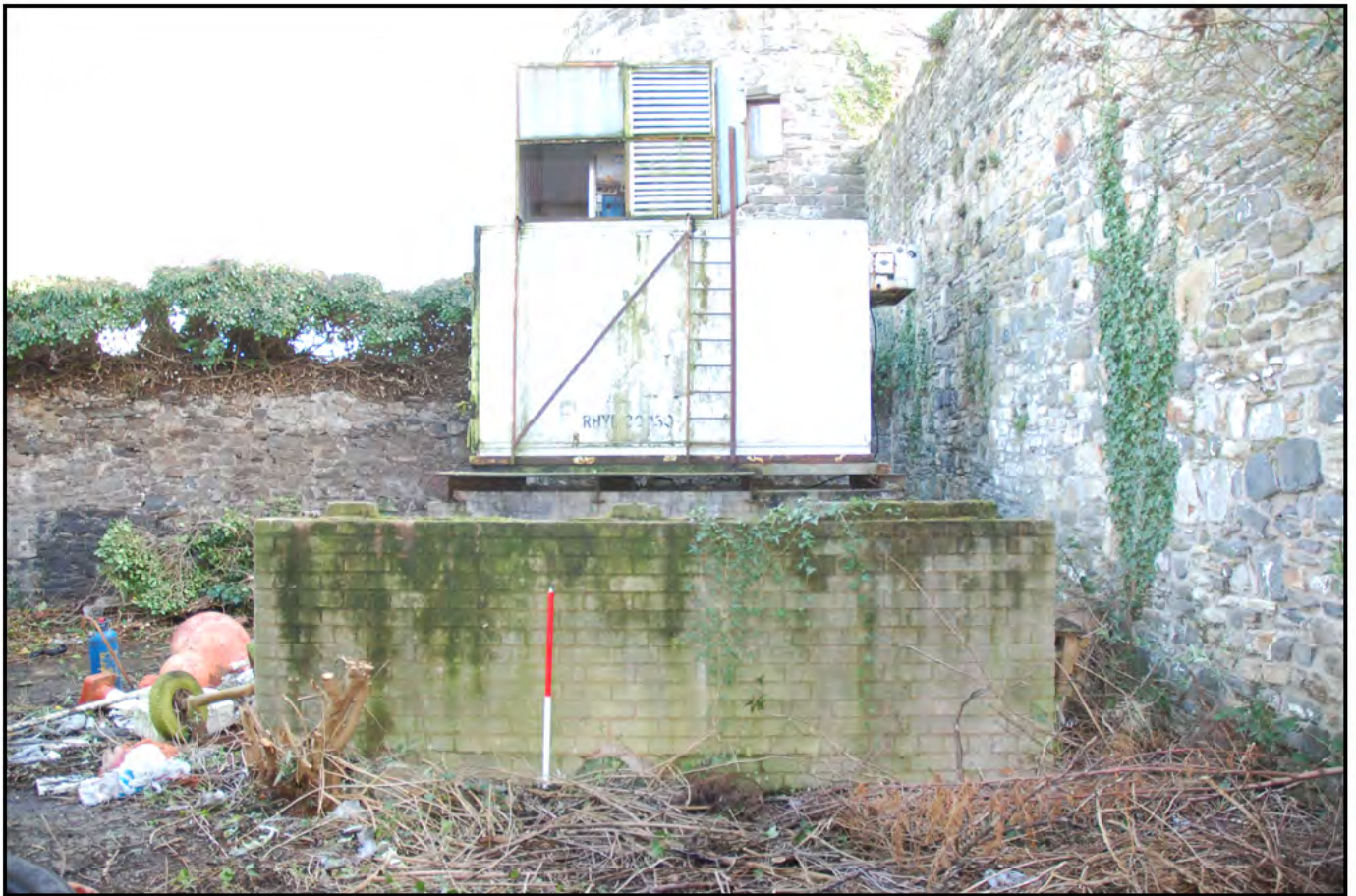
Plate 14: YARD 1 (PRN 30451): Ice plant built in 1993 to replace Building 23 (PRN 19749) (cf. plate 13). Located at the rear of Yard 1. This unit produced ice on demand but did not have the capacity to store surplus ice. (Ranging pole: 1.0m)
