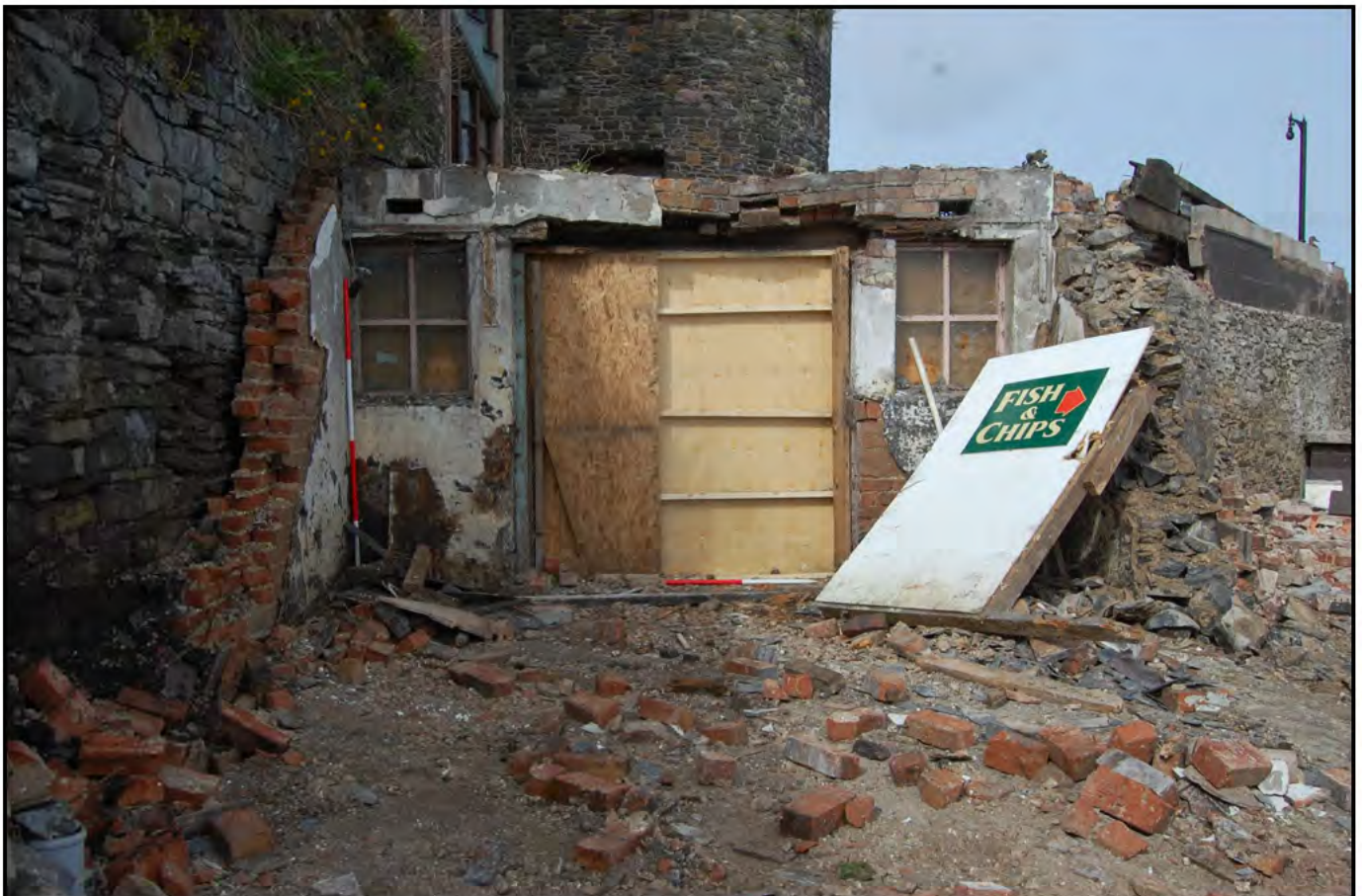
Plate 63: YARD 6 (PRN 30474): Building 08 (PRN 30476): demolition/watching brief phase: Building 08 utilised the existing short length of stone wall forming the rear elevation of Building 07 (PRN 30475), Cross Wall D and Wall A, forming, as a result, a small yard into which the slaughterhouse was built. Cross Wall D formed the lower part of the rear elevation with the upper levels built of brick. The town wall itself was not used and the SW elevation was built entirely of brick with a distinct gap between it and the town wall. (Ranging pole: 2.0m)
