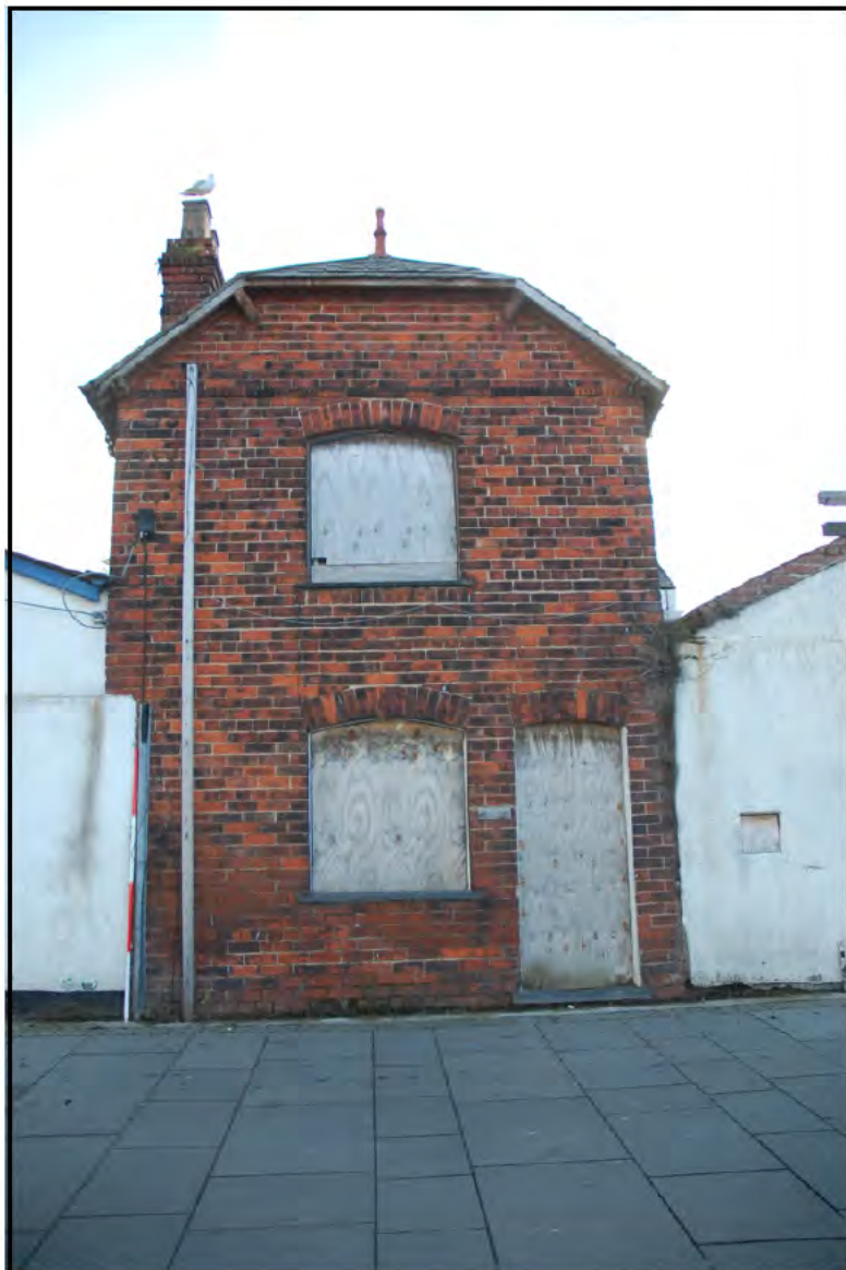
Plate 42: YARD 5 (PRN 30468): Building 05 (PRN 30469): east-facing elevation (quay side): a small two storey building in red brick (English Garden Bond) with a hipped roof of slate with ceramic ridge tiles. (Ranging pole: 1.0m)
