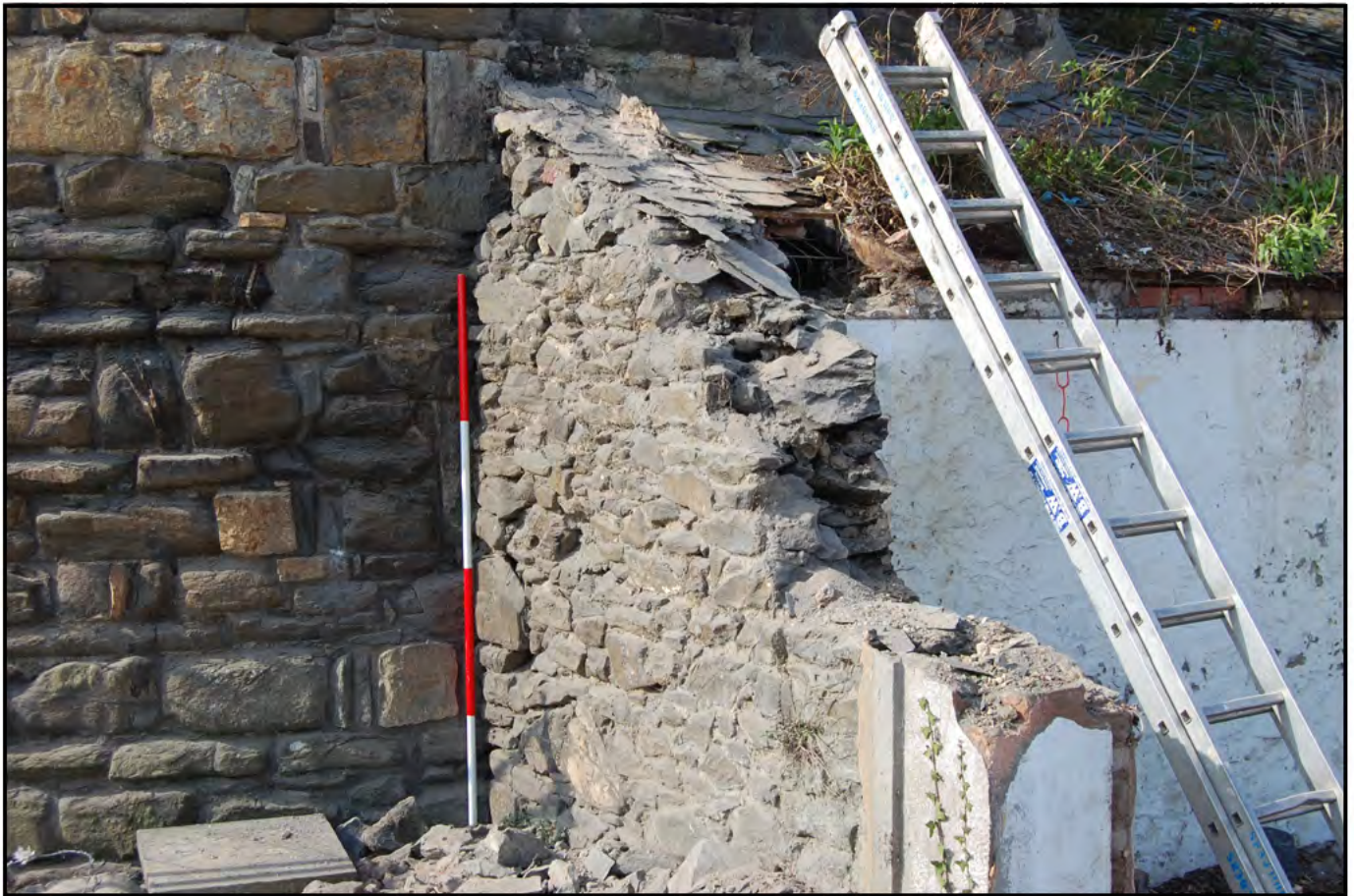
Plate 34: YARD 4 (PRN 30463): Building 14 (PRN 30465): during demolition: the roof of Building 14 was supported on half kingpost trusses of mid 19th century date. The king-posts lay against the town wall, supported on pillars built against the wall. The only part of this build that had insertions into the medieval wall was where the roof structure wrapped around tower 3, where timbers had been inserted into the tower wall. (Ranging poles: 1 x 2.0m and 1 x 1.0m)
