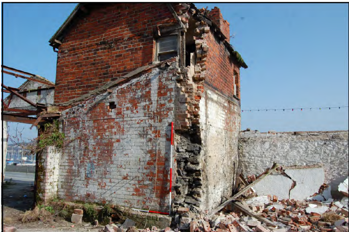
Plate 43: YARD 5 (PRN 30468): Building 05 (PRN 30469): image taken within YARD 5 during demolition phase: the original stone cross-wall (Cross Wall C) that formed the southern boundary of the yard, had been incorporated into the southern elevation of Building 05, with the upper floor built of brick. The former outline of Building 15 (PRN 30471) is visible along the west facing elevation of Building 05.
