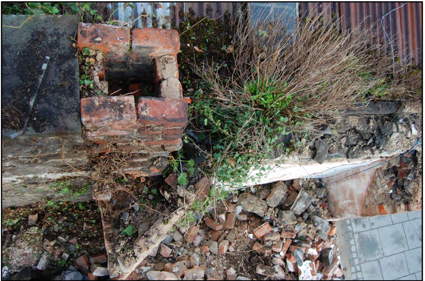
Plate 26: YARD 3 (PRN 30457): Building 13 (PRN 30462): during demolition a brick built chimney was identified built into the stone cross-wall (Cross Wall B) against which Building 13 was built. Birds' eye view during demolition detailing brick-built chimney and stone-built cross wall. (Ranging pole: 2.0m)
