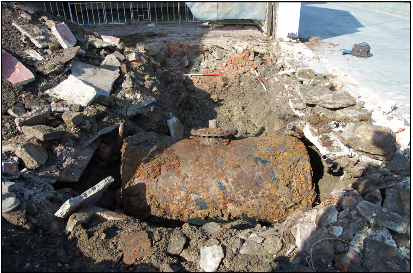
Plate 28: YARD 4 (PRN 30463): A series of redundant buried fuel tanks were identified withn Yard 4 during the demolition phase. The fuel tanks had been installed underground just inside the frontage of the garage (the central building within Building 04 (PRN 30464); cf. plate 26). A total of four tanks were found during the demolition. (Ranging poles: 1 x 1.0m and 1x 2.0m)
