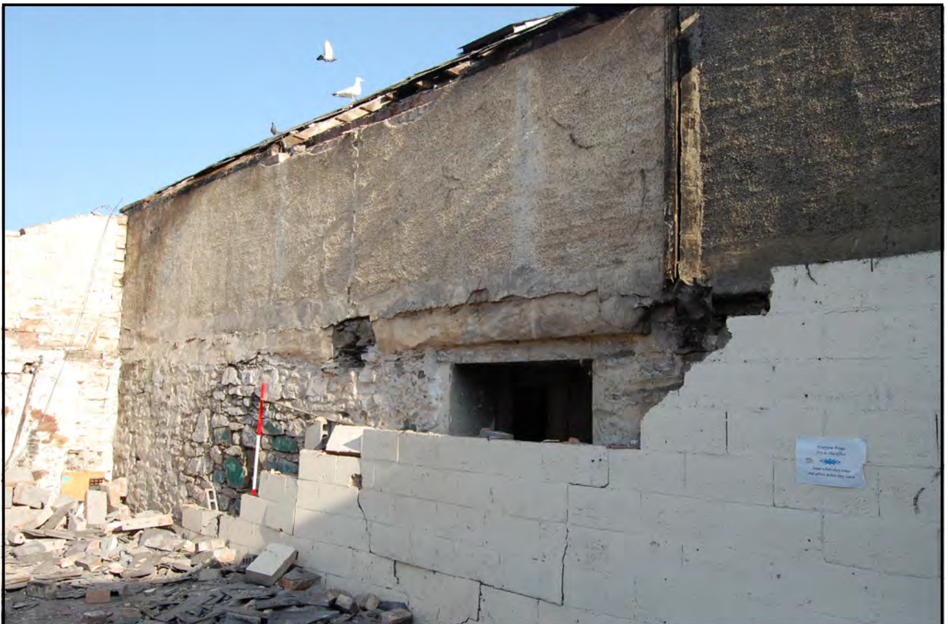
Plate 04: YARD 1/2 (PRN 30451/PRN 30454: Buildings 01 (PRN 30452) and 02 (PRN 30455) : doorway identified in the north elevation of Building 01 during the watching brief phase. The doorway linked Buildings 01 and 02 and was constructed through Cross Wall A. Building 02 was built from thermal blockwork whereas the exterior wall of Building 01 (facing north), covered by Building 02, was rendered, suggesting it was originally constructed to stand alone with Building 02 added later (Ranging pole: 2.0m)
