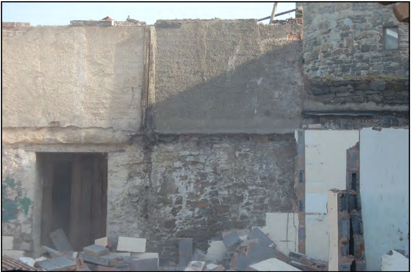
Plate 03: YARD 1/2 (30454): Building 01(PRN 30452): doorway identified in the north elevation of Building 01 during the watching brief phase. The doorway linked Buildings 01 and 02 (PRN 30455) and was constructed through Building 01/Cross Wall A and both buildings functioned as a single business.
