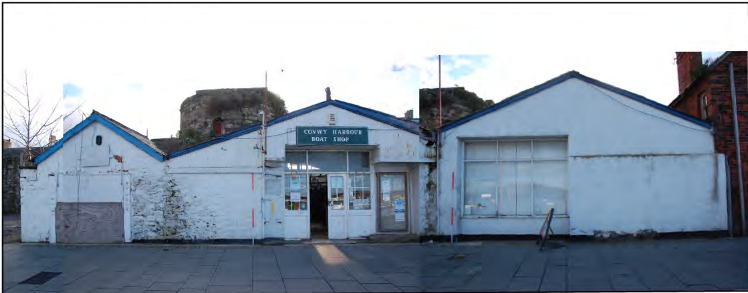
Plate 29: YARD 4 (PRN 30463): Building 04 (30464): composite image detailing the east facing elevation of Building 04. This building occupied the full width of Yard 4 and was extant as three bays. These lay north and in front of an earlier stone building that lay on a north-south axis against the town wall (Building 14 (PRN 30465): plate 33). The north, east and south walls of Building 04 also formed the yard walls, whilst the west wall used the existing east wall of Building 14. Each bay was roofed with a pitched roof running east-west, so the front onto the quay was made up of three gables. The wall fronting the quay partly made use of the earlier Wall A (the enclosure), though parts were rebuilt in brick plate 29. The east and west cross-walls (B and C) between Wall A and the town wall also partly survived in their original form, though had been raised in height from approximately 2.0m to 3.35m plate 22. The cross-walls were seen to abut Wall A. Access into the building was both from the quay and from Yard 3 to the east through wide doors (cf. plate 22)
