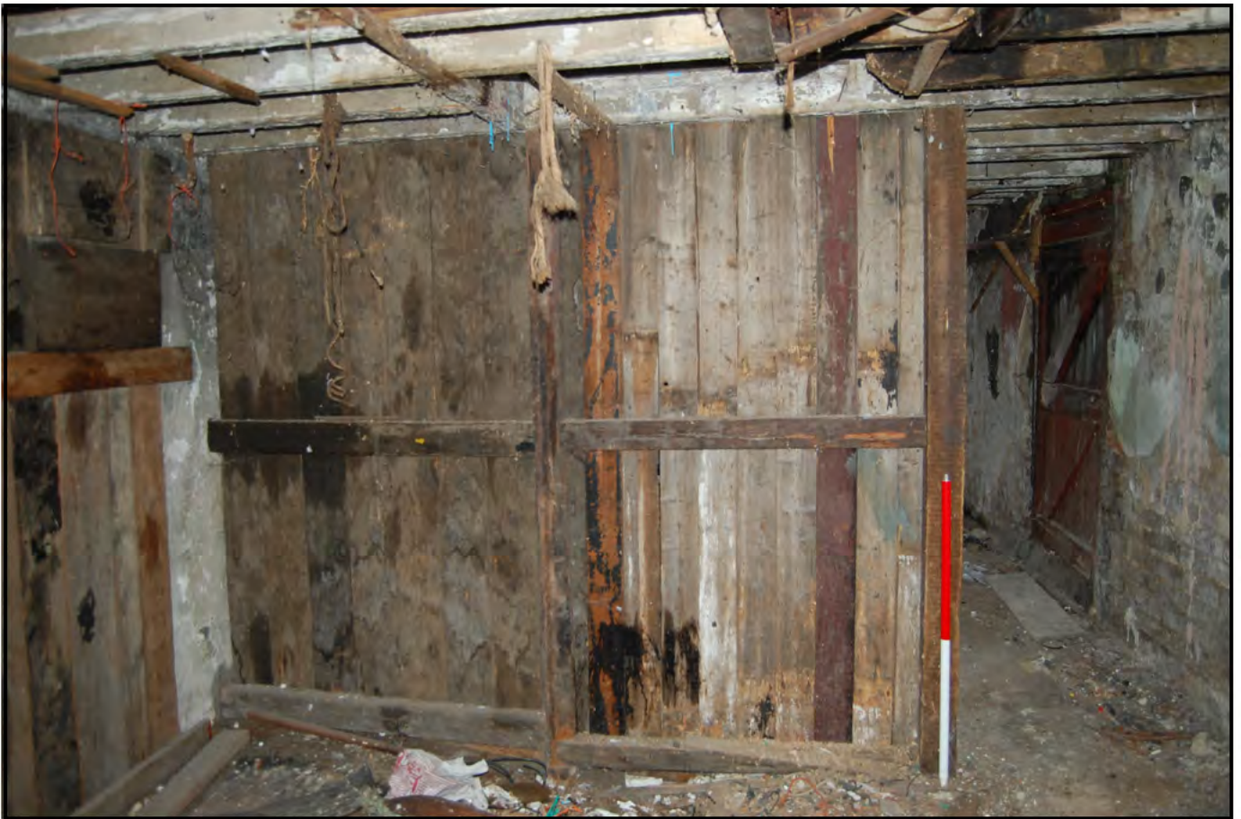
Plate 08: Yard 01 (PRN 30451)/Building 01 (PRN 30452): internal view detailing ground floor. Comprised two rooms divided by a timber partition. Internal walls were rendered, the floor was concrete and the first floor supported on wooden ceiling joists. (Ranging pole: 1.0m)
