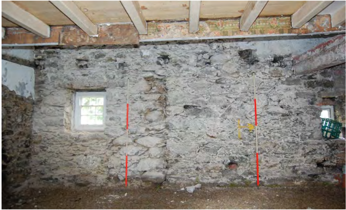
Fig. 8 Straight edge in north west wall indicating earlier phase of construction to the right, extending only to ground floor level. Scales 2 metres.
