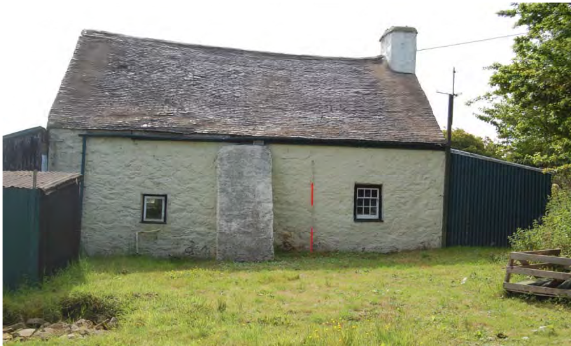
Fig. 19 Rhent from the north west. The 1960s buttress can be seen, along with the division between the two phases of building (near the 2m scale).
