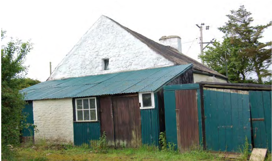
Fig. 17 Corrugated Iron and Brick sheds at north eastern end of the building. The croftlight can be seen above.
