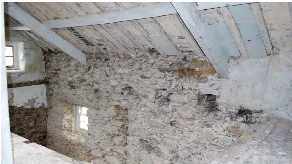
Fig. 9 First floor of north west wall showing smaller rubble masonry above level of straight joint and rafter holes for late 19 th century floor insertion.
