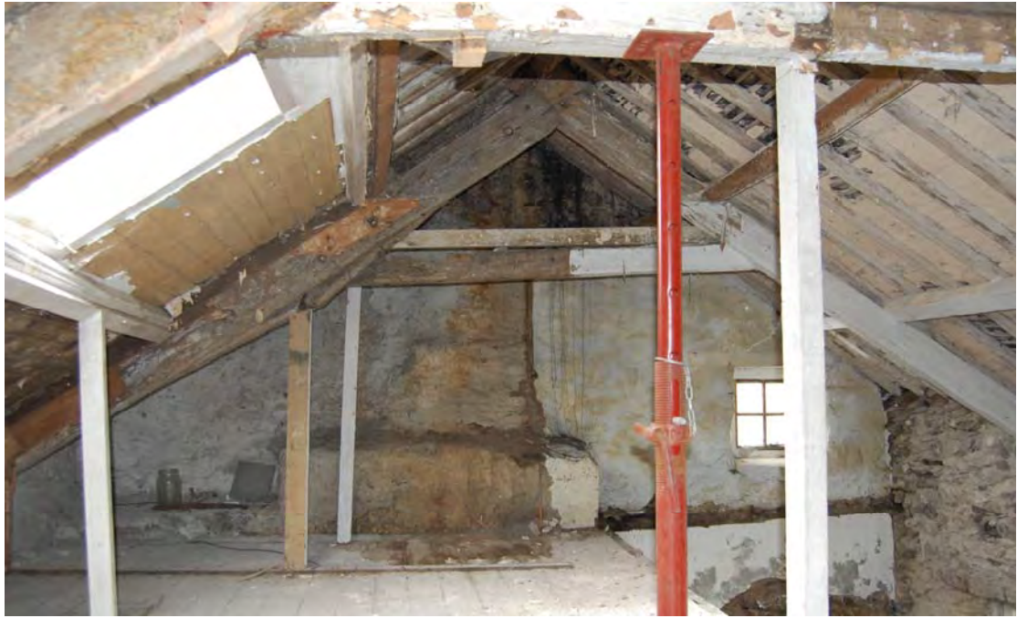
Fig. 10 The surviving Roof Structure of Rhent, showing wooden pegged principal rafters.
