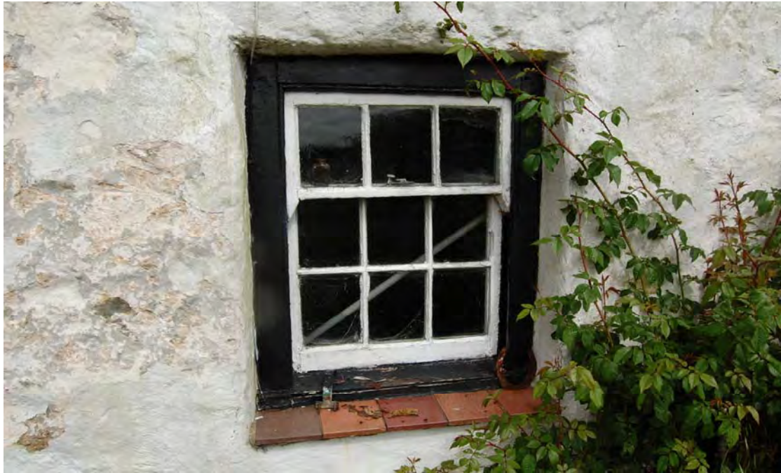
Fig. 14 Nine paned horned sash window
