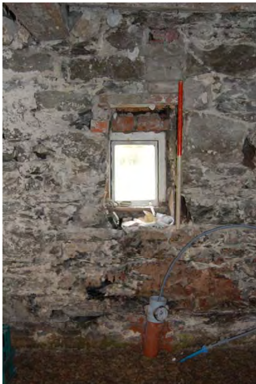
Fig. 15 Window at northern end of north west wall, showing infilled former slit opening above.
