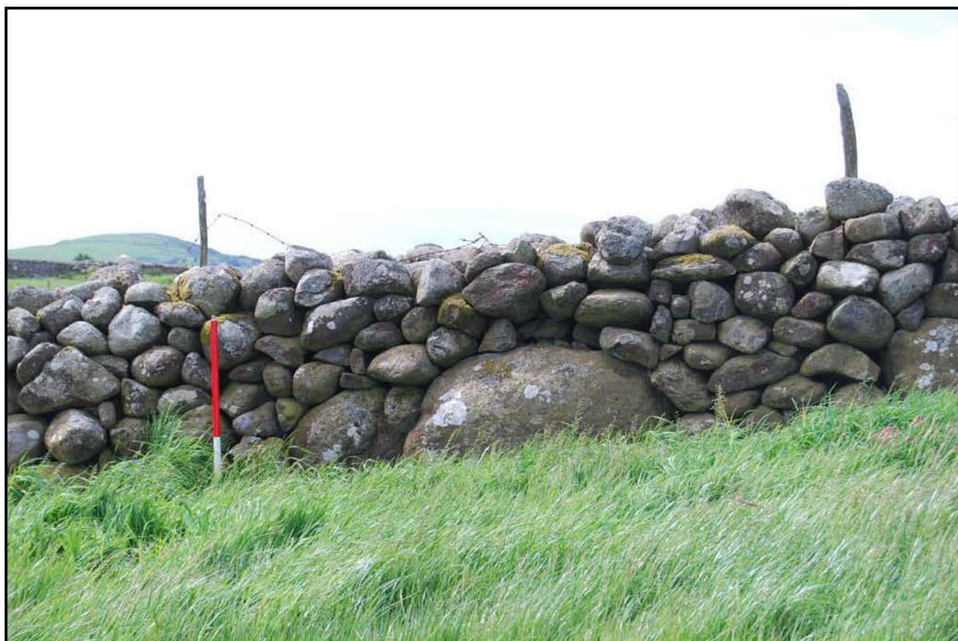
Plate 5. North facing section of boundary wall showing stone coursing and material size
