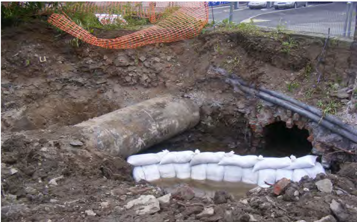
Fig. 6 The breached brick arched culvert (14) with concrete overflow pipe to the south. Facing South-West
