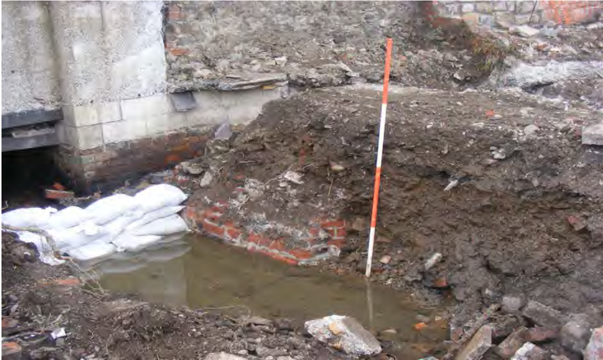
Fig. 7 Remnant of Brick waste tank at eastern end of culvert
