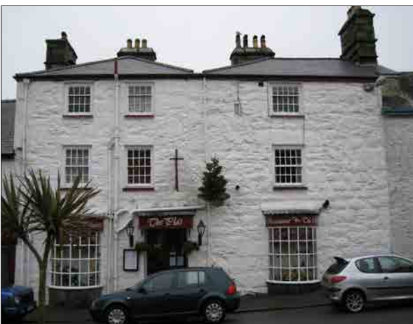
Plate 33. This view of the Plas Restaurant shows the early lateral chimney on the right, and the use of typical sash windows inserted c. 1830 when the earlier house was converted into the Blue Lion Inn.
