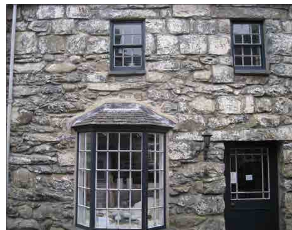
Plate 27. Several buildings show evidence of former paint or limewash, including the Pottery, Pentre'r Efail.
