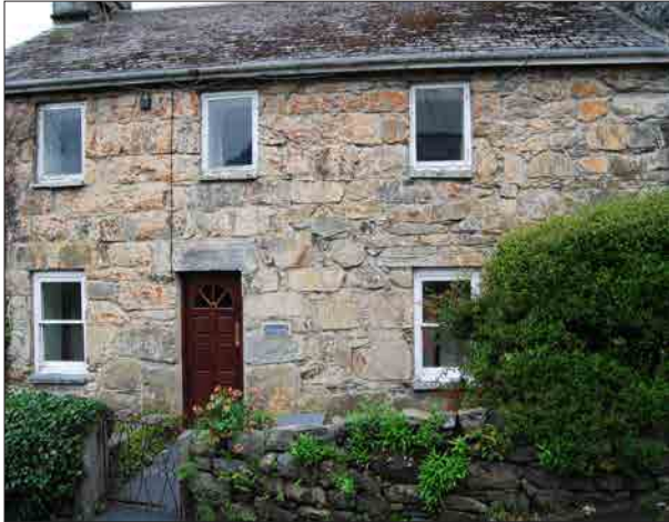
Plate 41. Caereinion, Penllech. The uncoursed masonry on the right is earlier than the roughly coursed masonry on the left.
