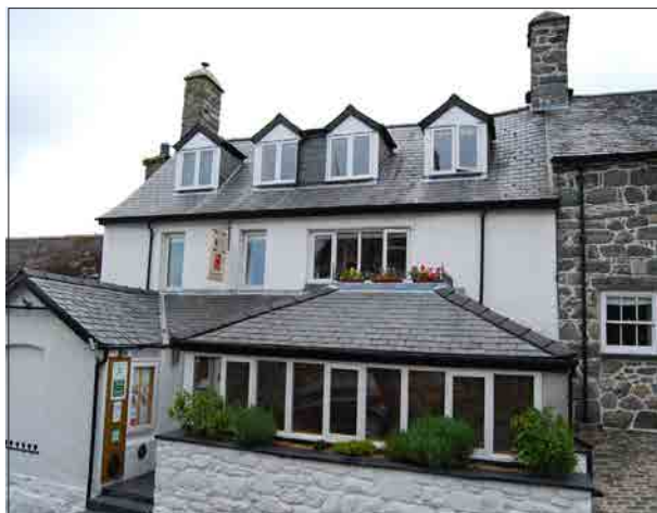
Plate 7. Behind the modern front of the Castle Croft Hotel can be seen the end chimneys and steep roof of the earlier building.
