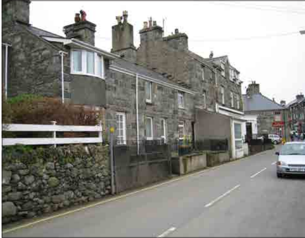
Plate 10. The Glyn Cywarch estate developed land adjacent to the new road in the 1840's. The fronts are of coursed masonry blocks, but the sides and rear are of uncoursed rubble masonry. The three-storey buildings quickly drop down to two-storey away from the square.
