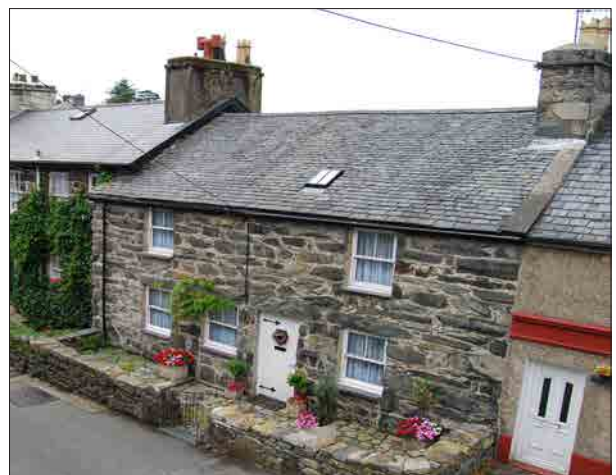
Plate 30. A later example of slates laid in diminishing courses at Pentre'r Efail.
