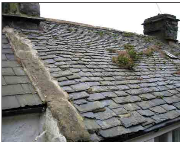
Plate 29. The roof at Siambr Wen with the slates laid in diminishing courses.
