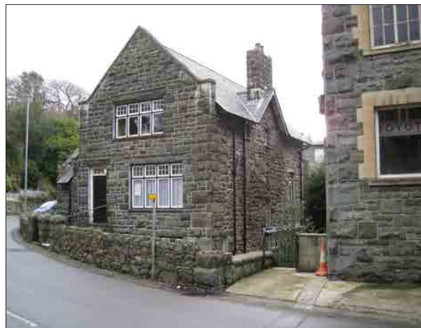
Plate 24. The front of the Institute is snecked masonry, though the sides are of rubble masonry.
