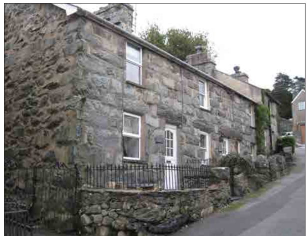
Plate 22. An example of roughly coursed rubble masonry from the 19th century (Pentre'r Efail).
