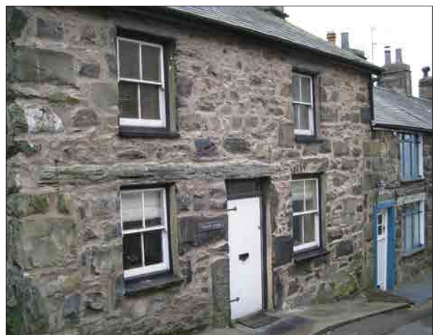
Plate 34. An example of the later four-pane sash window at Tryfar.
