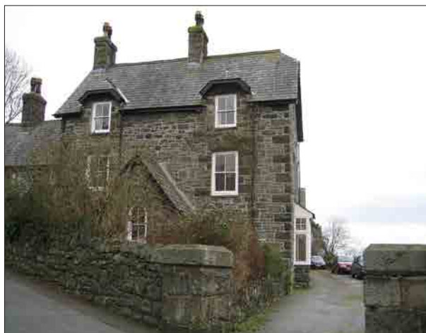
Plate 25. The end of Bronwen Terrace shows Holland's preference for uncoursed rubble with heavier quoins.
