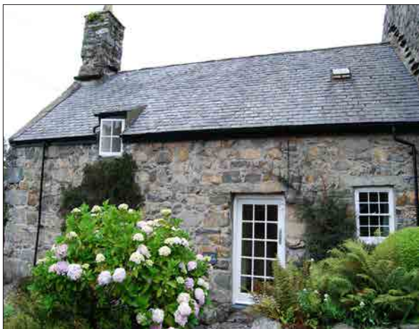
Plate 21. Rubble walling and squared quoins can be seen at Ty'r Felin, Penllech.
