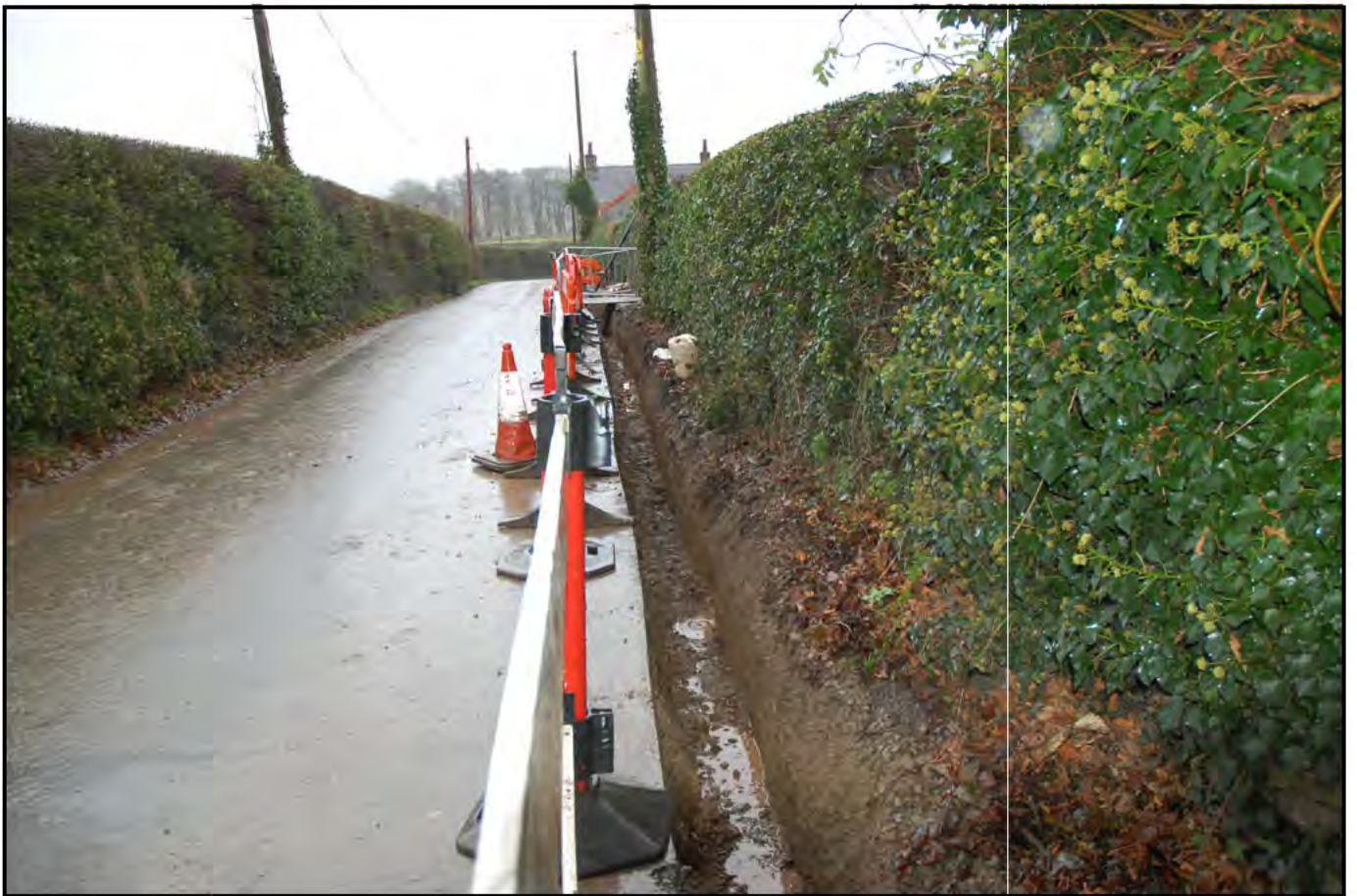
Plate 07: Ducting trench for sewer replacement project. Location: northwestern end of the project detailing full excavation depth
