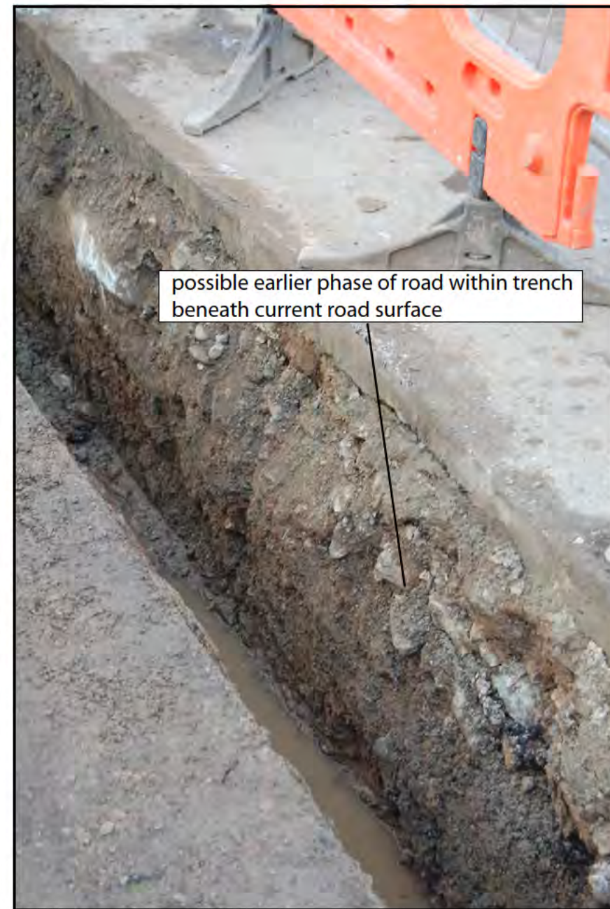
Plate 08: Ducting trench for sewer replacement project. Location: Cae Mawr cottages; the ducting trench contained deposits of glacial drift beneath a layer of rough stones. The stone-rich deposit was interpreted as possibly part of an earlier phase of road
