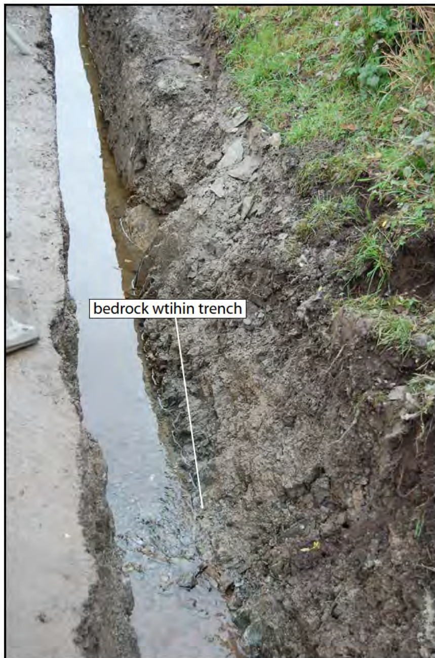
Plate 07: Ducting trench for sewer replacement project. Location: northwestern end of the project; bedrock extant at a depth of 0.20m below the existing road surface
