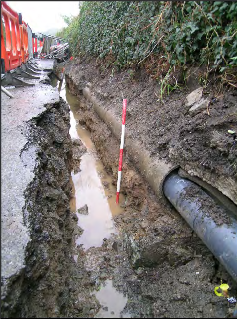
Plate 03: Ducting trench for sewer replacement project. Location: c.490.0m northwest of the 'Siwgr Plum' nursery, a storm drain encapsulated in concrete pipe (View South)
