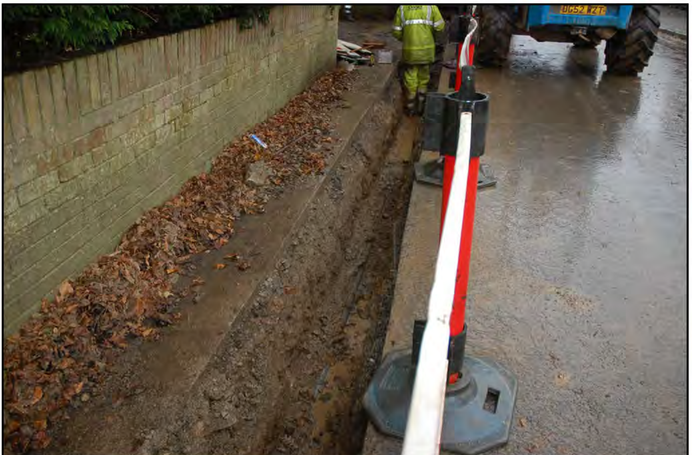
Plate 08: Ducting trench for sewer replacement project. Location: northwestern end of the project detailing full excavation depth and existing utilities at base of trench. The ducting trench was completed at this location.
