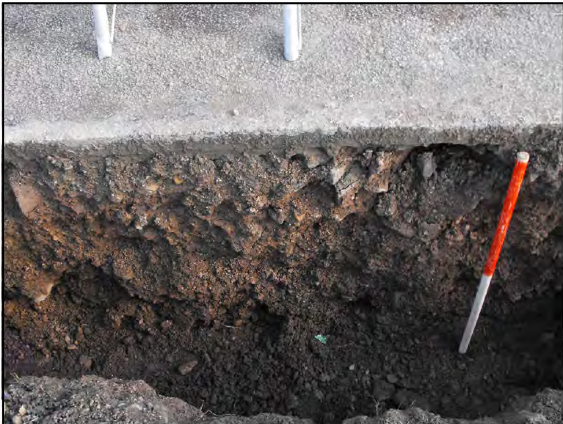
Plate 02: Ducting trench for sewer replacement project. Location: entrance to Bryn Celli Ddu car park. Full excavation depth with exposed stratigraphy; identified as road foundation material
