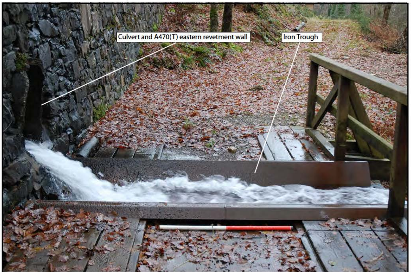
Plate 01: View south of Feature 4, culvert and trough.
