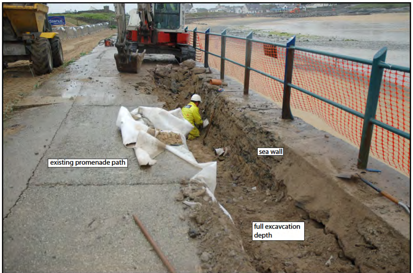
Plate 07: excavation at northern end of the promenade; note the reduced level of excavation (1.2m to 1.5m below ground level); construction of sea wall as before (Plates 03 to 06) but degraded sheet piles not extant; excavation material below path included foundation material and sand
