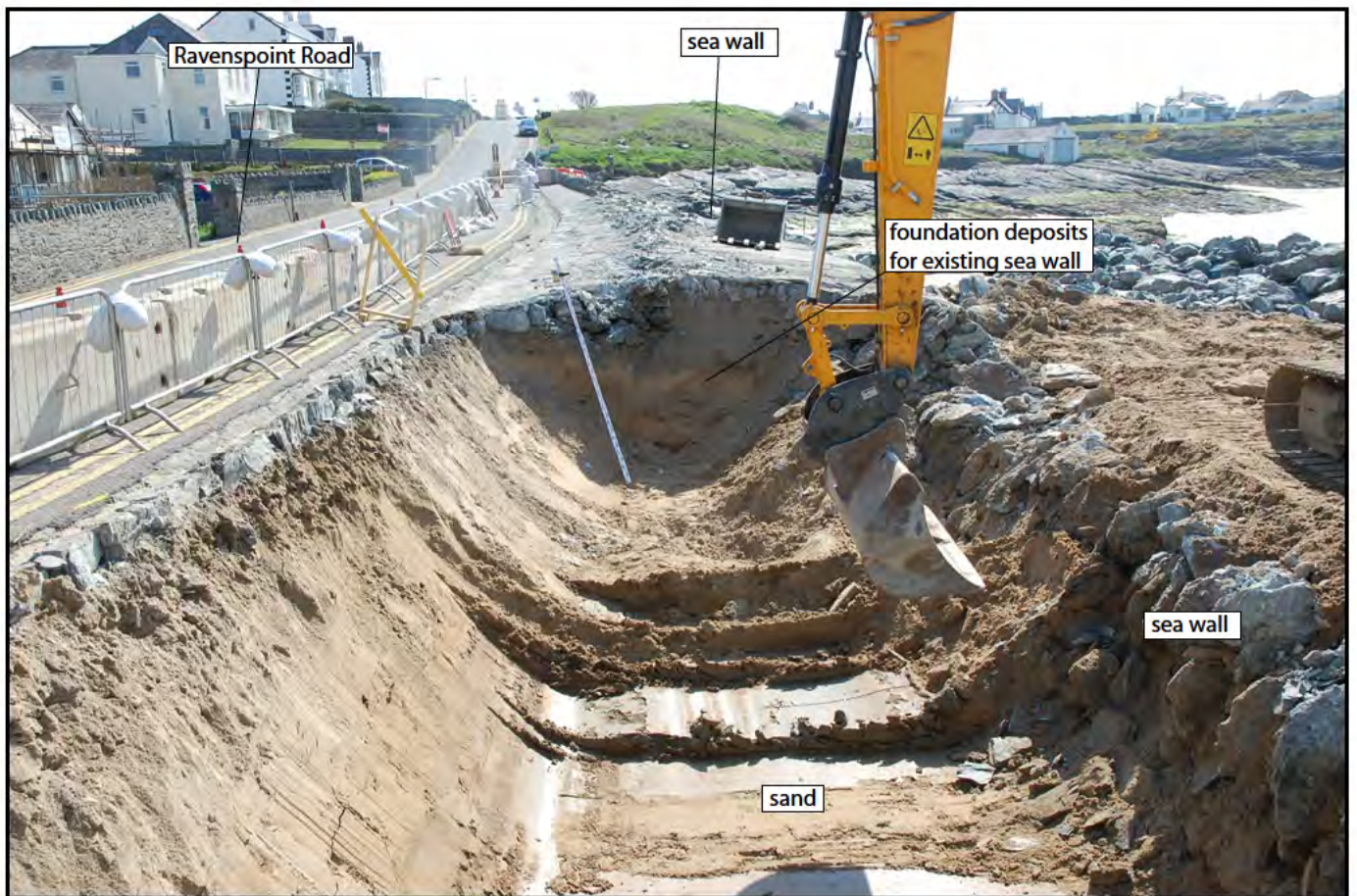
Plate 11: Ravenspoint Road - detail of existing sea wall during excavation. The sea wall was built on sand and sealed with concrete
