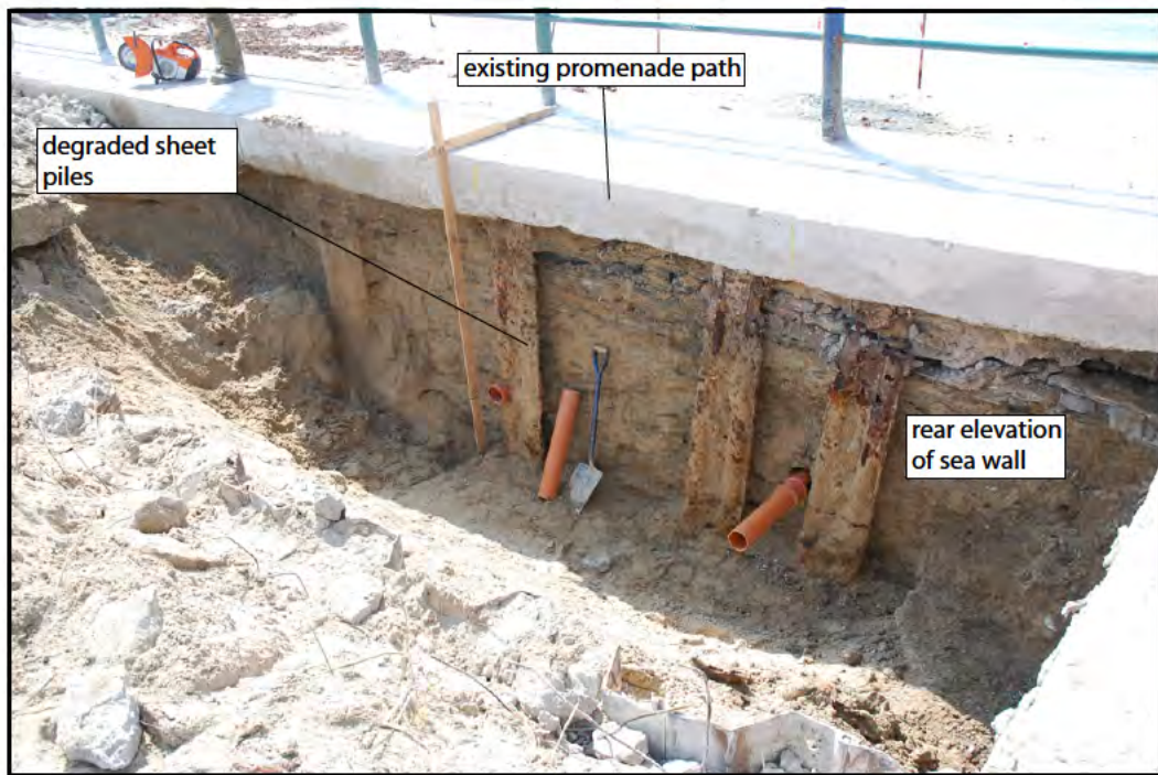
Plate 03: promenade path excavation bay detailing full excavation depth with existing sea wall rear elevation exposed; note degraded sheet piles attached to rear elevation and new drainage pipes
