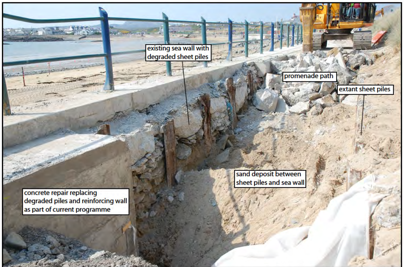
Plate 05: excavation of promenade path detailing existing structural material; note sheet piling on left of image denoting edge of path, also the thick sand deposit between the sheet piles and the sea wall; note also the reinforced concrete on the right of image that replaced degraded sheet piles as part of current works programme
