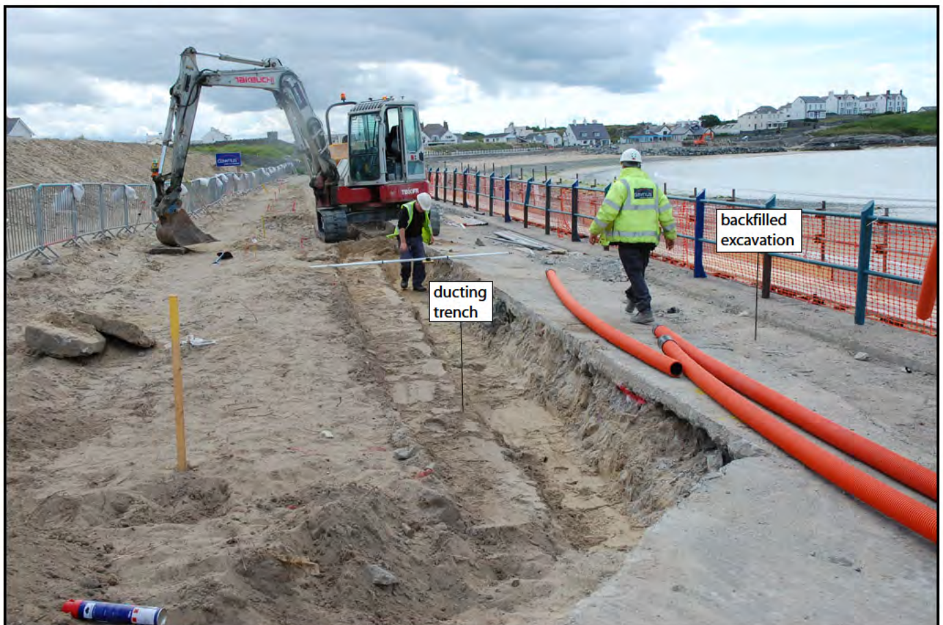
Plate 07: excavation at northern end of the promenade; note the reduced level of excavation (1.2m to 1.5m below ground level); construction of sea wall as before (Plates 03 to 06) but degraded sheet piles not extant; excavation material below path included foundation material and sand
