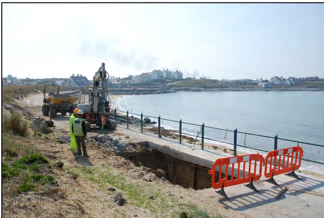
Plate 02: view southwest of the promenade during the excavation of a twelve-metre long "bay"
