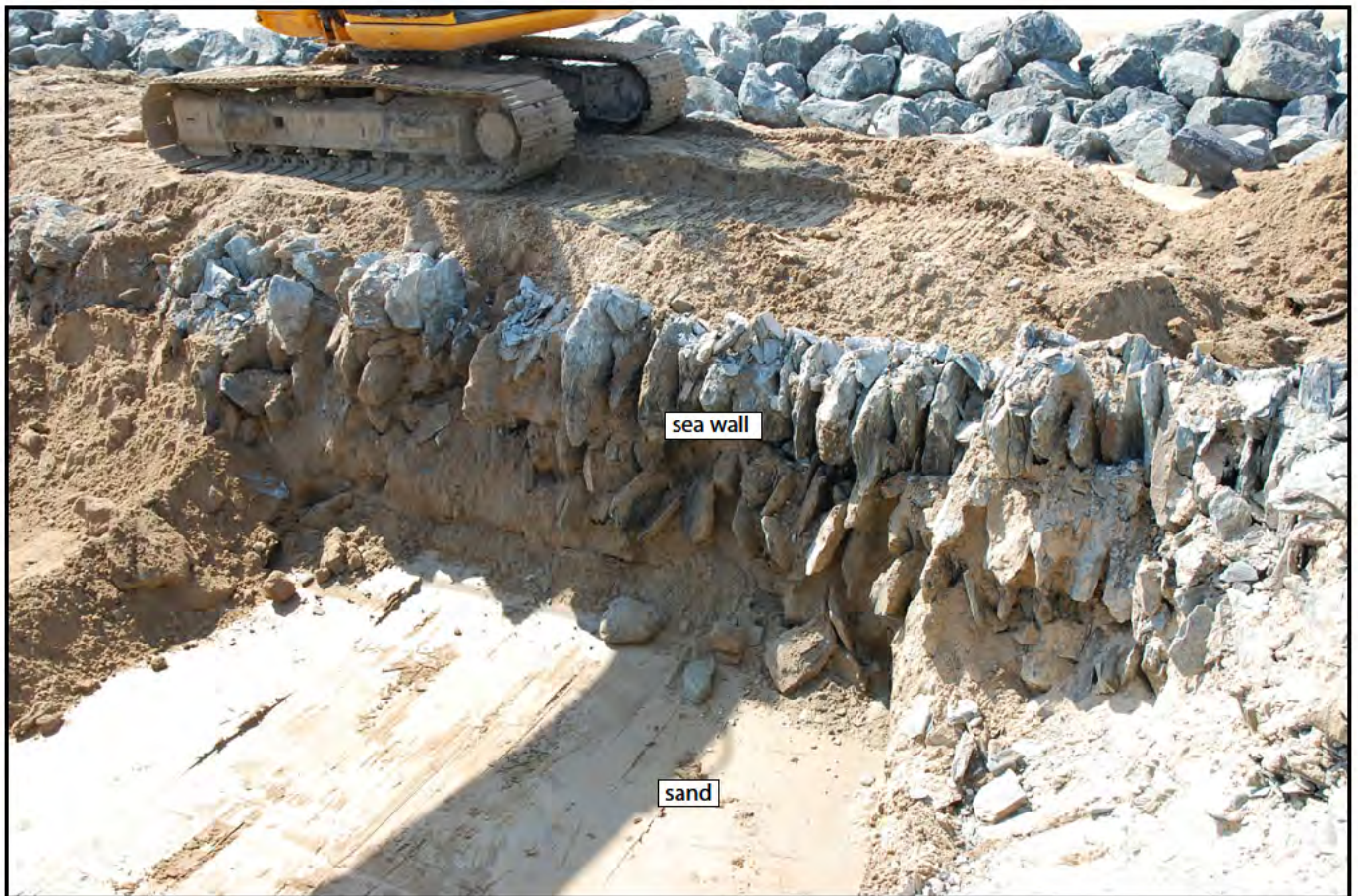
Plate 09: Ravenspoint Road - excavation of existing sea wall
