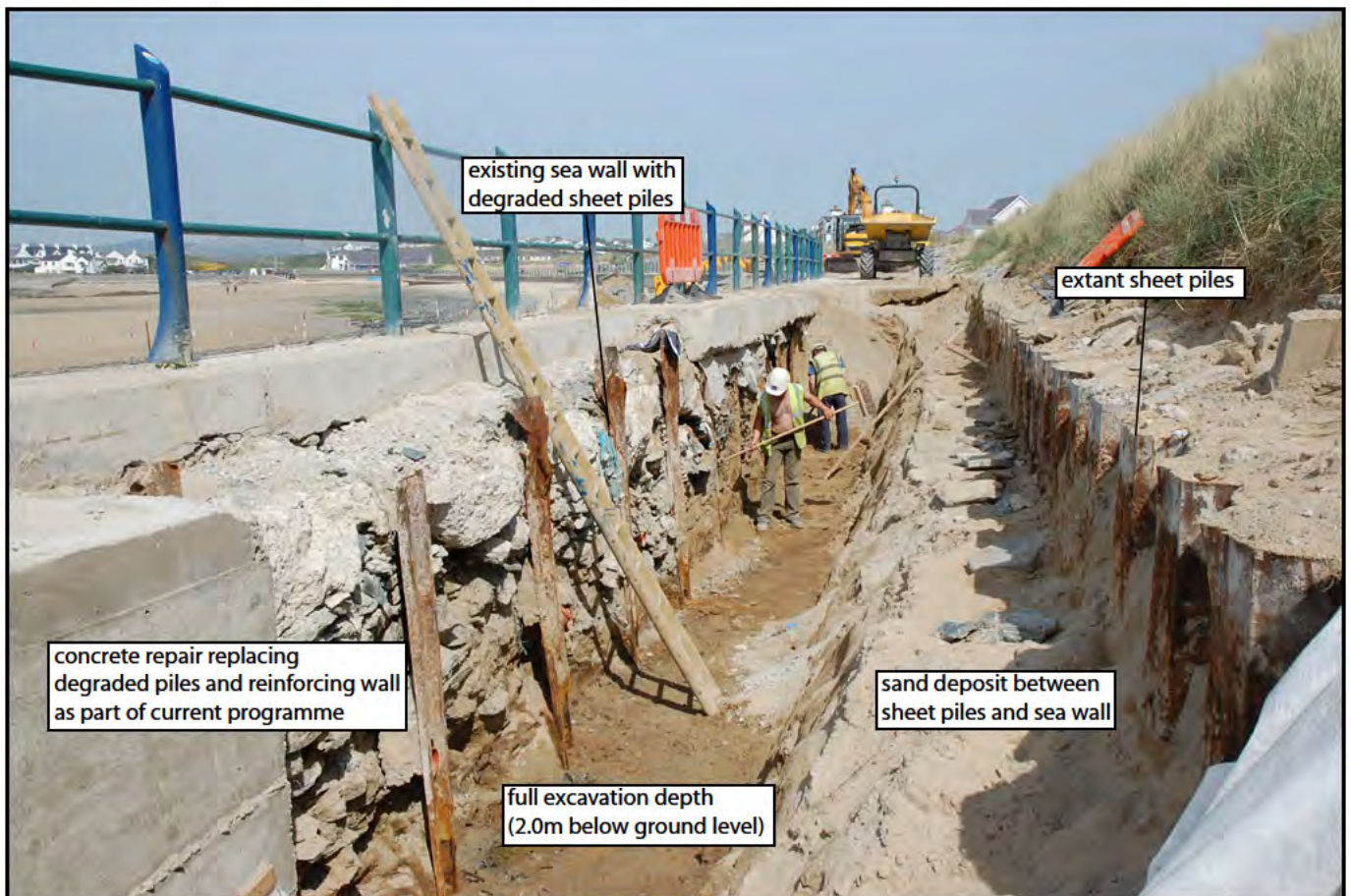
Plate 05: excavation of promenade path detailing existing structural material; note sheet piling on left of image denoting edge of path, also the thick sand deposit between the sheet piles and the sea wall; note also the reinforced concrete on the right of image that replaced degraded sheet piles as part of current works programme
