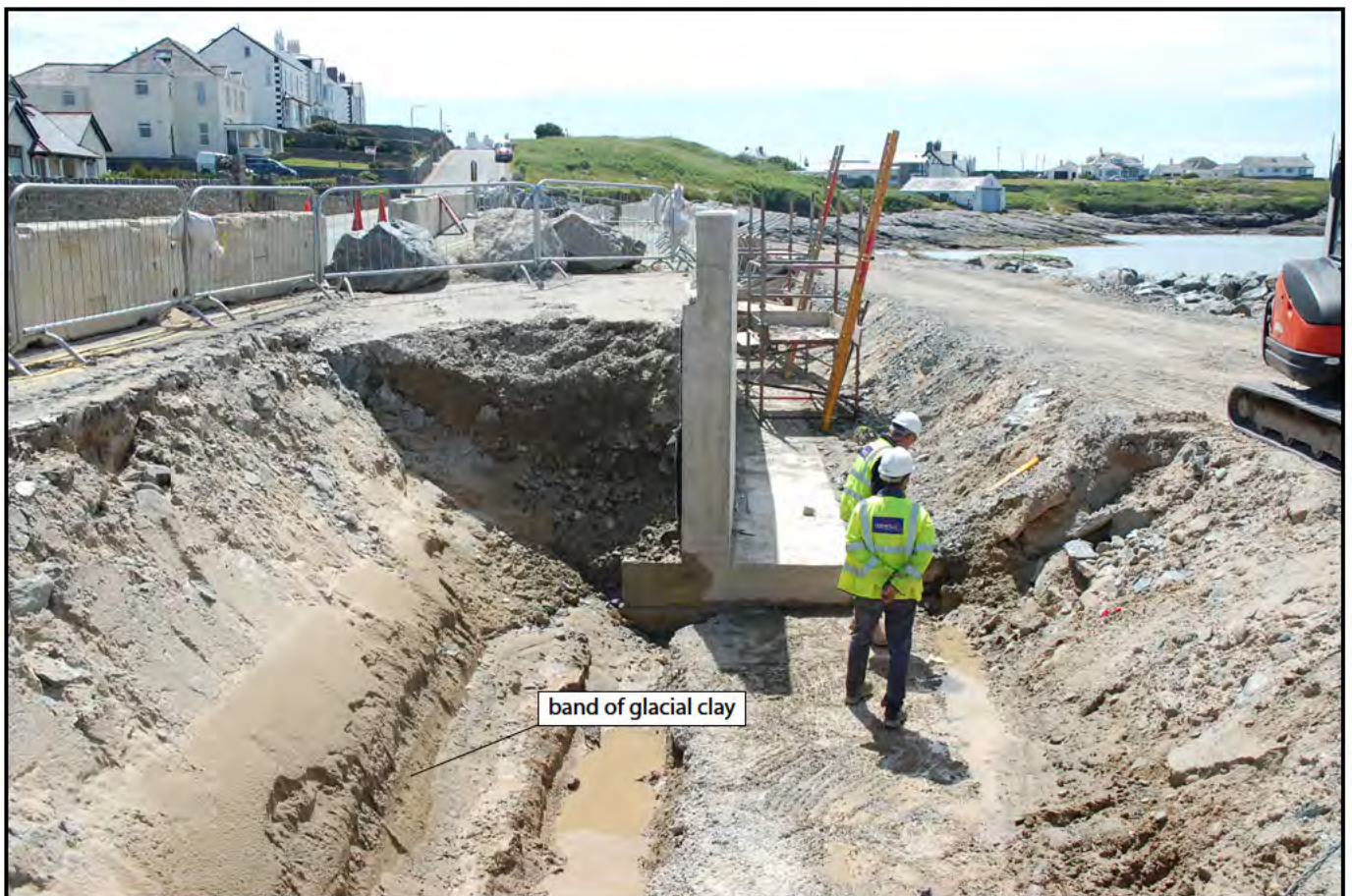
Plate 12: Ravenspoint Road - construction phase for new sea wall detailing full excavation depth (2.0m) and reinforced concrete wall; a band of glacial clay was identified at the limit of excavation
