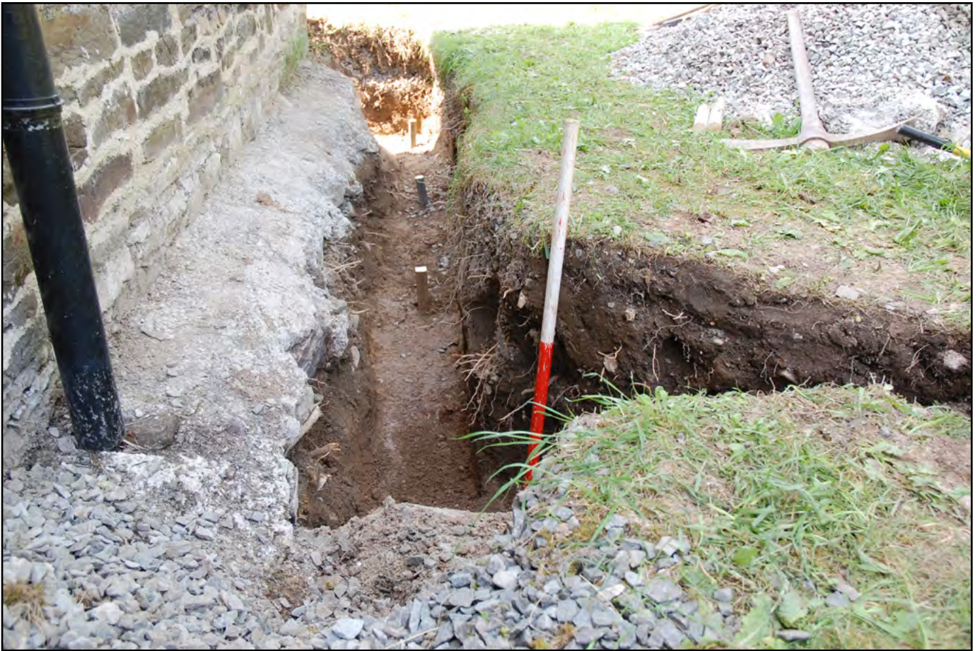
Plate 03: Location of sump and start point of new drainage trench
