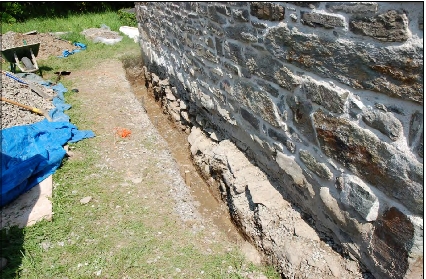
Plate 02: View of groundworks area along west facing elevation. Note foundation course
