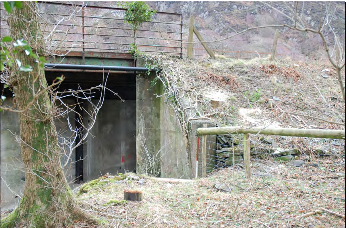
Plate 16: detail of short concrete abutment attached to north facing elevation. Measures up to 4.97m in height and 4.06 in length
