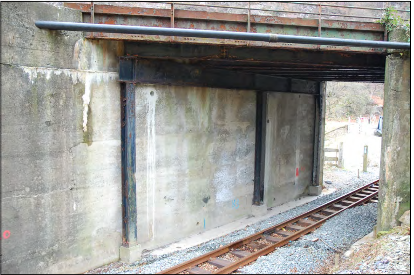
Plate 15: detail of steel girders supporting bridge superstructure
