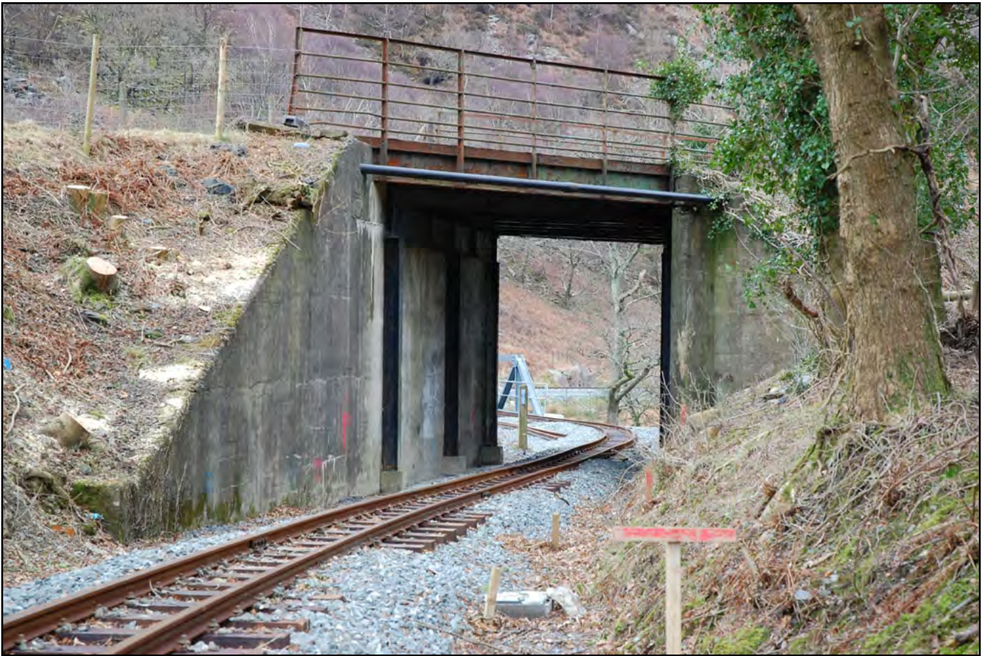
Plate 13: close-up of north-facing elevation prior to demolition, detailing steel parapet, road plate, concrete abutment and steel girder shell
