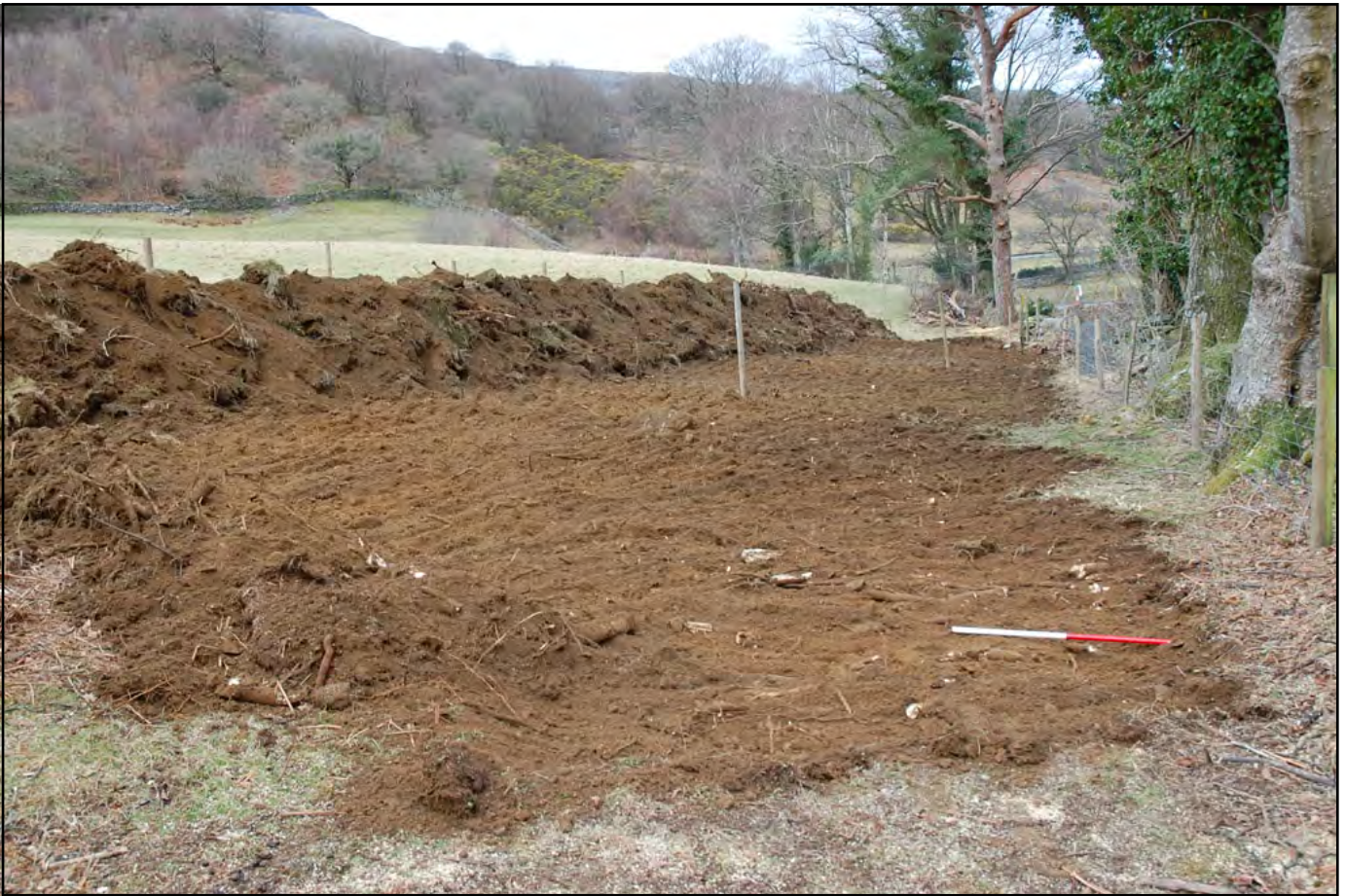
Plate 05: view north of temporary relief road area during excavation. Note the shallow excavation depth; a geotextile membrane was placed over this area and the road surface on top
