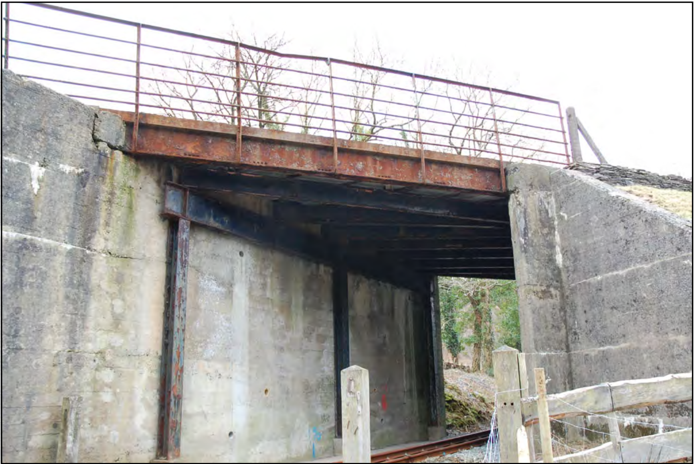
Plate 19: detail of steel girders supporting road plate and existing parapet
