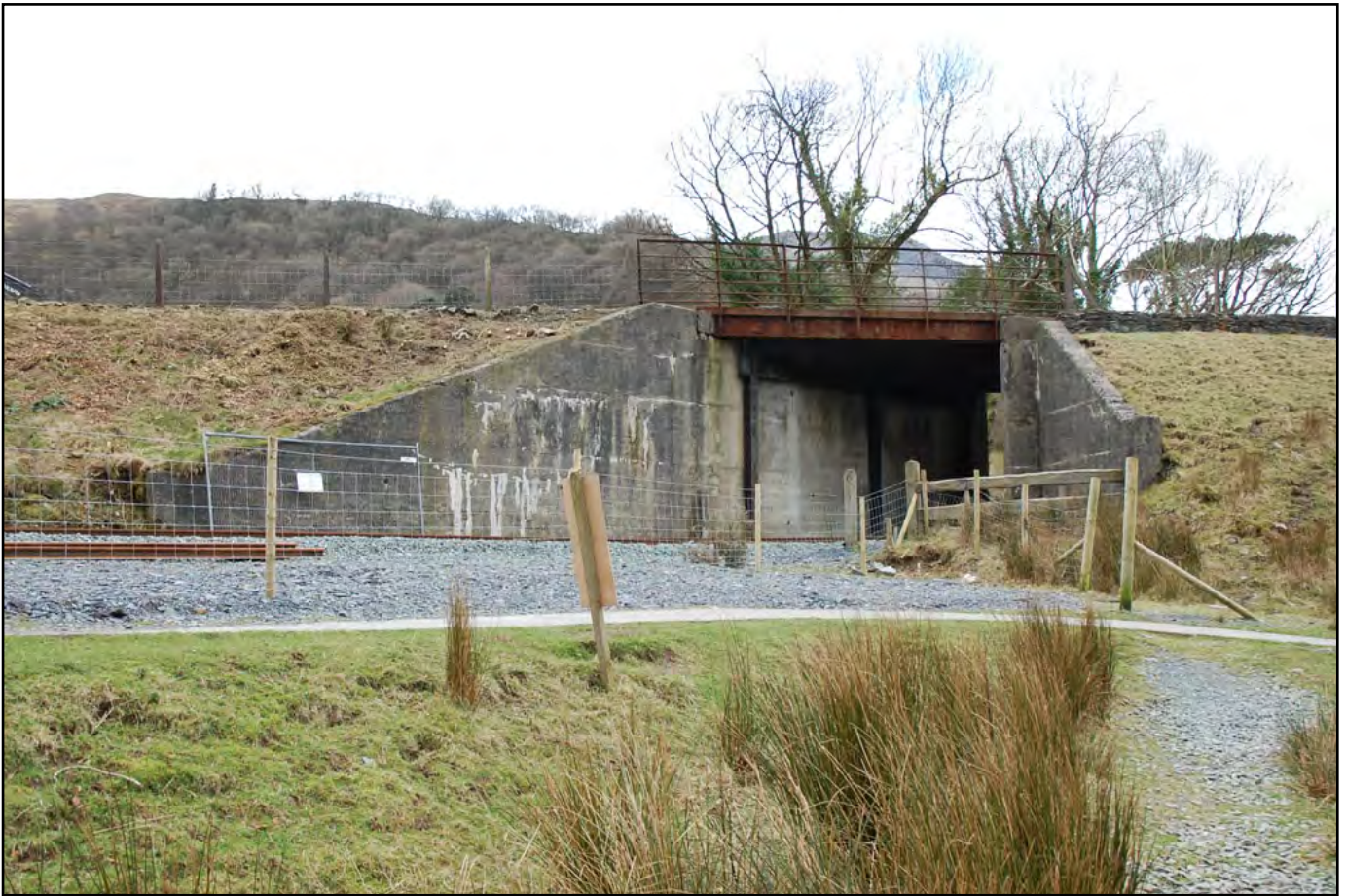
Plate 17: south-facing elevation comprising two concrete abutments, steel girder shell, road plate and steel parapet
