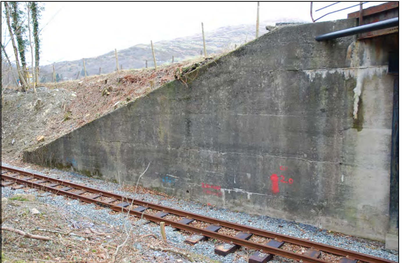
Plate 14: close-up of concrete abutment attached to north-facing elevaton. Measures 4.97m in height and 12.2m in length
