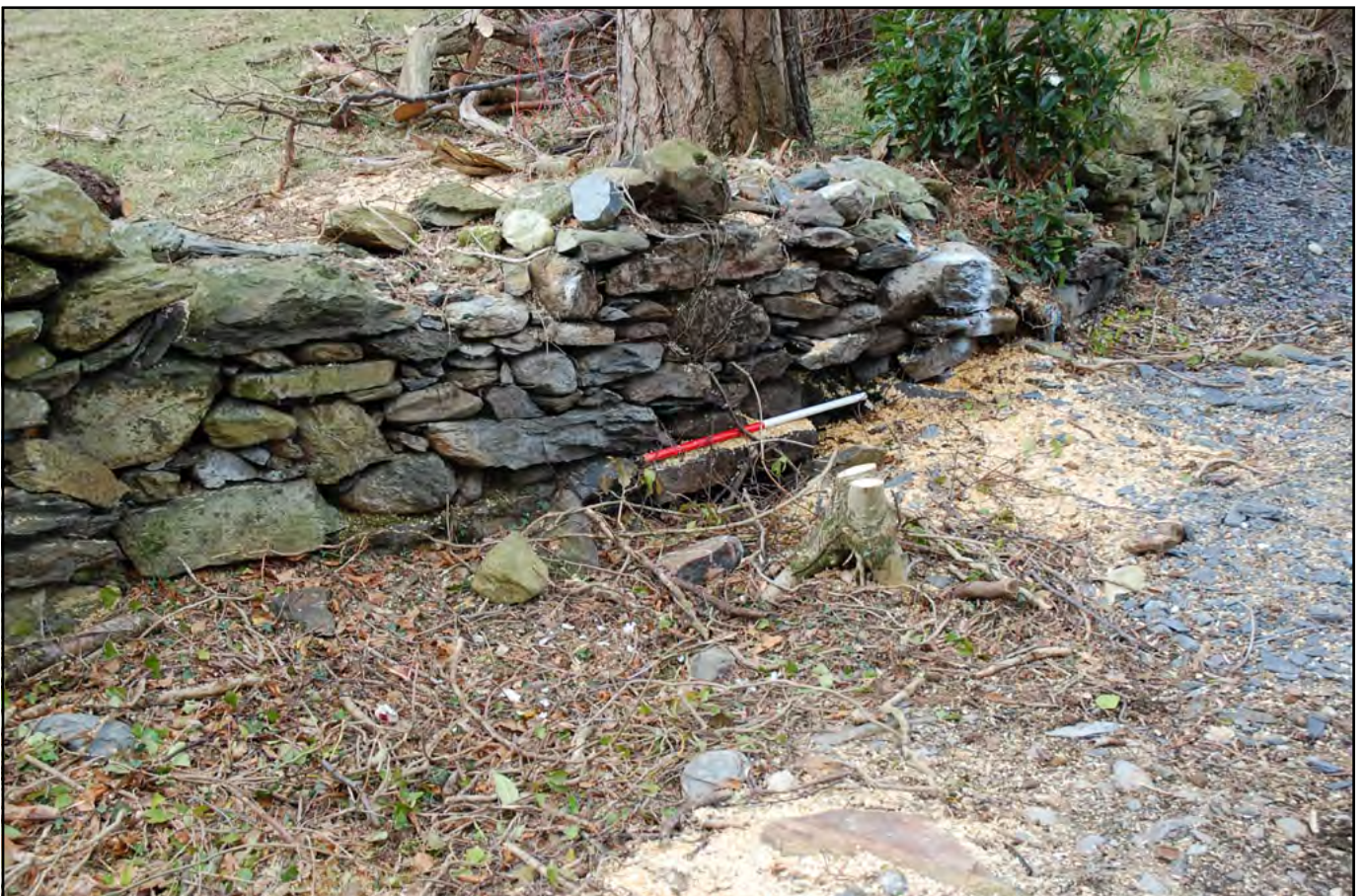
Plate 08: view west of boundary wall prior to breach. Ranging pole is positioned across a stone-built culvert incorporated into the wall
