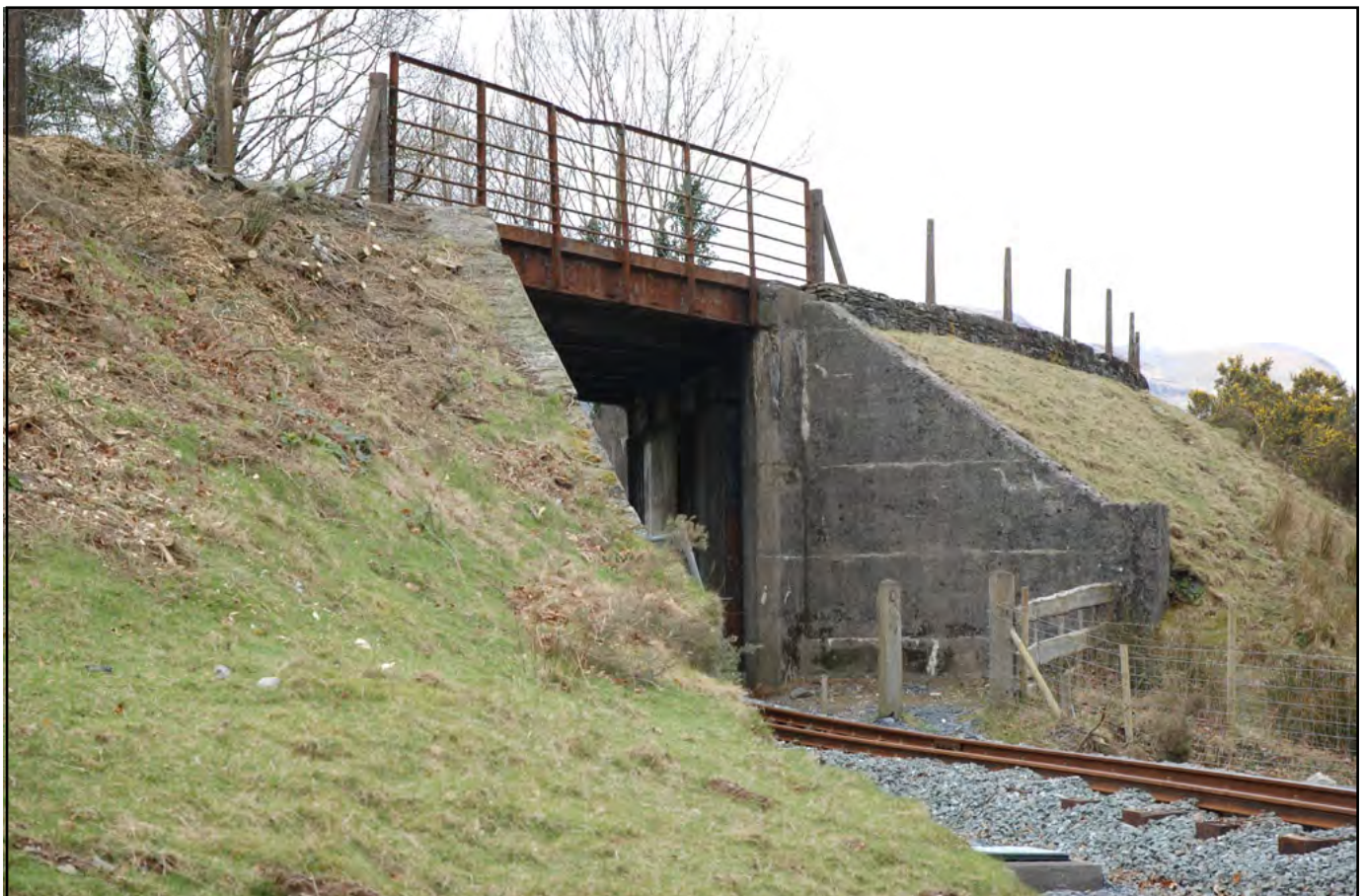
Plate 18: short concrete abutment attached to south-facing elevation. Measures 4.97m and 3.26m in length
