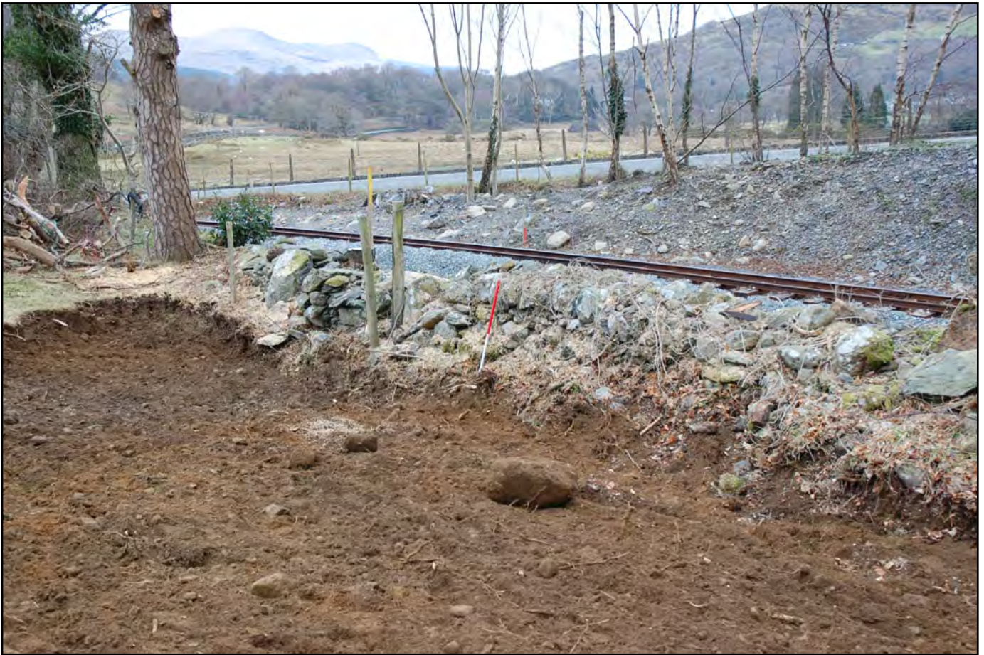
Plate 07: view northeast of temporary relief road. The ranging pole is positioned against a boundary wall that was breached during works to allow the relief road to cross the railtrack
