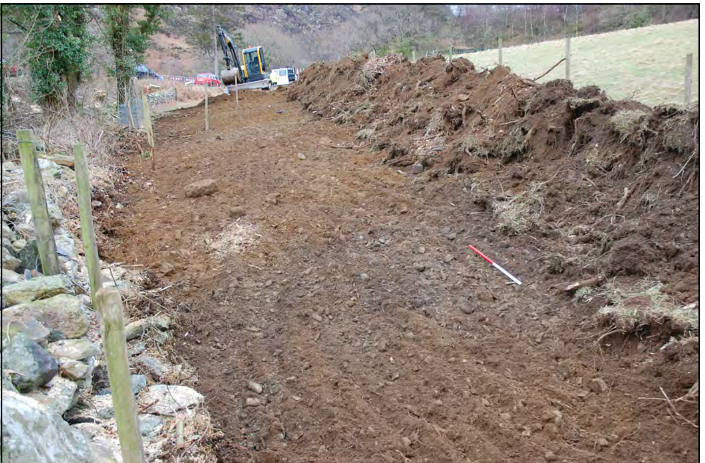
Plate 05: view north of temporary relief road area during excavation. Note the shallow excavation depth; a geotextile membrane was placed over this area and the road surface on top
