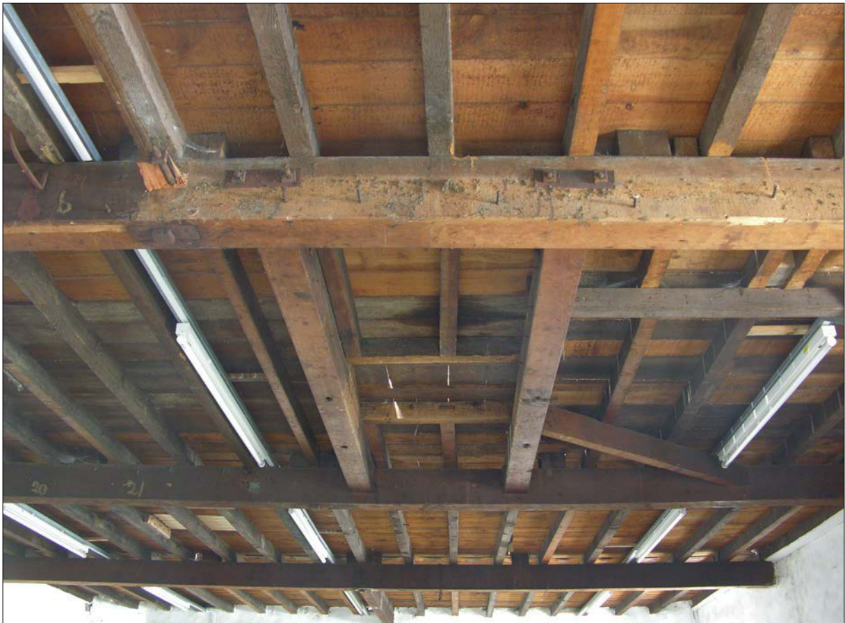
Fig. 20. North warehouse: attic beams, joists and trap access.
