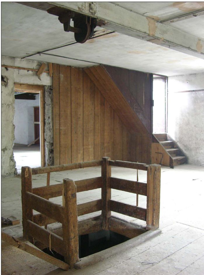
Fig. 40. South warehouse - first floor pulley, trap-door and attic stair
