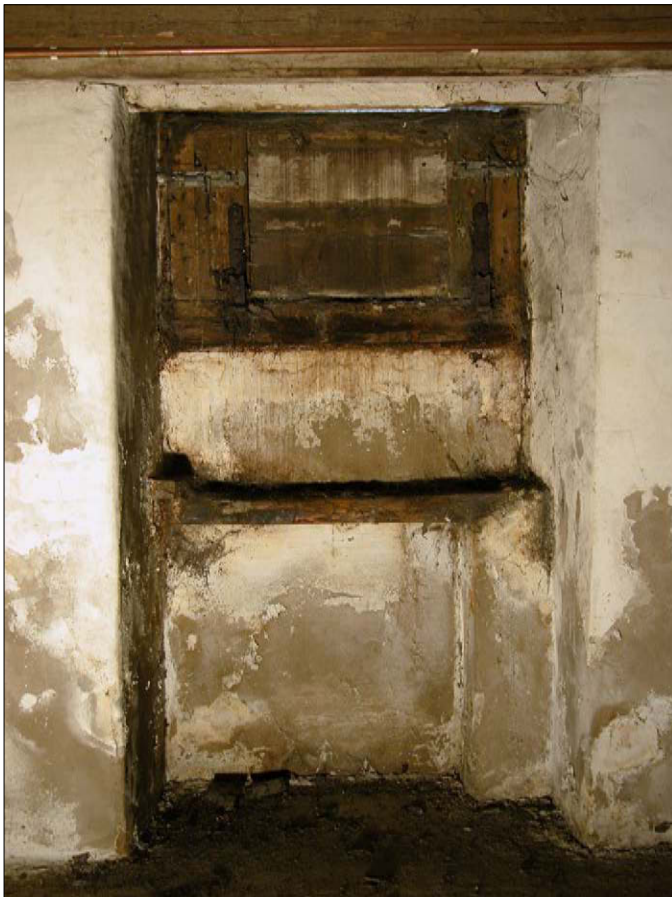
Fig.36. South warehouse - basement chute
