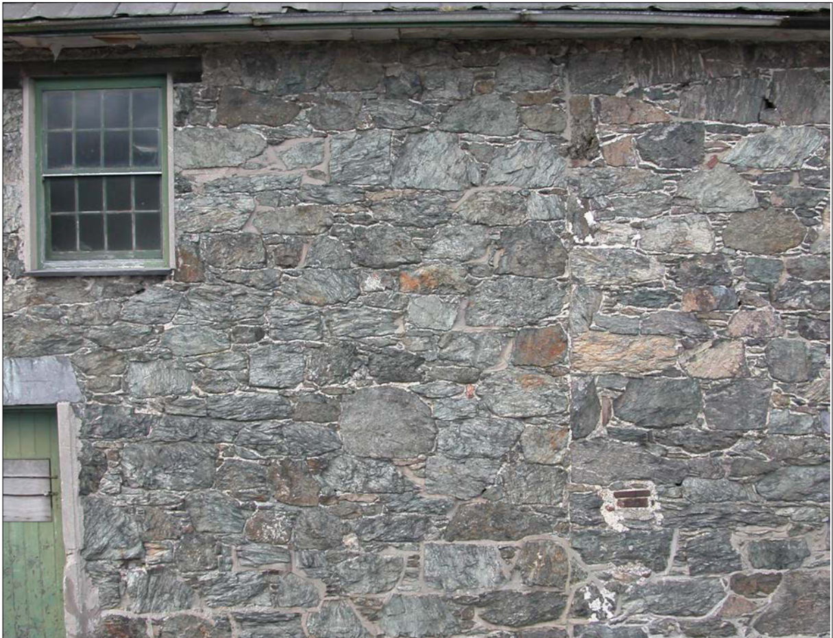
Fig. 22. North and south warehouses: butting join visible
