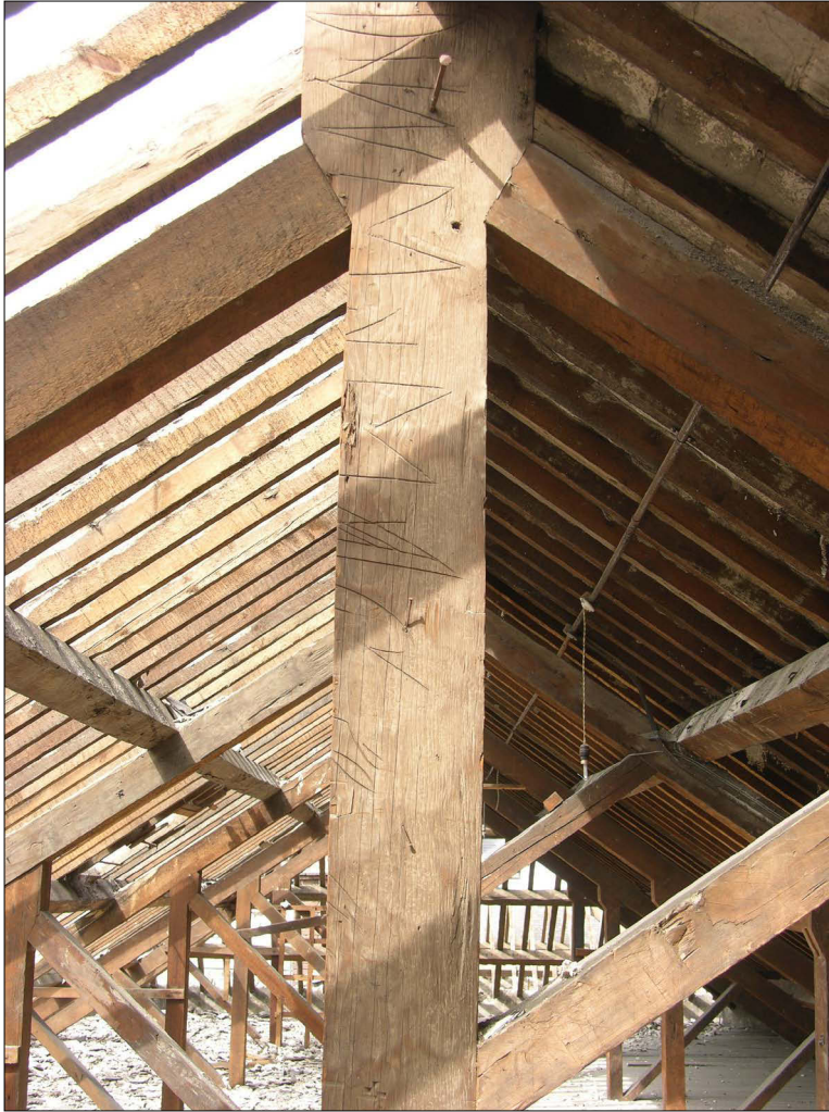
Fig. 52. Shipping marks on timber in main warehouse roof and on basement beams
