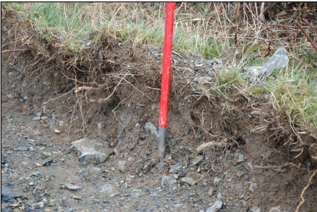
Plate 04: Chainage CH0425: Full excavation depth. Note the appearance of slate waste fragments within the section and at the base of the excavation area. This material represents the foundation layer of the modernised road and verge and was found at this depth throughout the watching brief.
