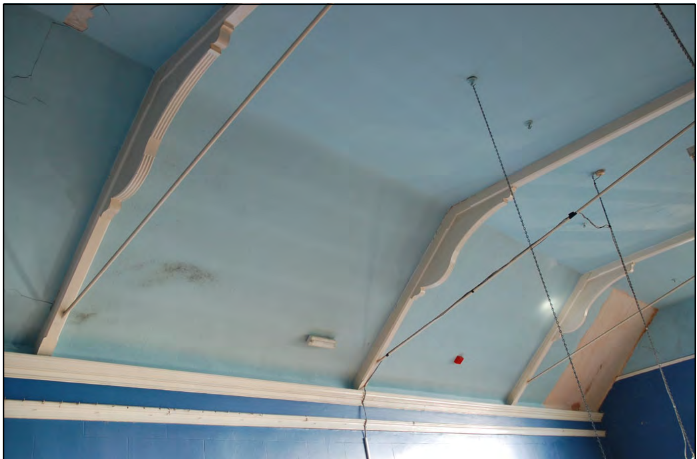
Plate 76: First Floor: Room F03: Roof trusses with moulded details
