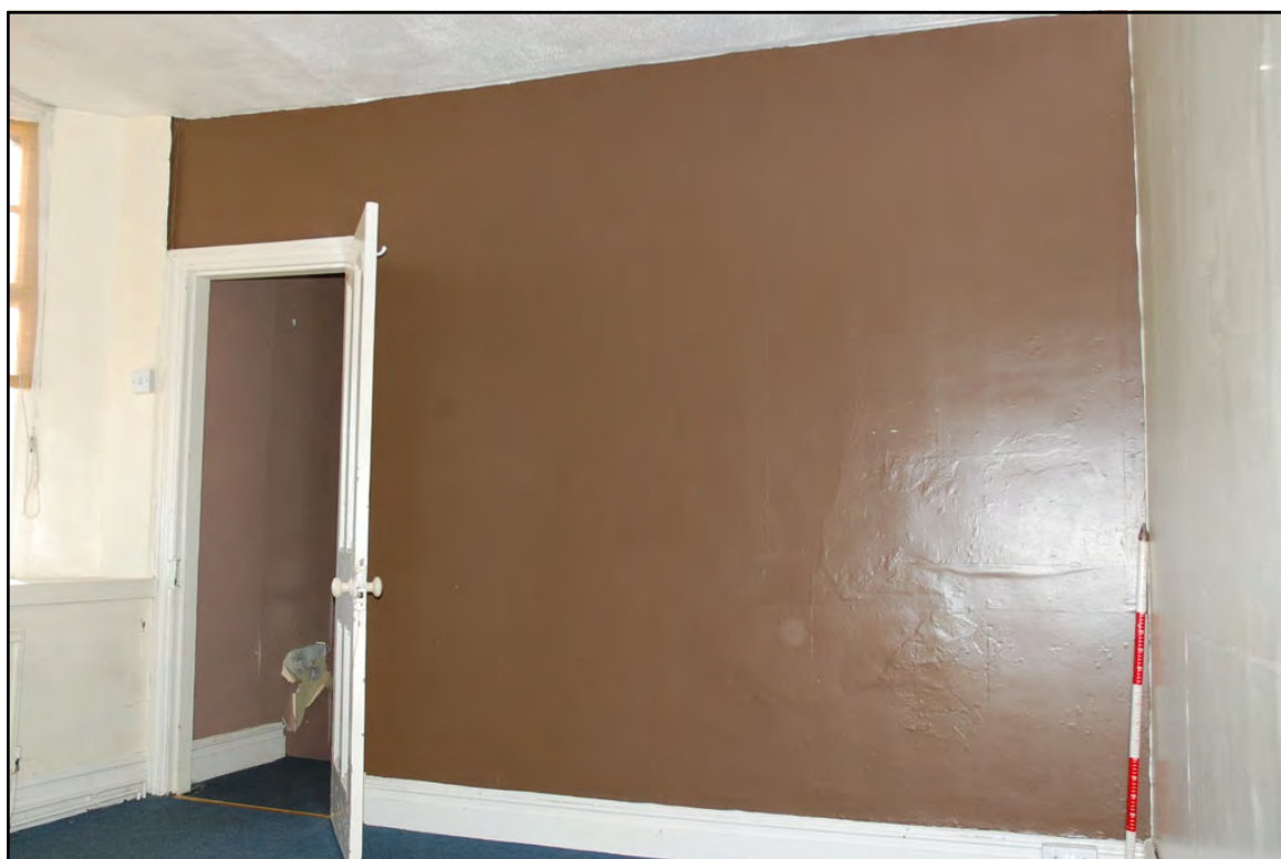
Plate 94: Second Floor: Room S02. Door D31 is open. Original moulded skirting; no crown moulding
