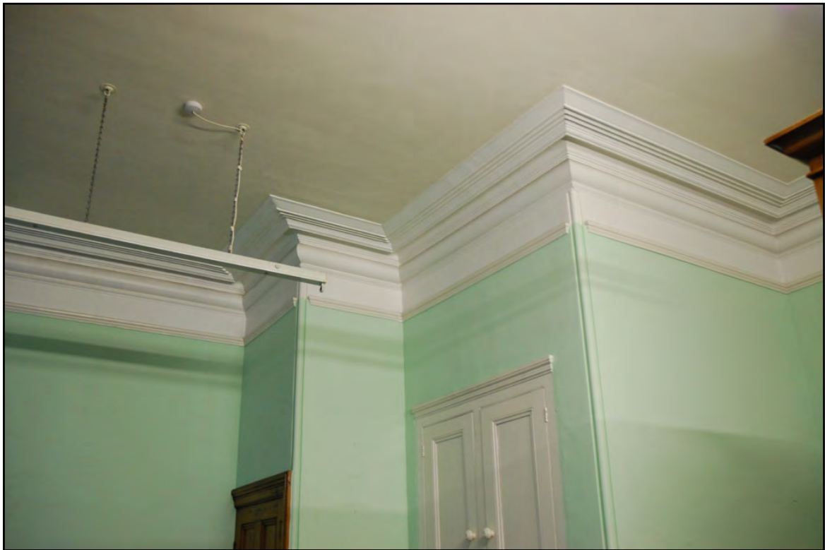
Plate 55: Ground Floor: Room G12: Crown moulding detail
