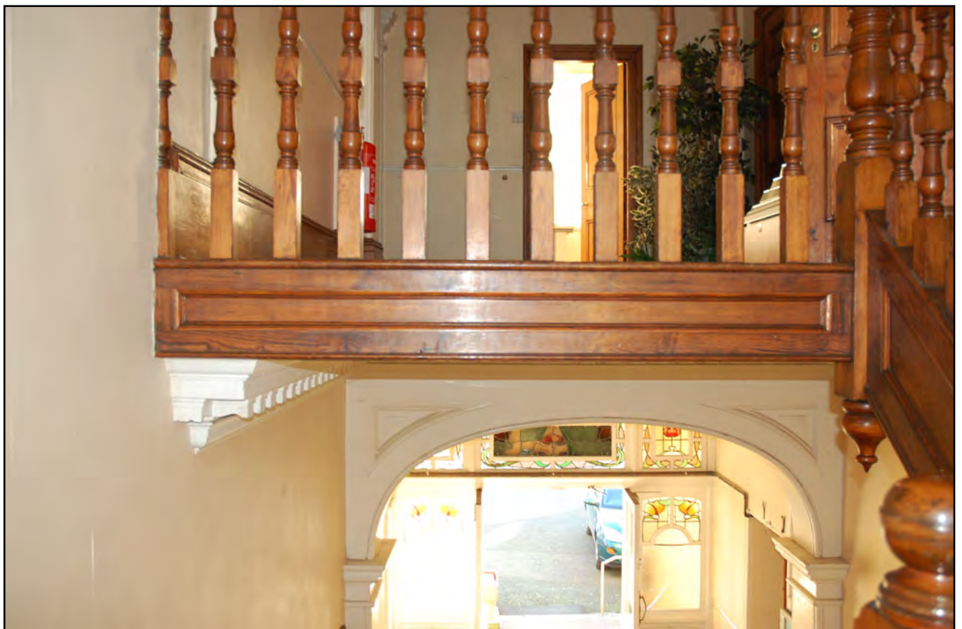
Plate 64: Staircase with view of arch moulding for G02 and crown moulding for landing support
