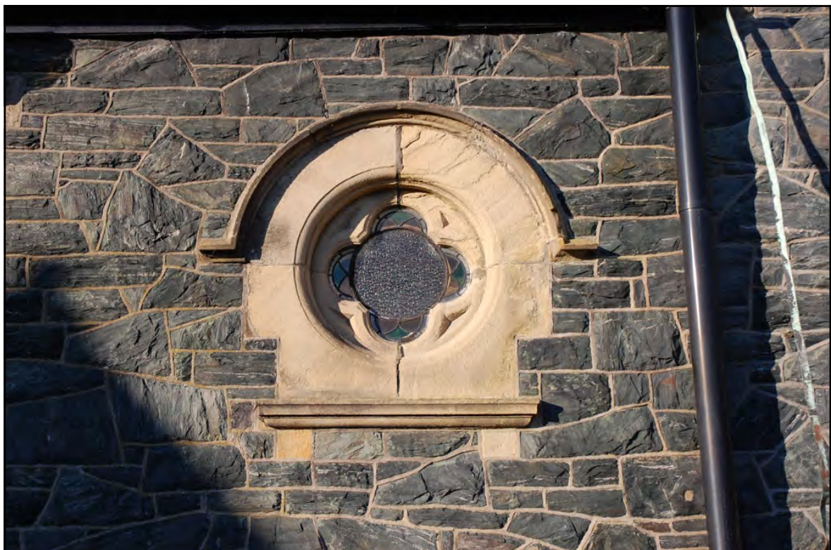
Plate 08: Room G10 External Quatrefoil Light Detail
