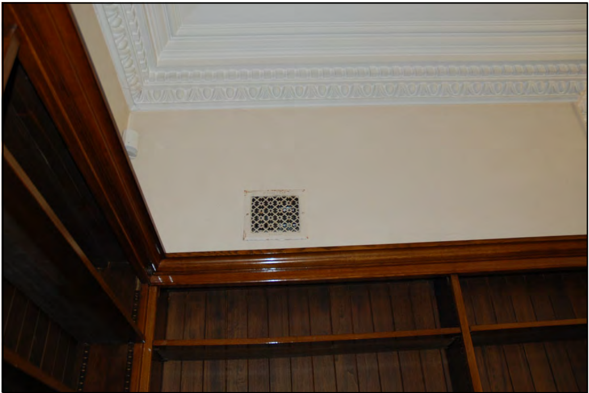
Plate 39: Ground Floor: Room G04: panel detail and wall vent; latter is stamped J. Stott & Co. Oldham
