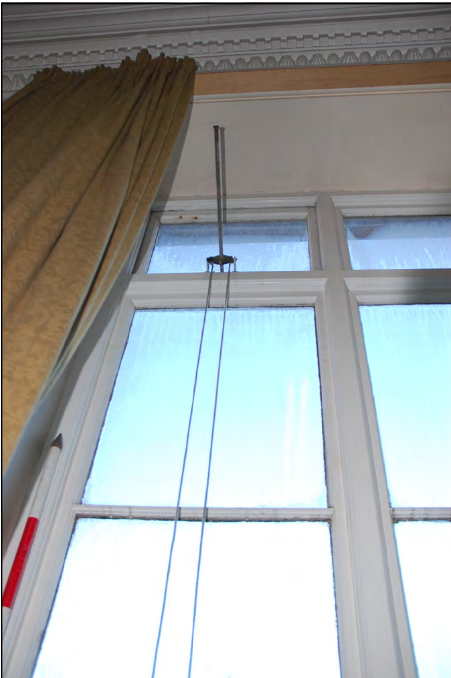
Plate 47: Ground Floor: Room G06: window W07 detail of casement pulley system
