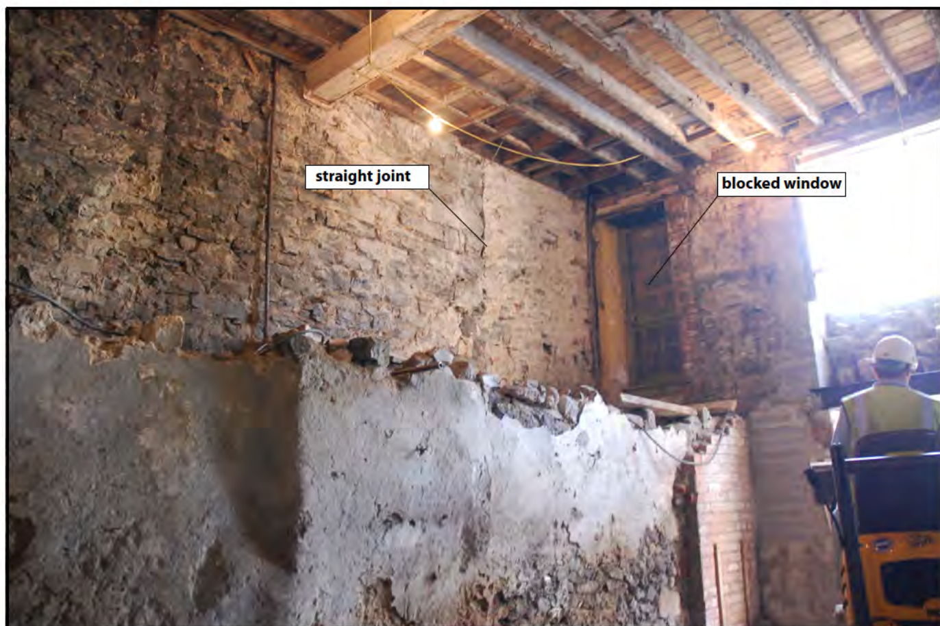
Plate 09: North-facing elevation at Lower Basement Level & Basement level. Note blocked window on basement level and vertical joint in masonry (straight joint)
