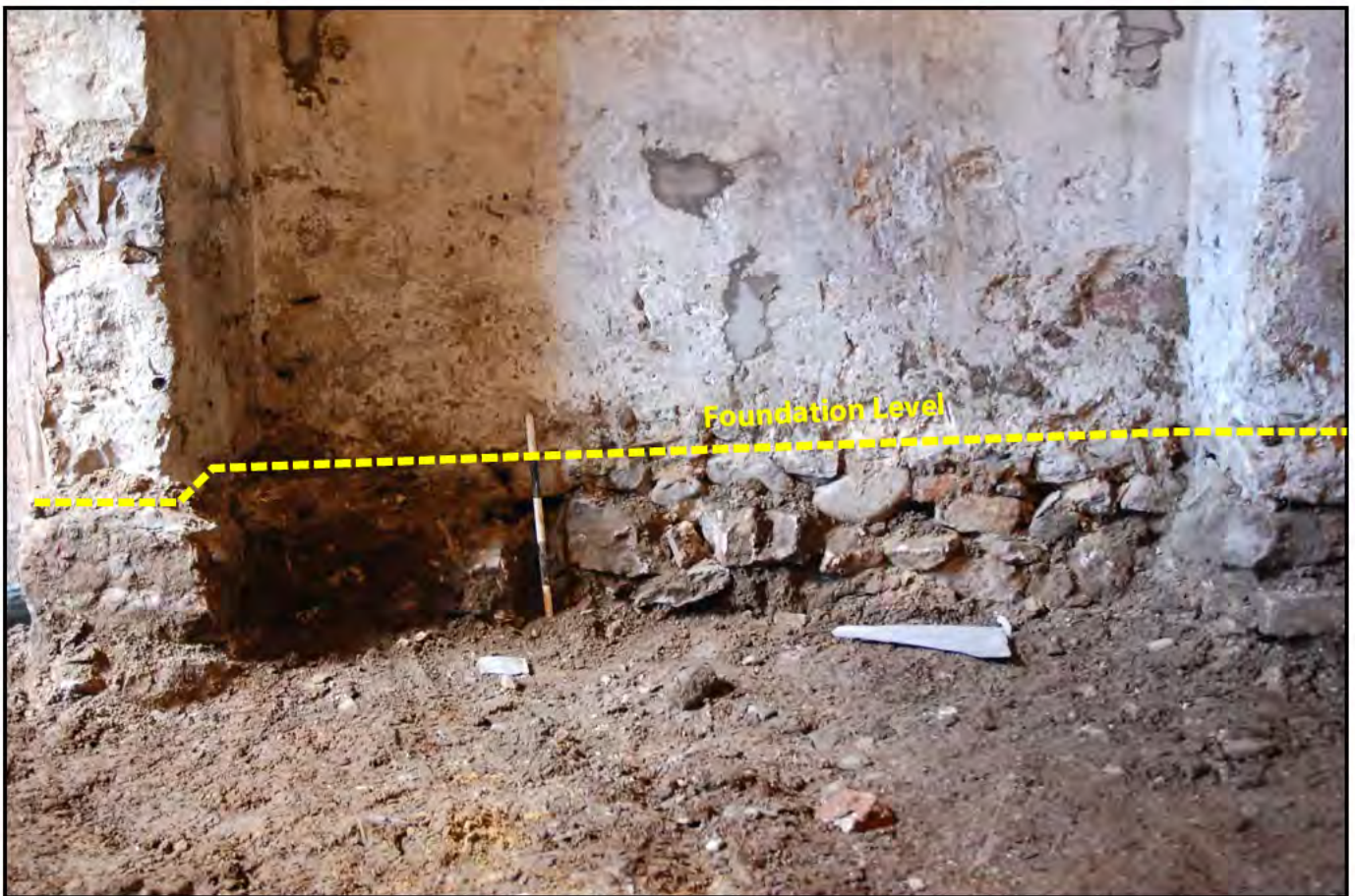
Plate 11: South facing elevation at Lower Basement Level. Final excavation level for groundworks team detailing building technology used. Note use of sandstone blocks at foundation to support buttresses. Similar stones identified along north-facing elevation. In this instance, they appear to have been reused
