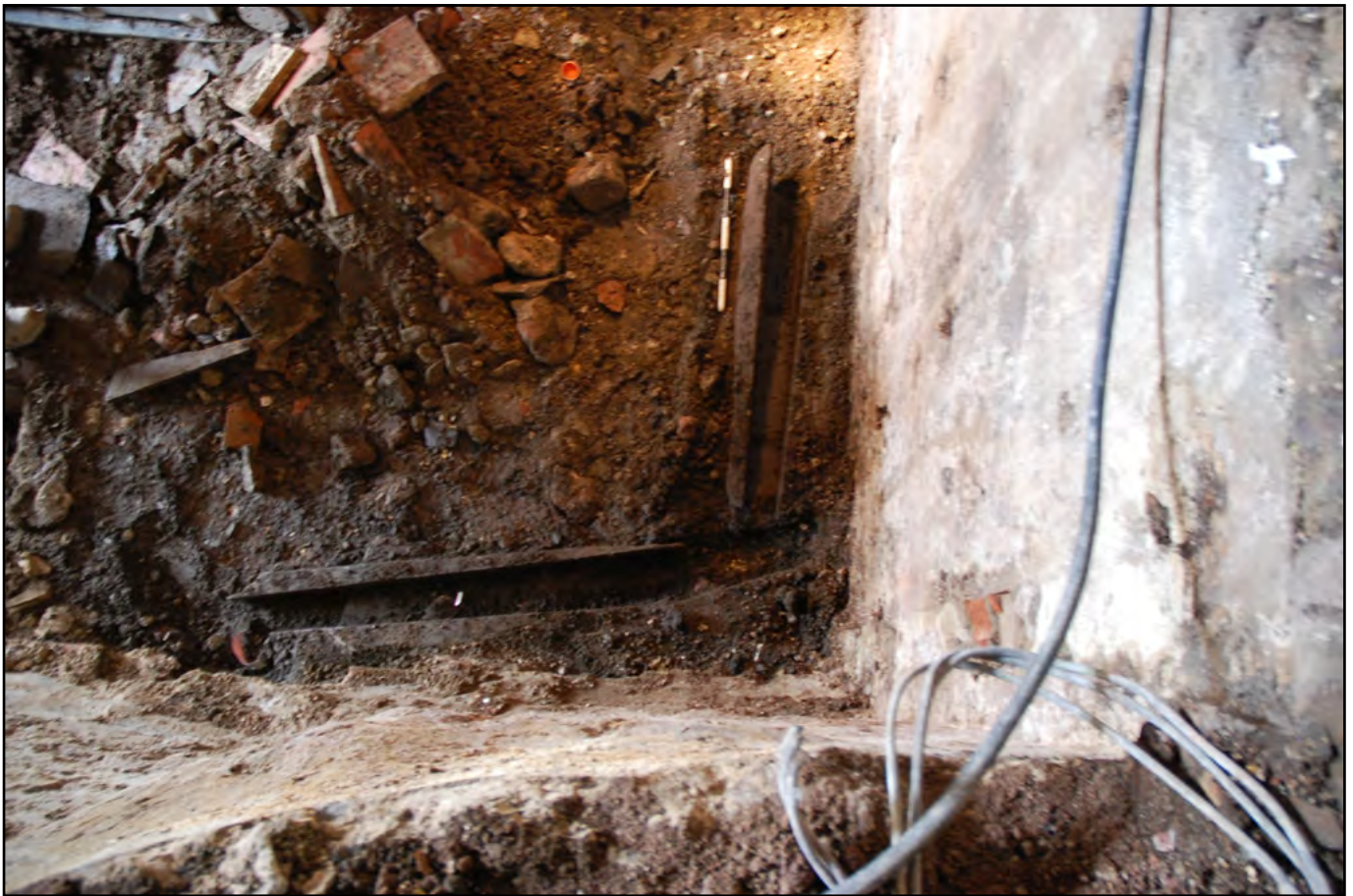
Plate 15: Watching Brief Phase: Slate-lined culvert. The culvert fed into the sump identified in Trench 02 (cf. Plates 02 to 04). The culvert was removed during groundworks, exposing post-medieval levelling material, below which was the suspected medieval structure (Plates 13 and 14; Figures 04 and 05)
