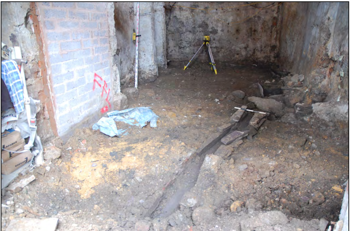
Plate 16: Watching Brief Phase: Slate-lined culvert, which fed from the sump identified in Trench 02 (cf. Plates 02 to 04). The culvert was removed during groundworks. The yellow sand was part of the levelling material for the modern floor surface (removed)
