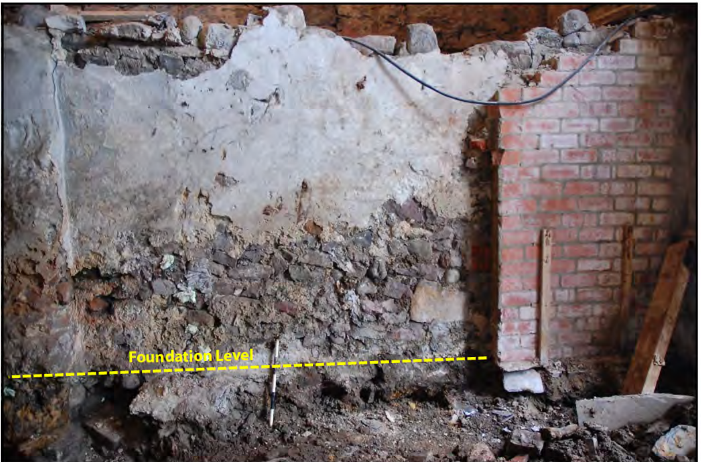
Plate 08: South-facing elevation/west end at Lower Basement Level, detailing construction/foundation level at final excavation level required by groundworks team. Note modern brick wall and original build material where render has been removed. A quarry tile can be seen at bottom left of screen, which could suggest this section of wall was built or repaired during nineteenth/ twentieth century
