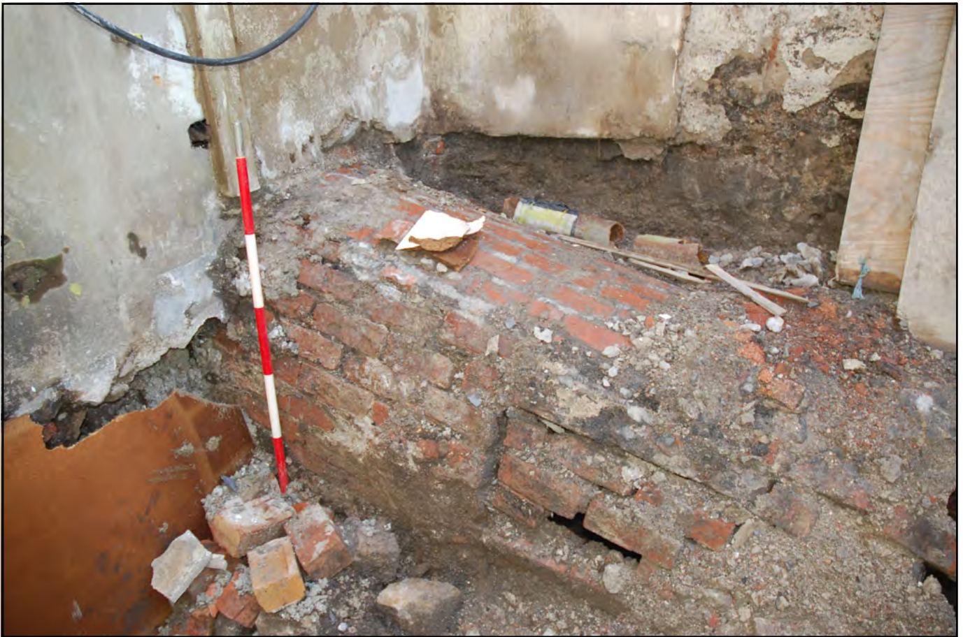
Plate 17: Brick-Built culvert, exposed during work in the rear "courtyard".
