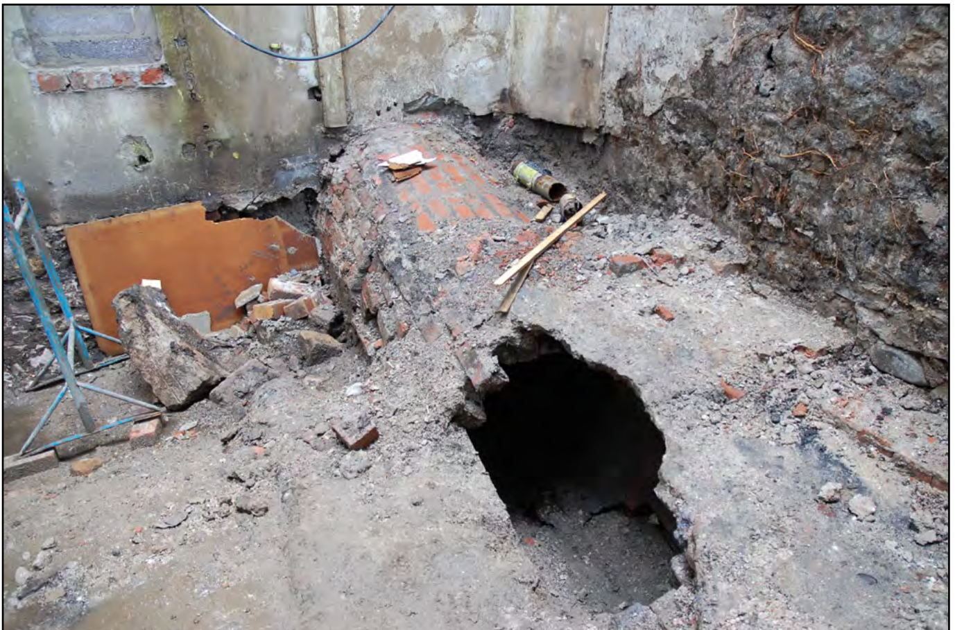
Plate 18: Brick-Built culvert, exposed during work in the rear "courtyard" during subsequent breach
