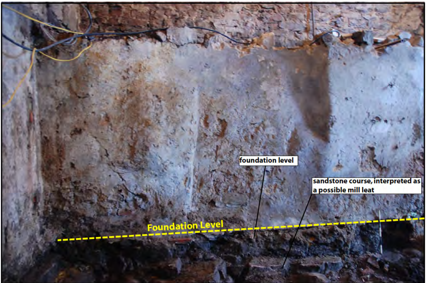
Plate 07: North-facing elevation/east end at Lower Basement Level, detailing construction/foundation level (including a separate sandstone course).
