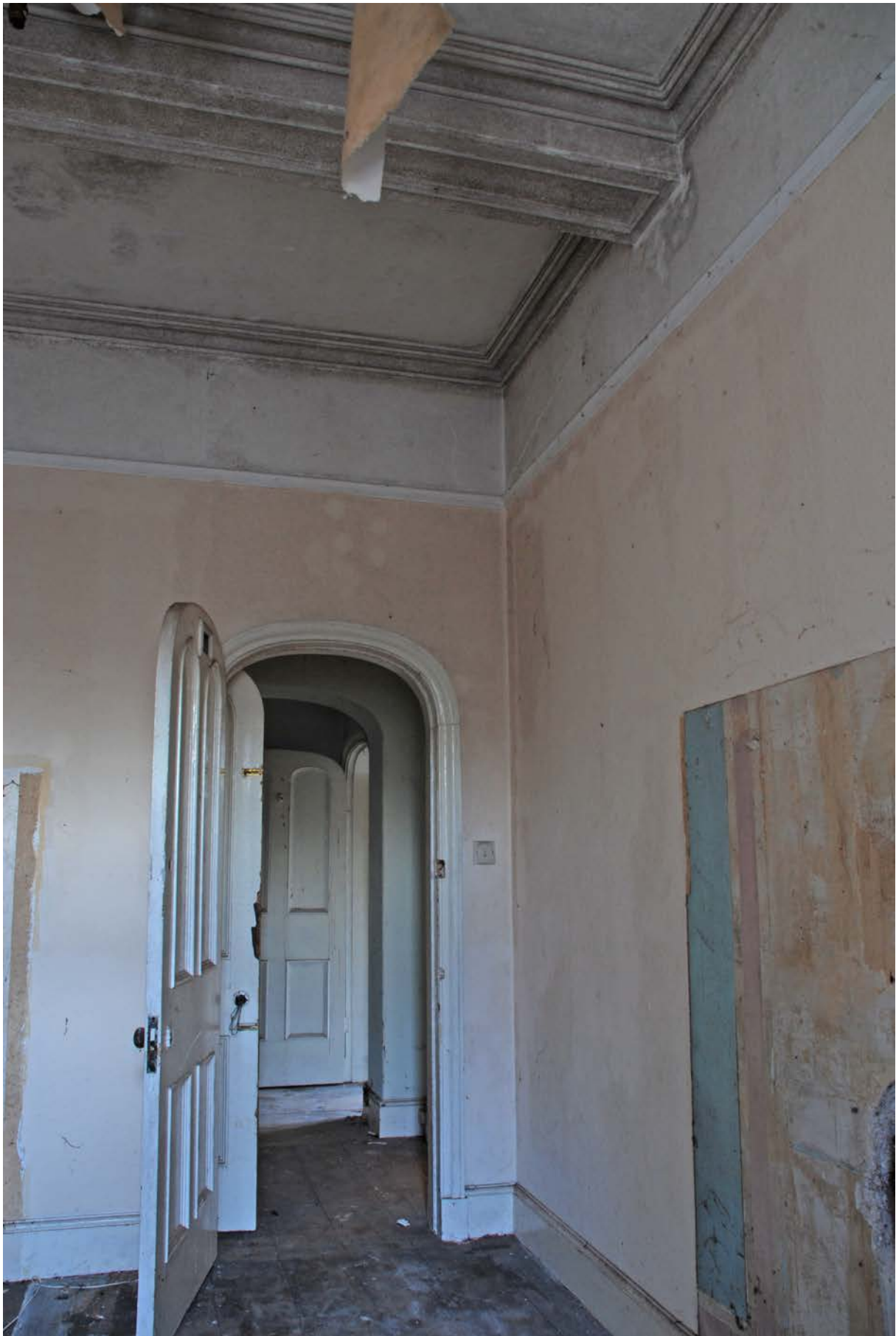
The room above the early Victorian dining room with lath and plaster partition scheduled for removal
