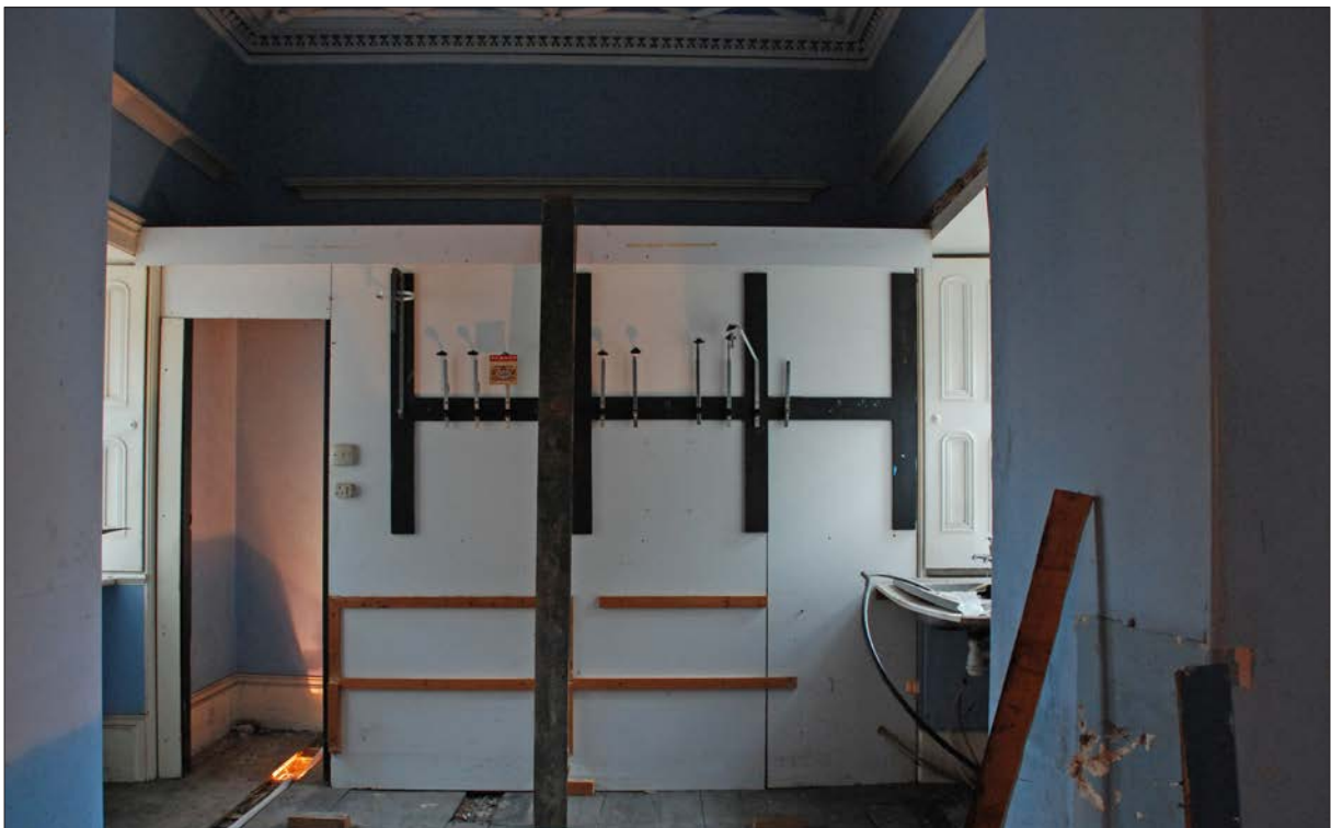
The first floor above the porch and the stud partition scheduled for demolition
