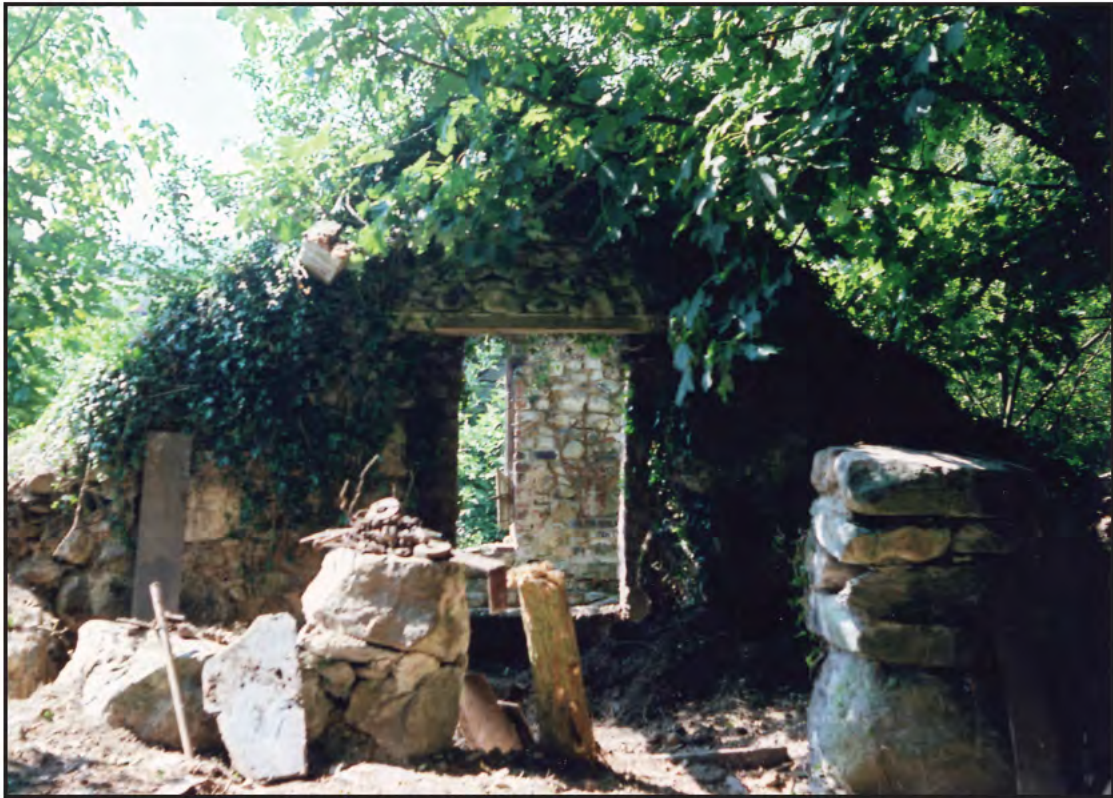
Plate 1. South facing image of the north gable prior to collapse.
