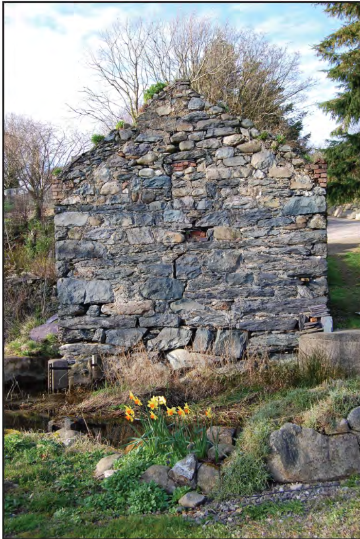
Plate 9. North facing image of south gable.
