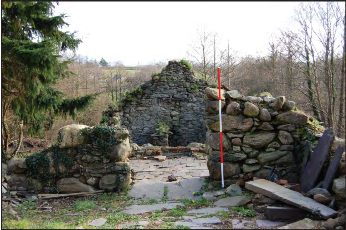
Plate 3. South facing image of the north gable.
