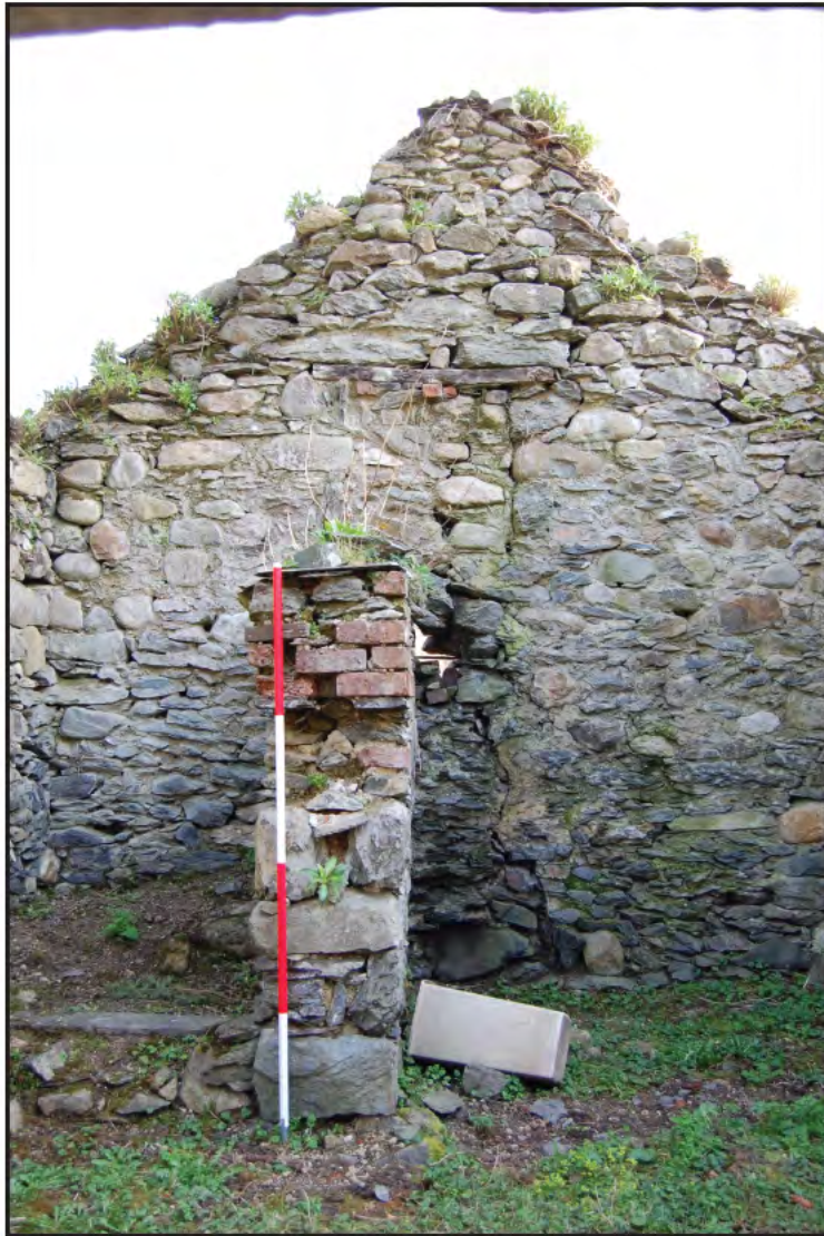
Plate 7. South facing image of internal of the south gable showing the dividing wall.
