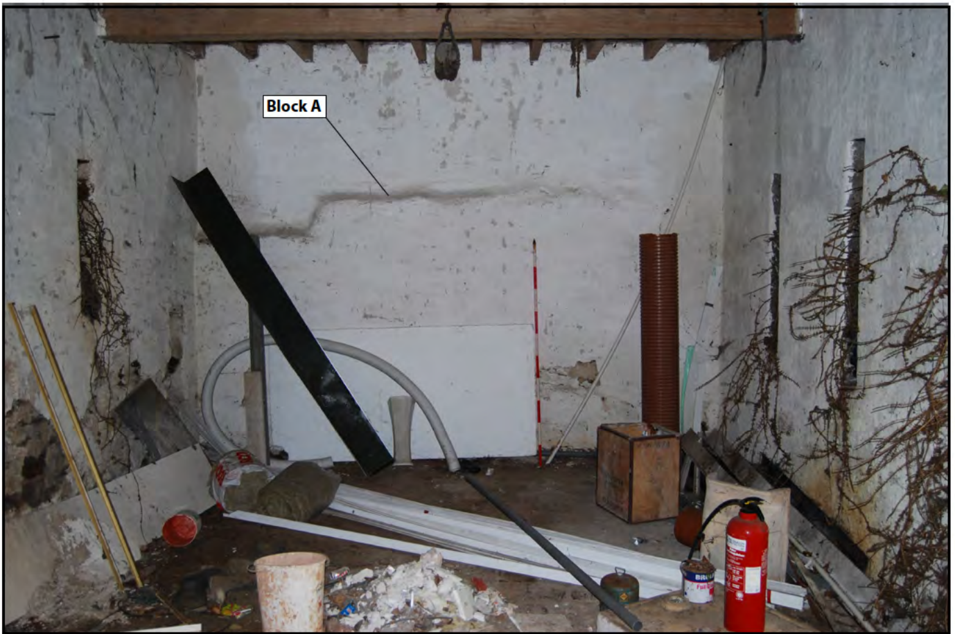
Plate 17: Southwest facing internal elevation of Block B (Ground Floor). Note line defining where Block A and Block B are attached
