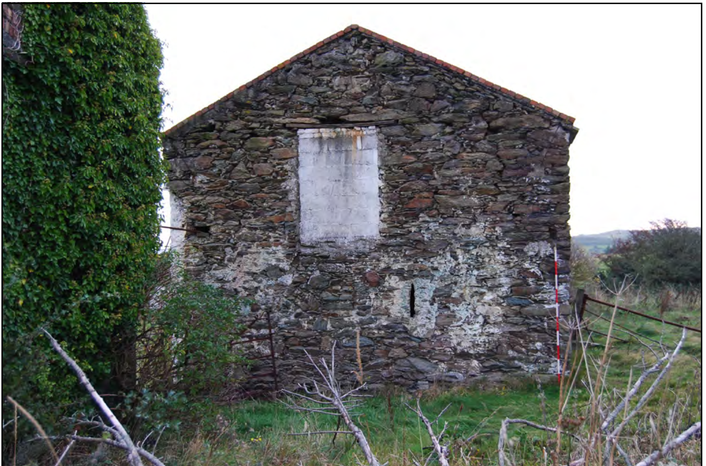
Plate 22: Northwest facing elevation of Block C. Note blocked window
