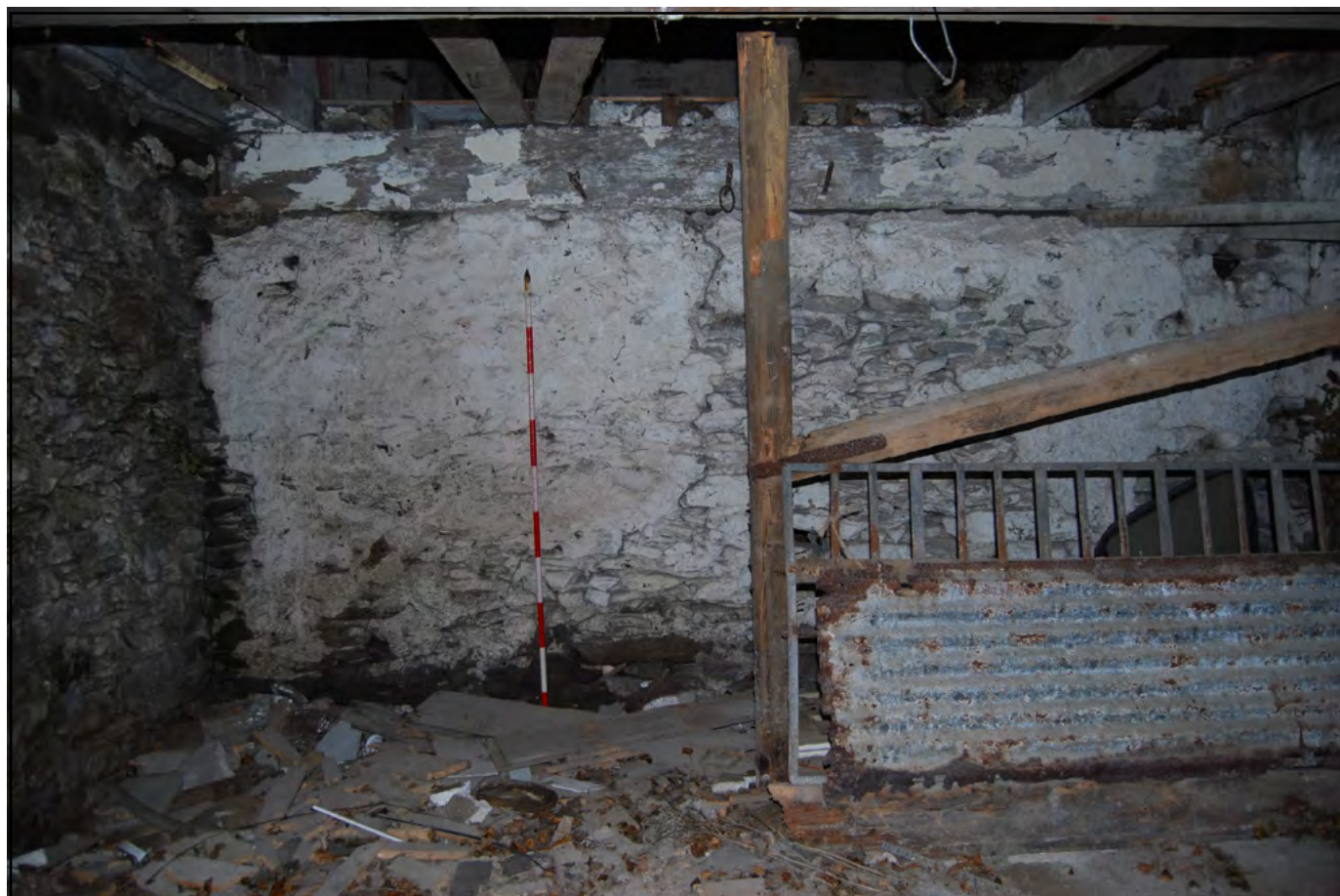
Plate 29: Southwest facing internal elevation of Block D room (First floor). Note stockade constructed from timber and corrugated iron
