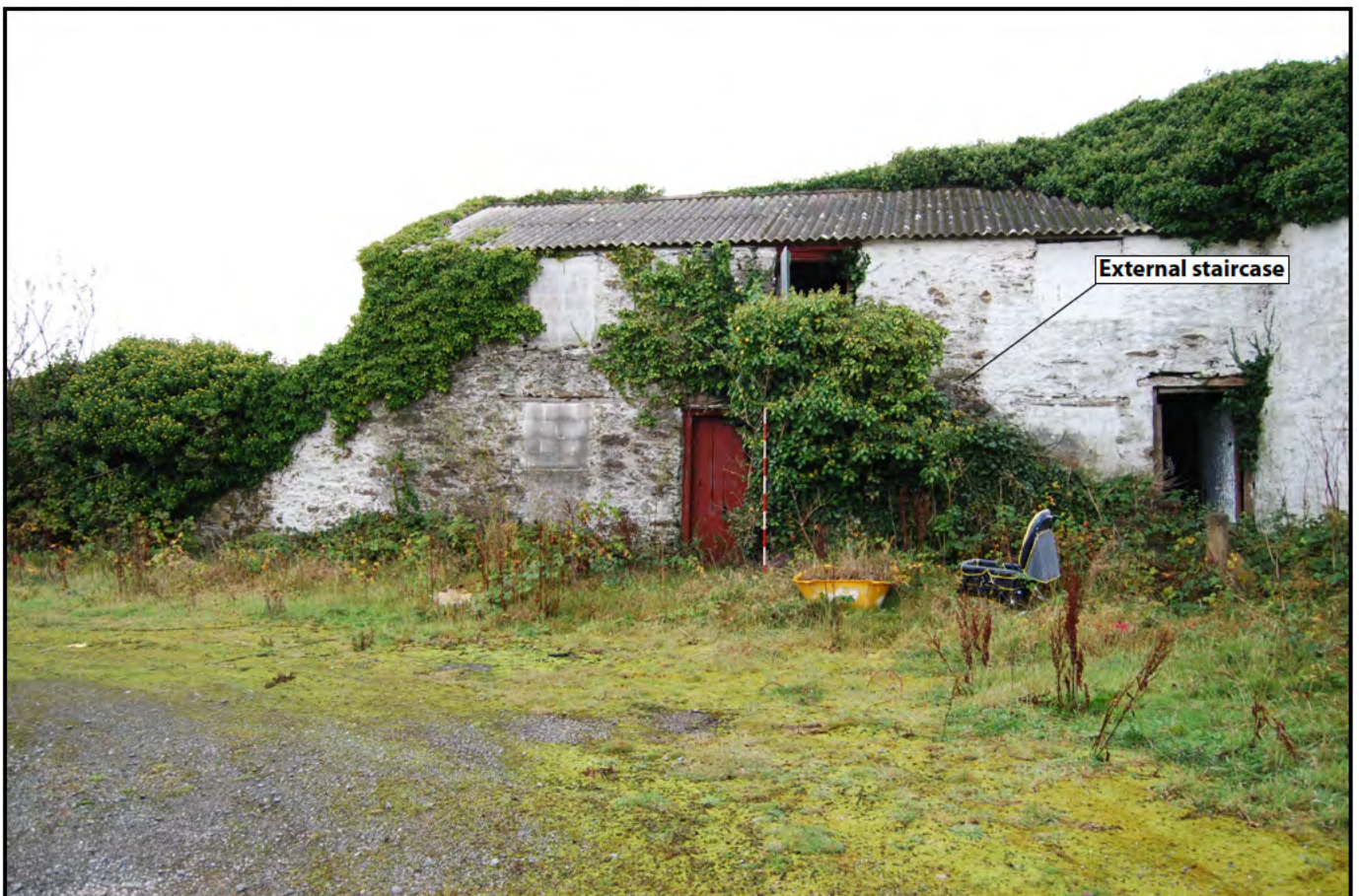
Plate 26: Northwest facing elevation of Block D. Note modern roof, external staircase and blocked windows
