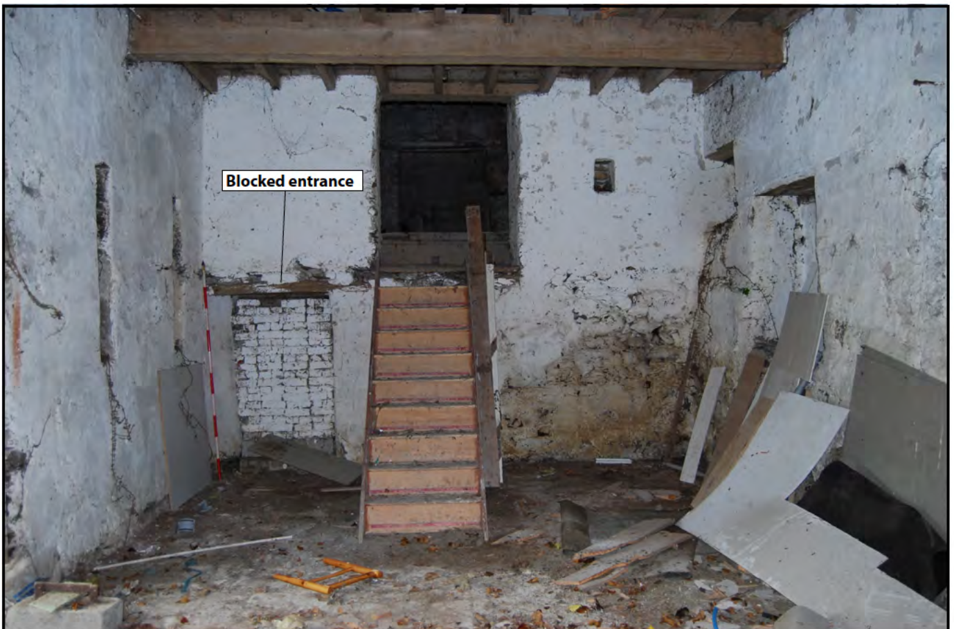
Plate 18: Northeast facing internal elevation of Block B detailing modern stairs leading to first floor. Note blocked entrance leading to adjacent ground floor room
