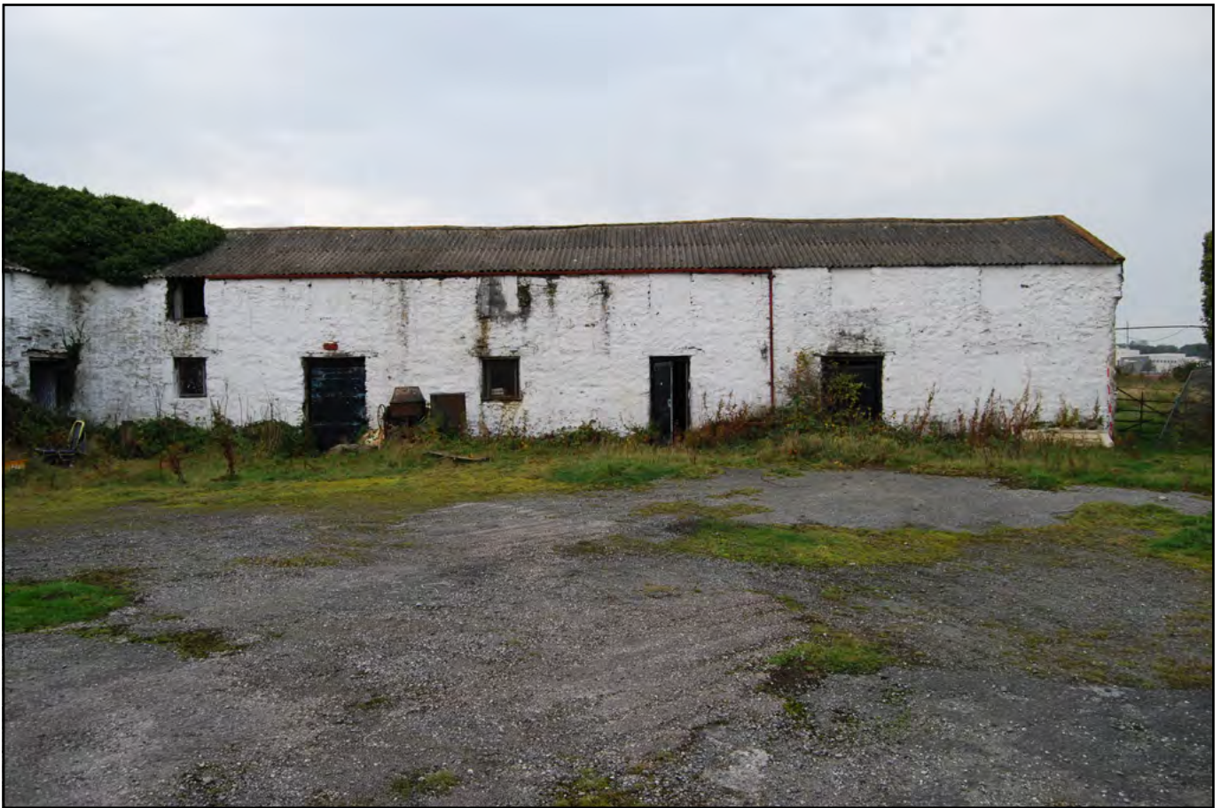
Plate 21: Northeast facing elevation of Block C. Note modern corrugated roof, blocked windows and modern entrances
