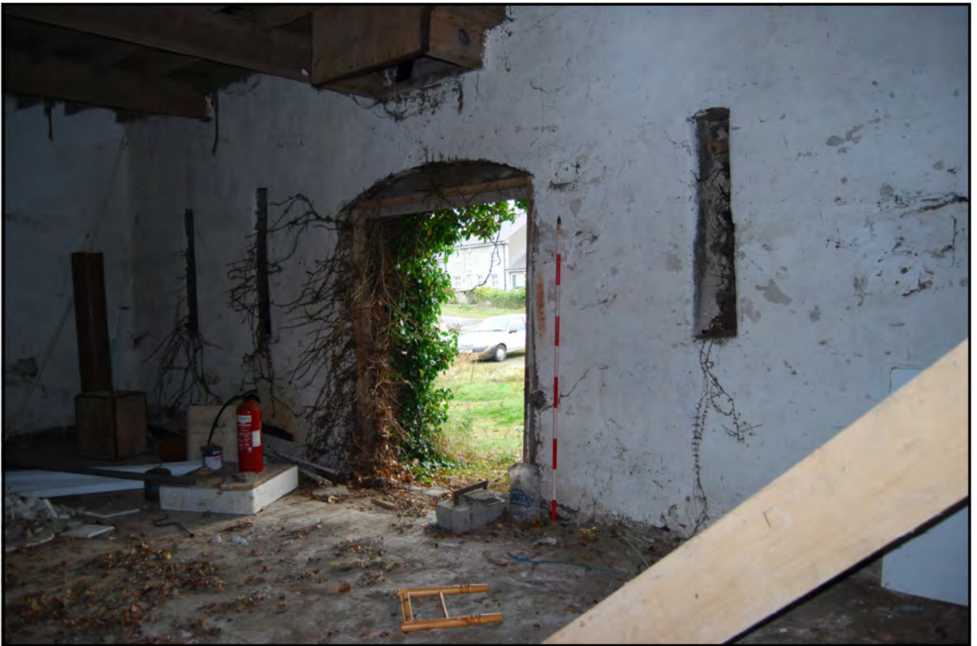
Plate 15: Block B Northwest facing Internal elevation. Note remodelled archway entrance.
