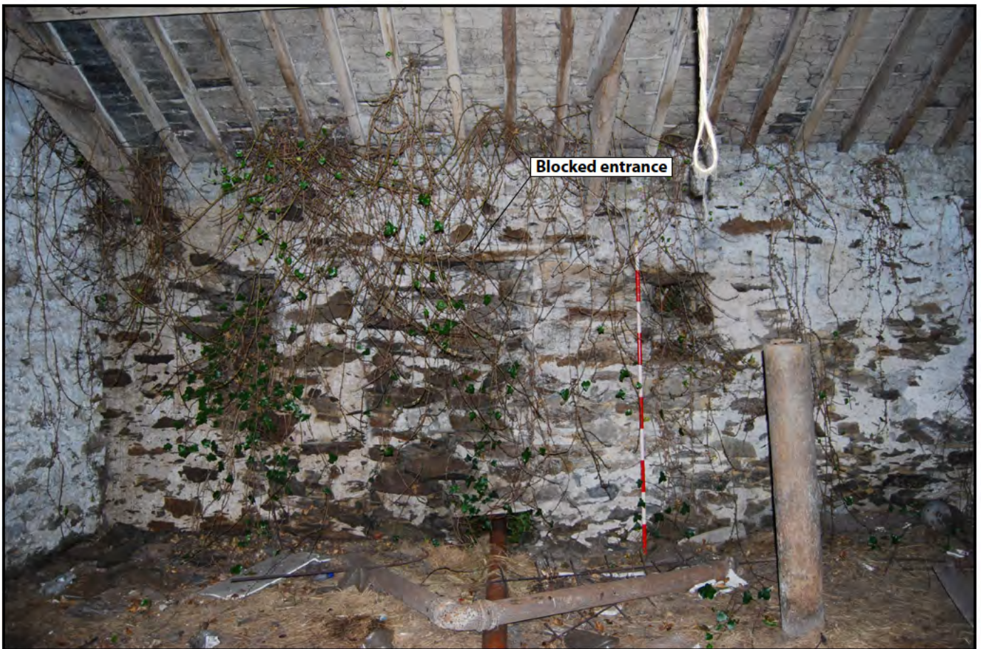
Plate 5: Southeast facing internal elevation of Block A building: detailing wall and roof construction and current use. Note the blocked entrance and apertures either side.
