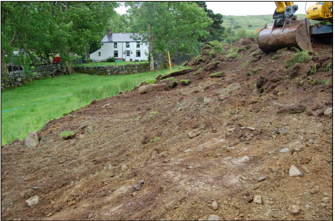
Plate 03: View East of Powerhouse Location during works. Shale-rich Subsoil exposed.
