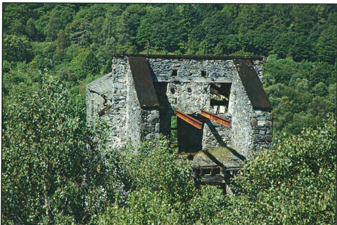
Plate 6: CN156: Turbine House/Stone Breaker Room and Aerial Ropeway Link
