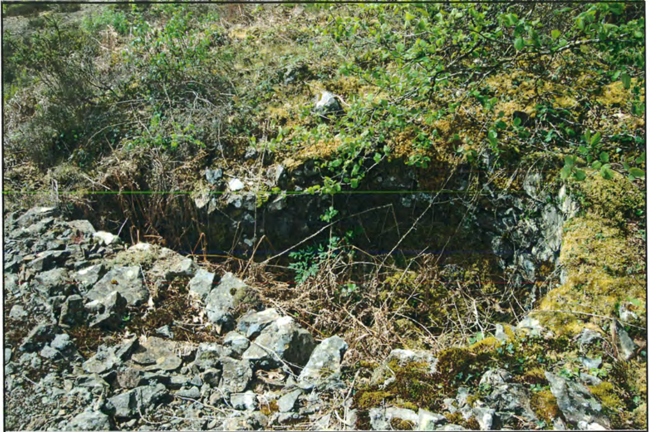
Plate 7: CN332: Capstan Pit
