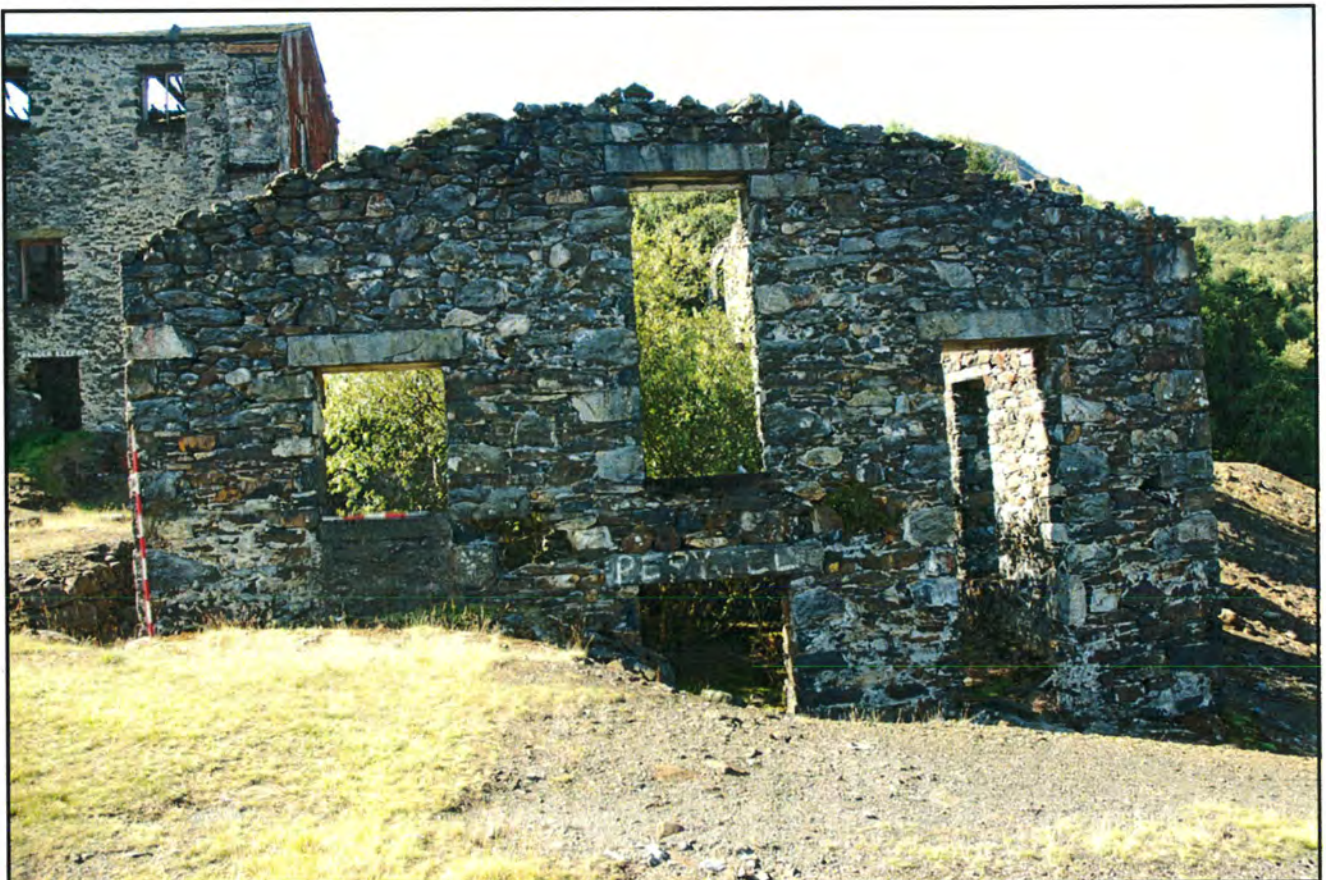
Plate 4: CN156: North Facing Elevation of Former Jig House
