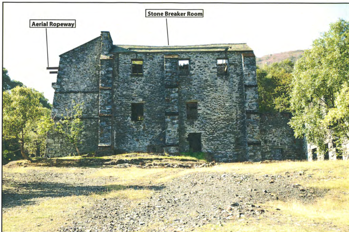
Plate 1: CN156: North Facing Elevation Turbine House/Stone Breaker Room and Aerial Ropeway
