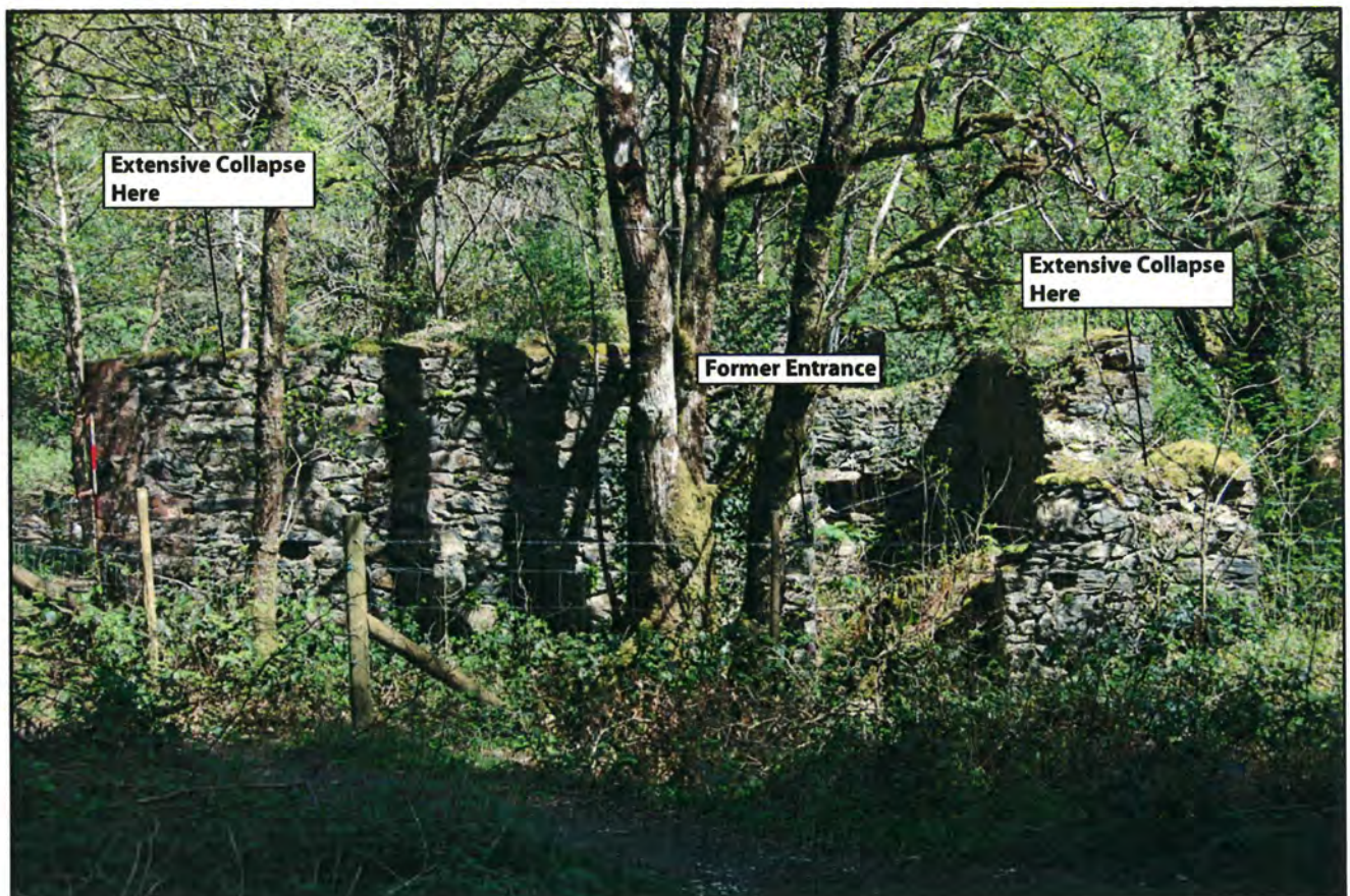
Plate 4: CN331: Southwest Facing Elevation of Mill Building
