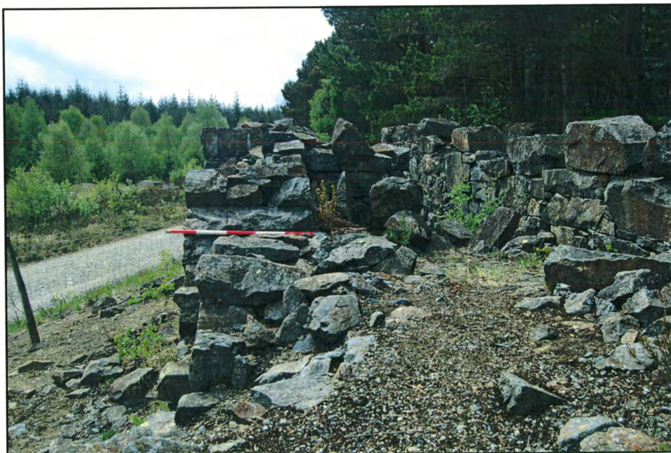
Plate 16: CN332: Wheel Pit No. 1: Detail of Ruined East Facing Elevation
