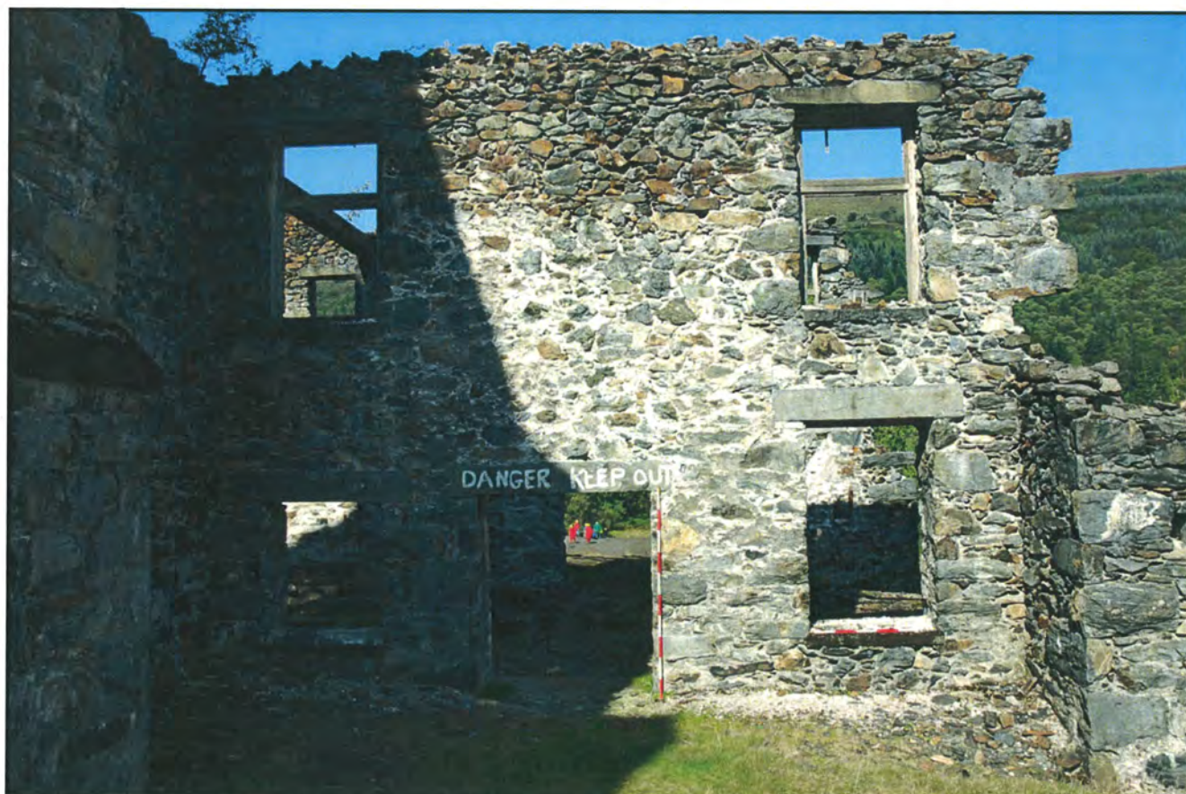
Plate 2: CN156f: Wheel Pit No. 1: Detail of Ruined East Facing Elevation
