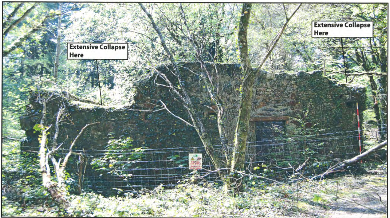
Plate 1: CN331: Northeast Facing Elevation of Mill Building
