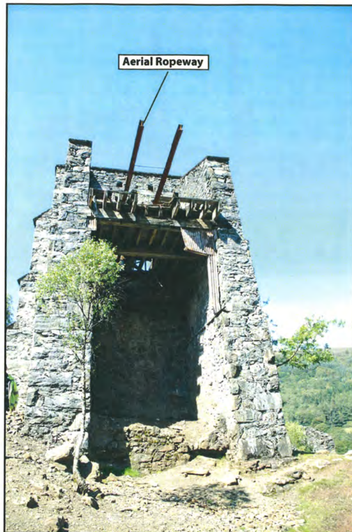
Plate 5: CN156: Detail of Aerial Ropeway into Stonebreaker Room
