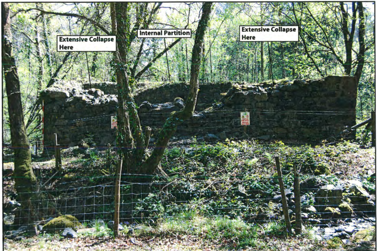
Plate 3: CN331: West Facing Elevation of Mill Building
