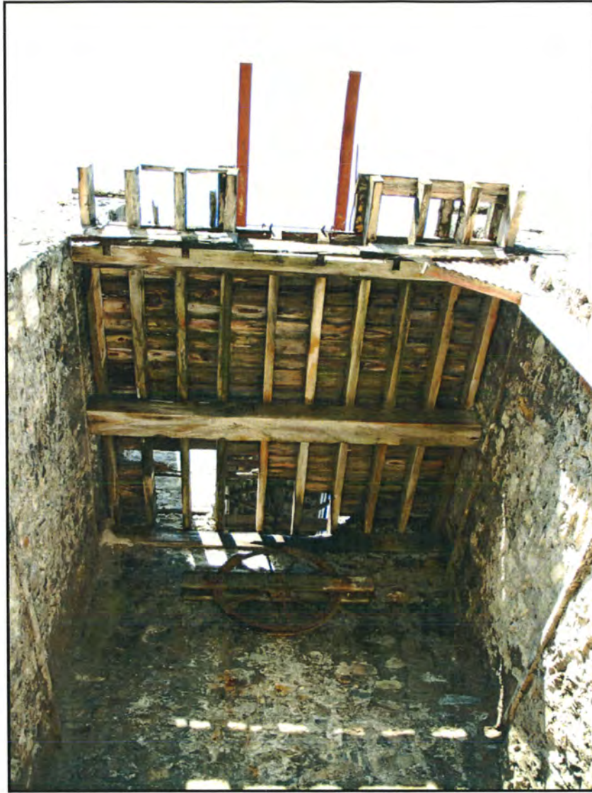
Plate 7: CN156: Detail of Aerial Ropeway
