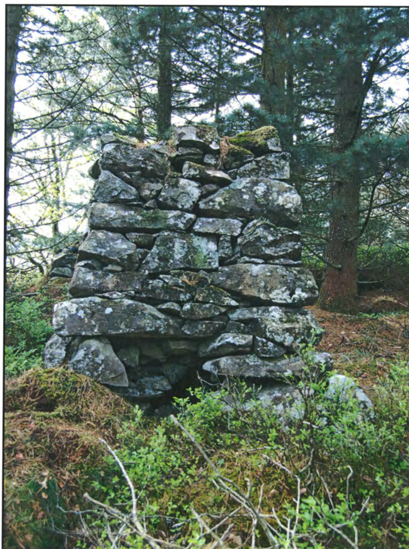
Plate 2: CN332: Aqueduct Platform (View South)
