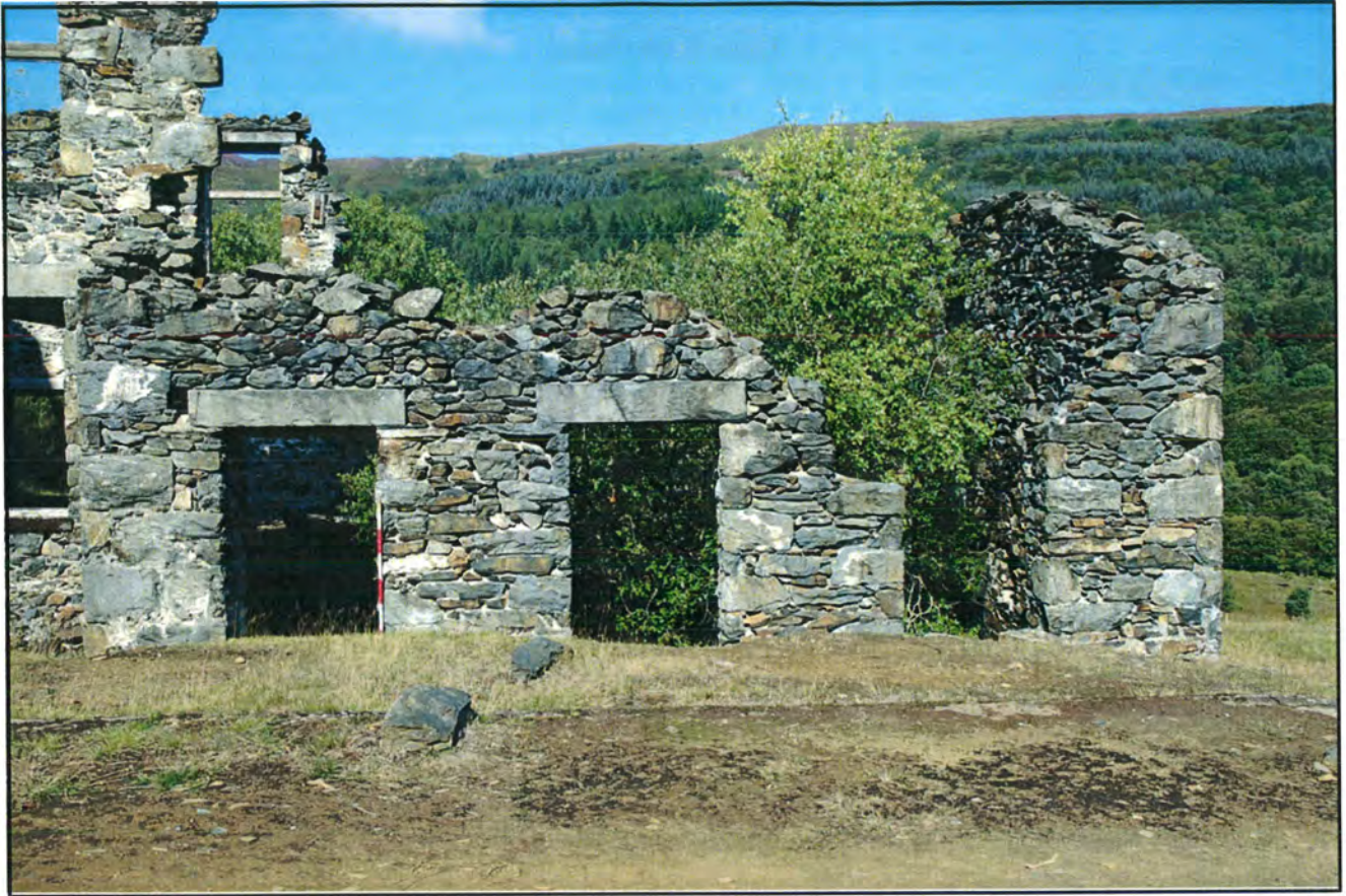
Plate 3: CN156: East Facing Elevation of Former Jig House
