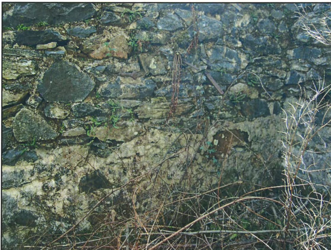
Plate 6: CN331: Internal Partition: Detail of Limewash and Fittings
