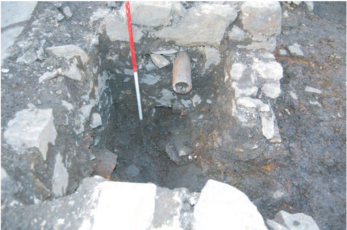
Fig. 21. The privy cess pit chamber from the west with the pit emptied, showing the original rear drain hole and the inserted pipes of the later toilet at a higher level. Scale with 50cm divisions.
