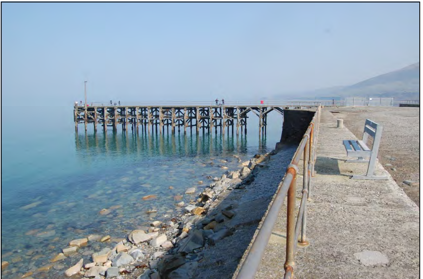
Plate 4: Trefor: View East of Nineteenth Century Wooden Pier (PRN25013)
