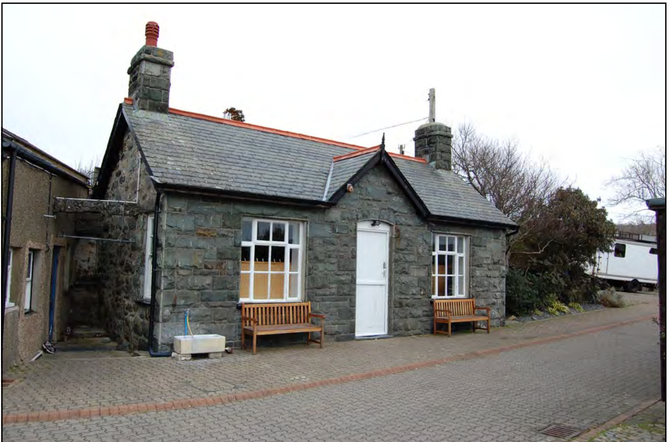
Plate 4: Pensarn: nineteenth Century Wharf Office (PRN25055)
