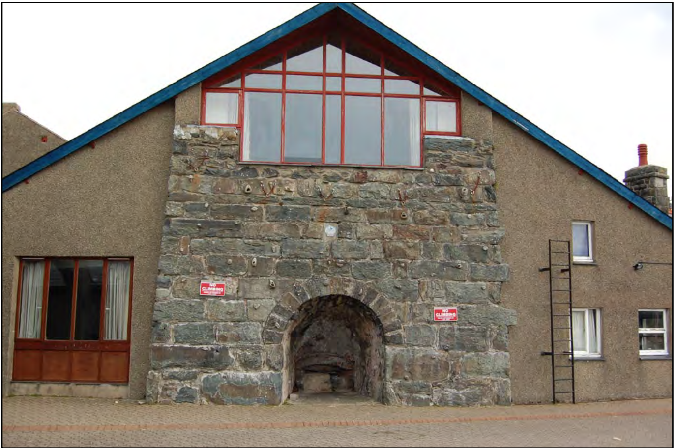
Plate 3: Pensarn: Former Limekiln incorporated into a Late twentieth Century Building (PRN25050)
