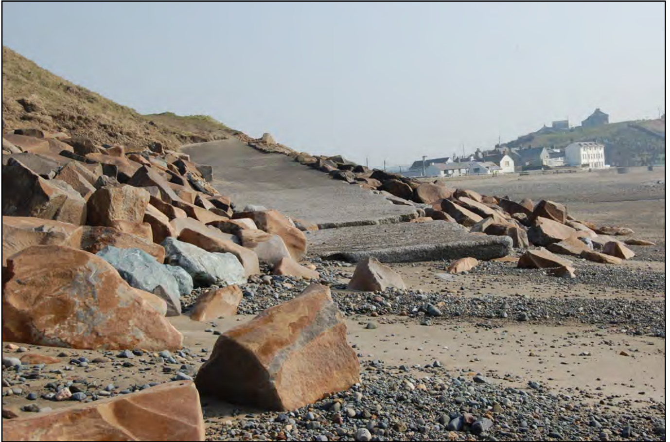
Plate 11: Aberdaron: View East of Concrete Slipway (PRN 25005). Note State of Disrepair Suggesting Lack of Use.
