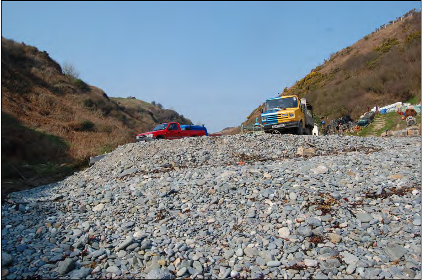
Plate 19: Raised Parking Area Created from Beach Stone.
