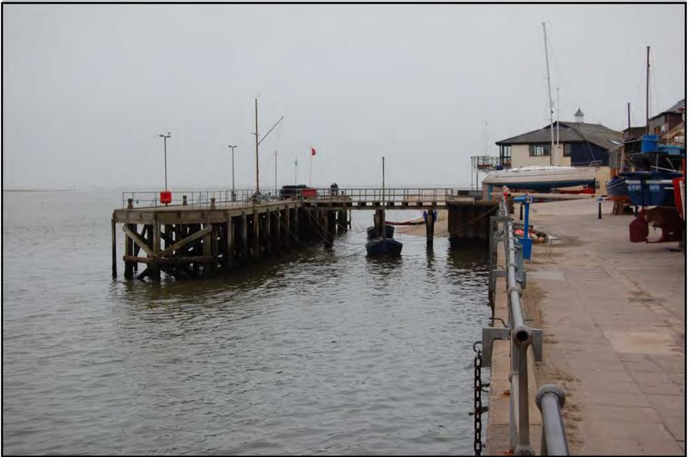
Plate 1: Aberdyfi: View of Pier
