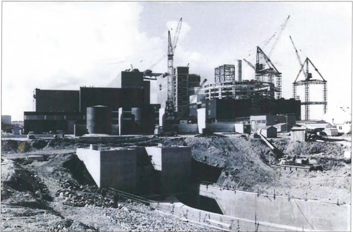
Photograph 1: Wylfa under construction: showing the outflow and the reactors and turbine hall
