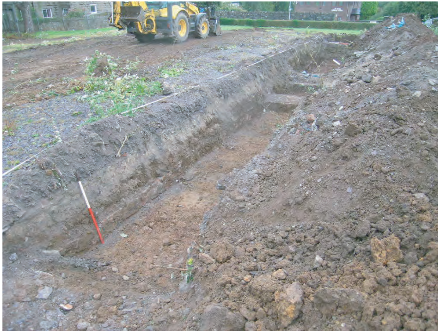
Sir Hugh Owen Lower School Development Fig. 8 Trench 3, General view from south-east excavated to the subsoil surface, showing in section the buried 19th century ploughsoil, school construction made-ground and demolition debris. Scale with 0.50m divisions
