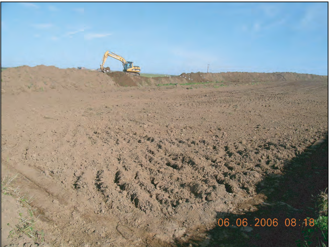
Plate 2: Phase I Area: Stripping of area during Site Compound construction
