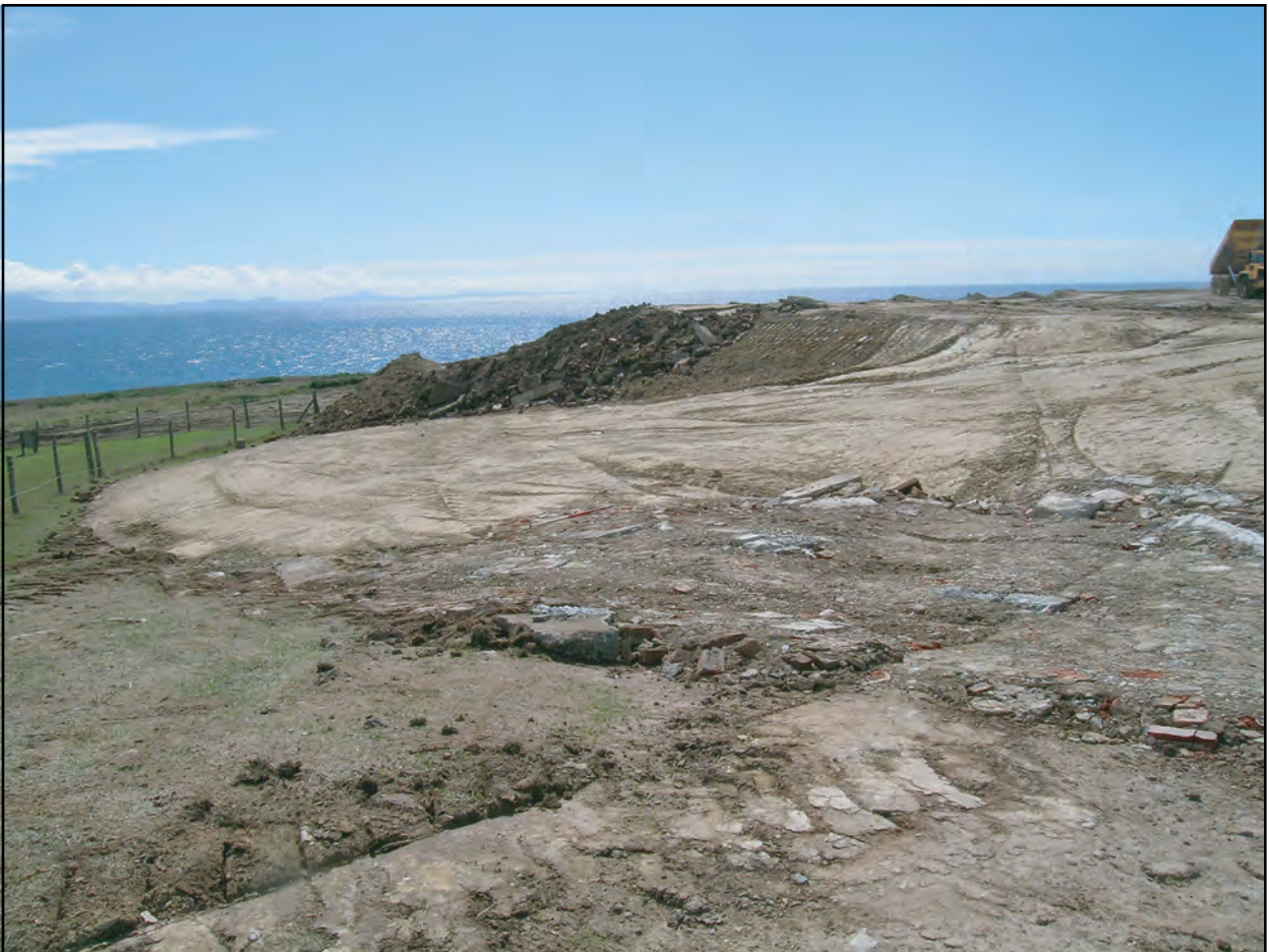
Plate 10: Phase II Area: Construction of Landscaping Bund
