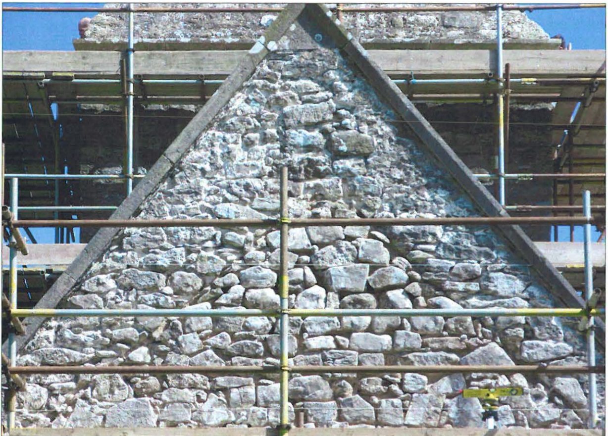
Nave, west gable, showing lower roof line
