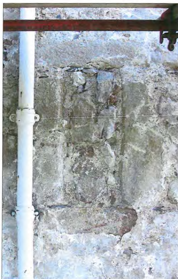
Early window at first floor level, south of the south stack
