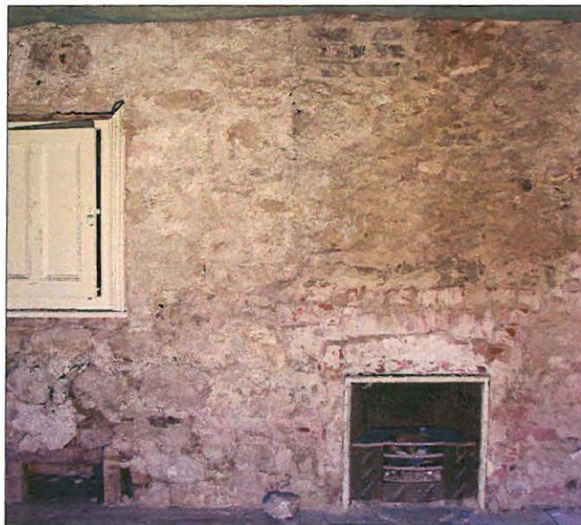
First floor south fireplace, plaster stripped
