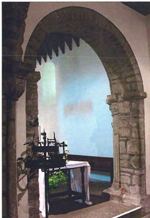
Plain back of arch from tower to nave, showing rebate for screen in impost
