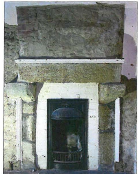
Second floor south fireplace, plaster stripped
