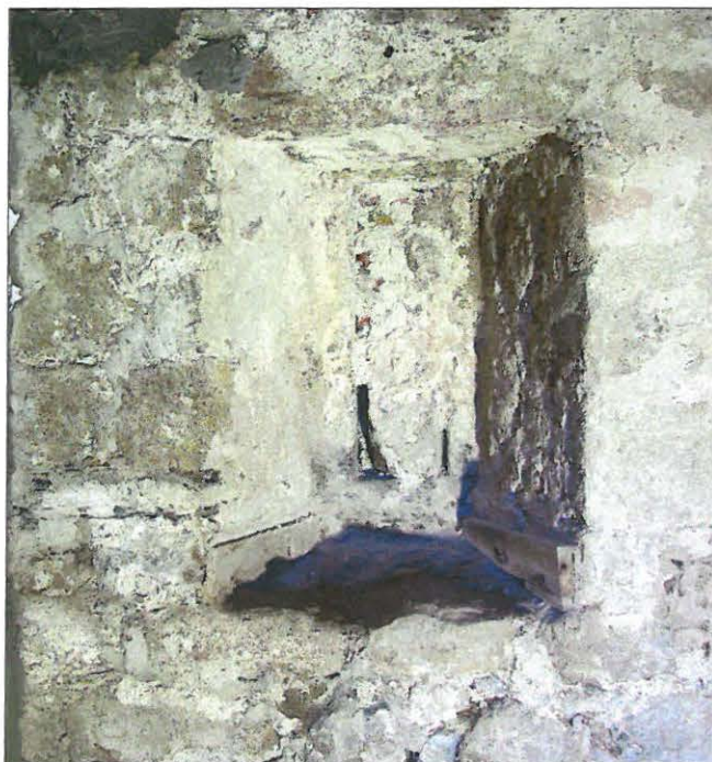
First floor south, early window revealed behind cupboard
