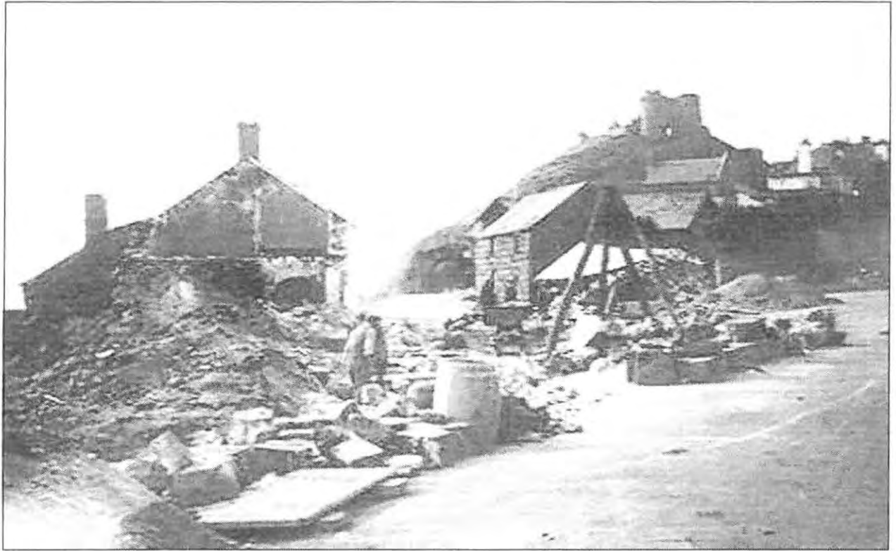
Figure 9. Abermarchnad following the storm of 1927. (Gwynedd Archives).
