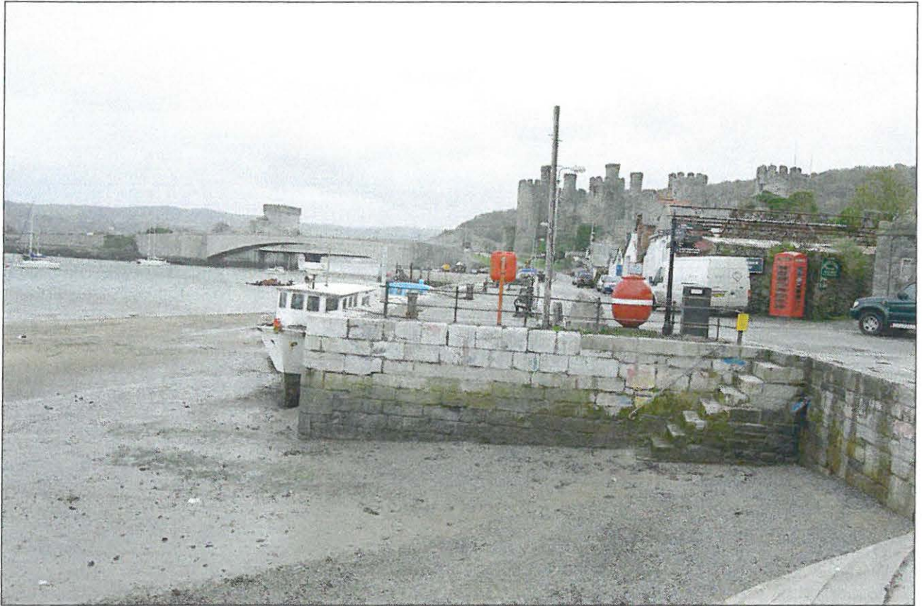
Figure 13. The quay built in 1833 (PRN 19750)
