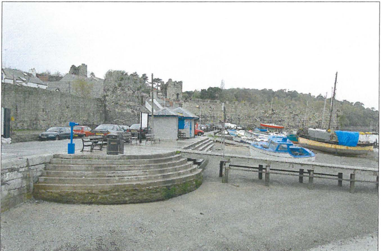
Figure 14. General view of Lower Gate Street and the 1965 jetty (PRN 19769)
