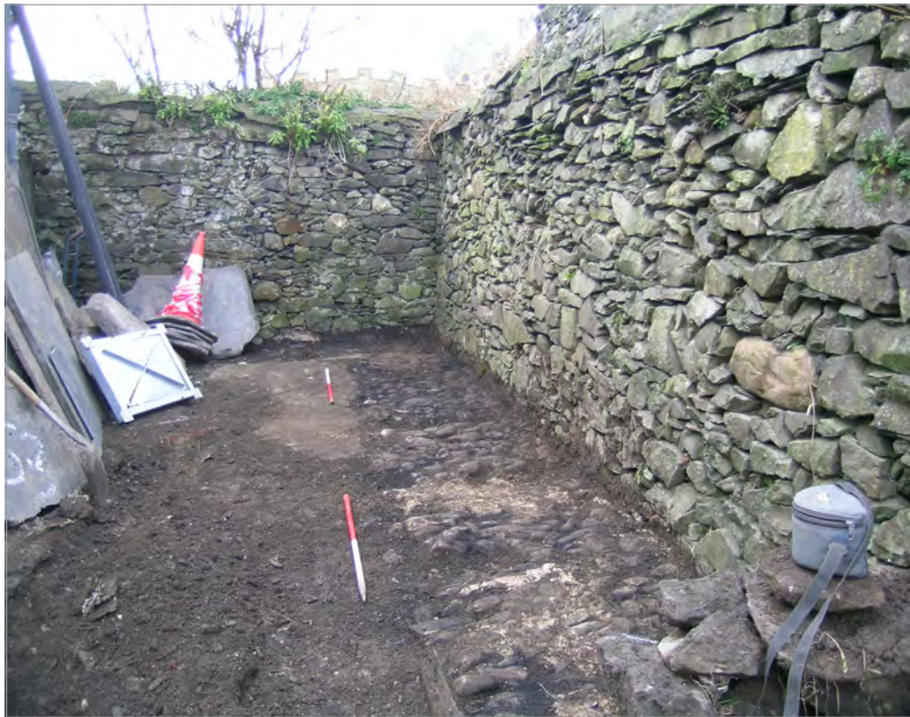
Plate 7: View West of Former Coal Shed Area with Surviving Cobbled Floor. (Note: Coal Dust on the Cobbles and Redundant Roof Slates Embedded at the Top of the Boundary Wall)
