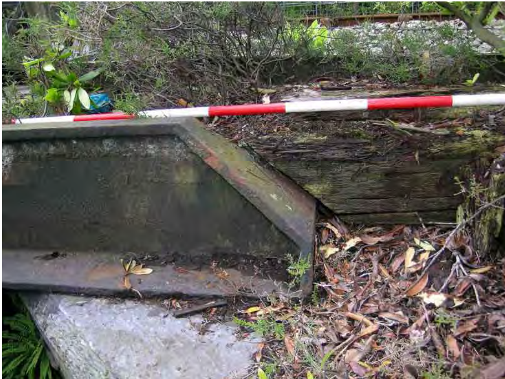
Plate 19 Bridge 67, girder end fitted to baulk
