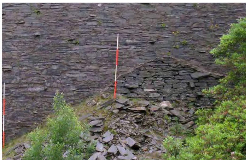
Plate 32 Masonry styles; earlier drystone masonry exposed by erosion
