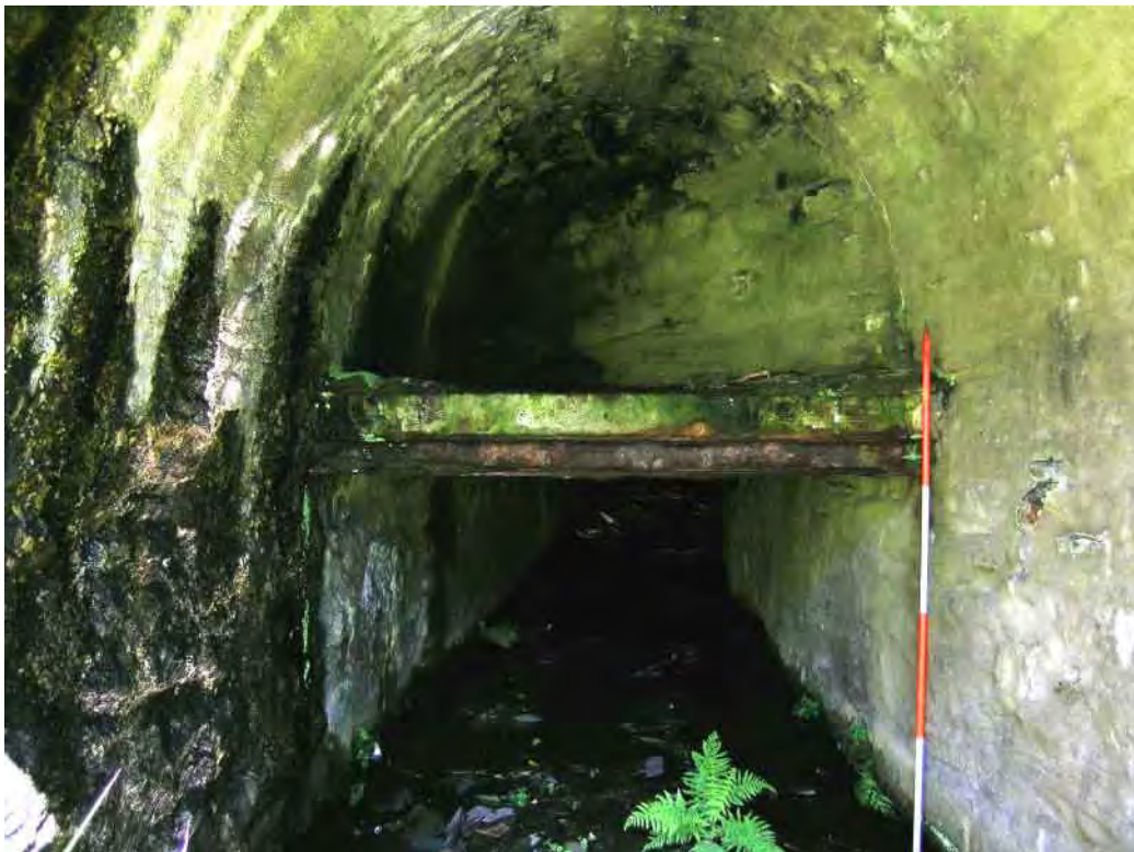
Plate 34 Incline tunnel, W side, partial blocking within tunnel
