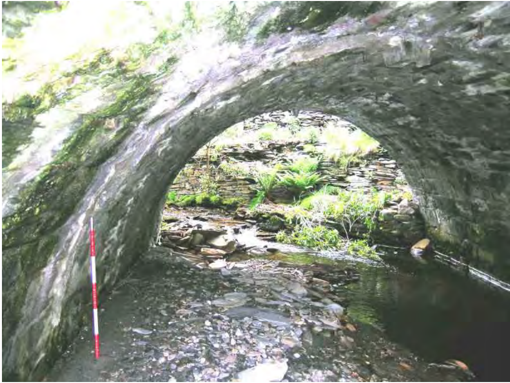
Plate 37 Afon Barlwyd tunnel, two phases of masonry within roof
