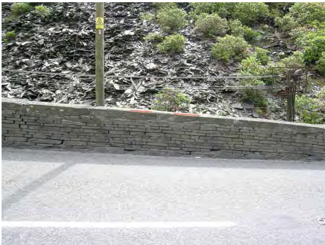
Plate 31 Masonry styles; roadside parapet, dry laid slate
