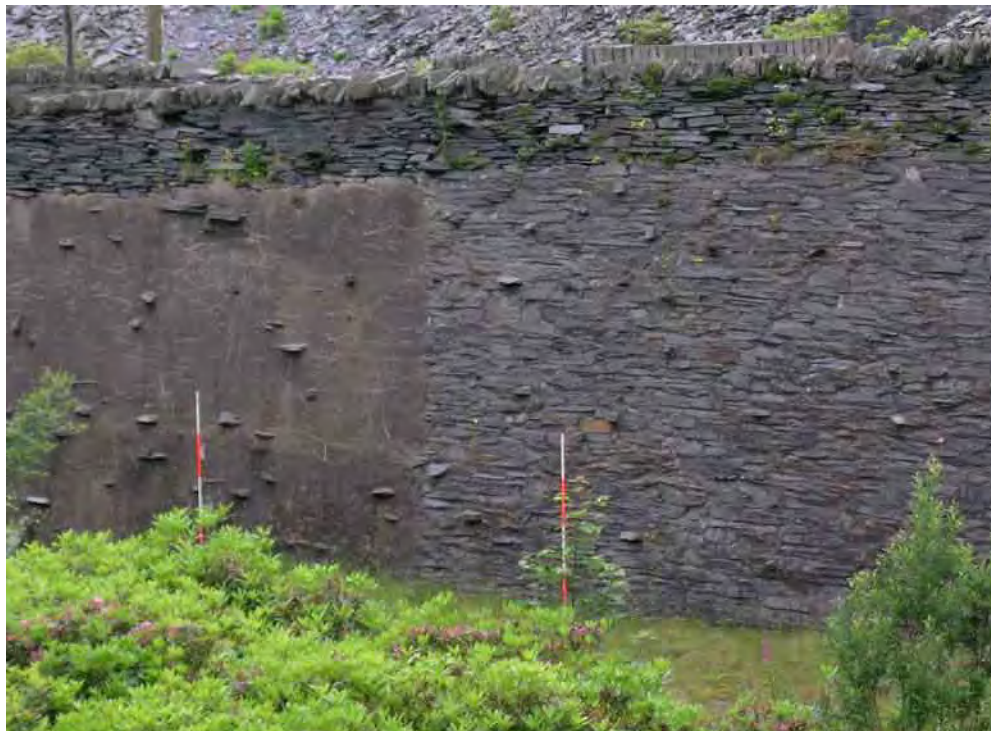
Plate 30 Masonry styles; slate with spray concrete render and pointing
