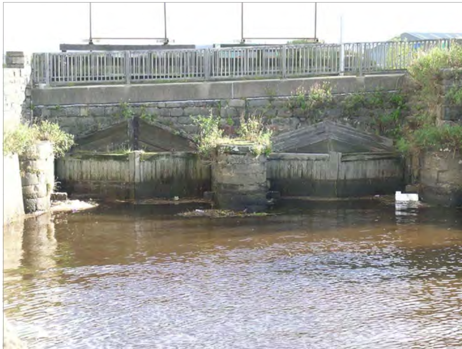
Plate 1: Tidal Gates A and B Closed
