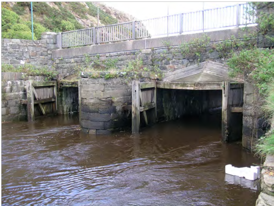
Plate 2: Tidal Gates A and B Open (Tidal Gate B In Foreground)
