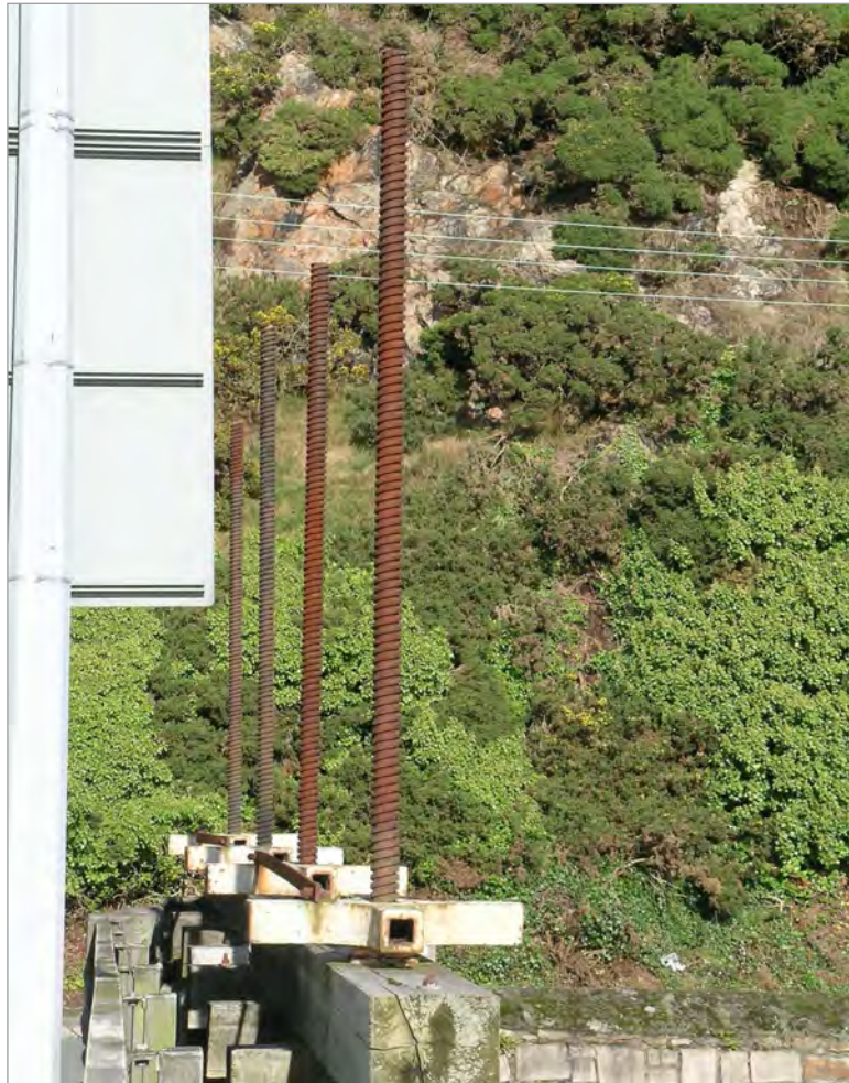
Plate 14: Detail of Penstock Winding Mechanism
