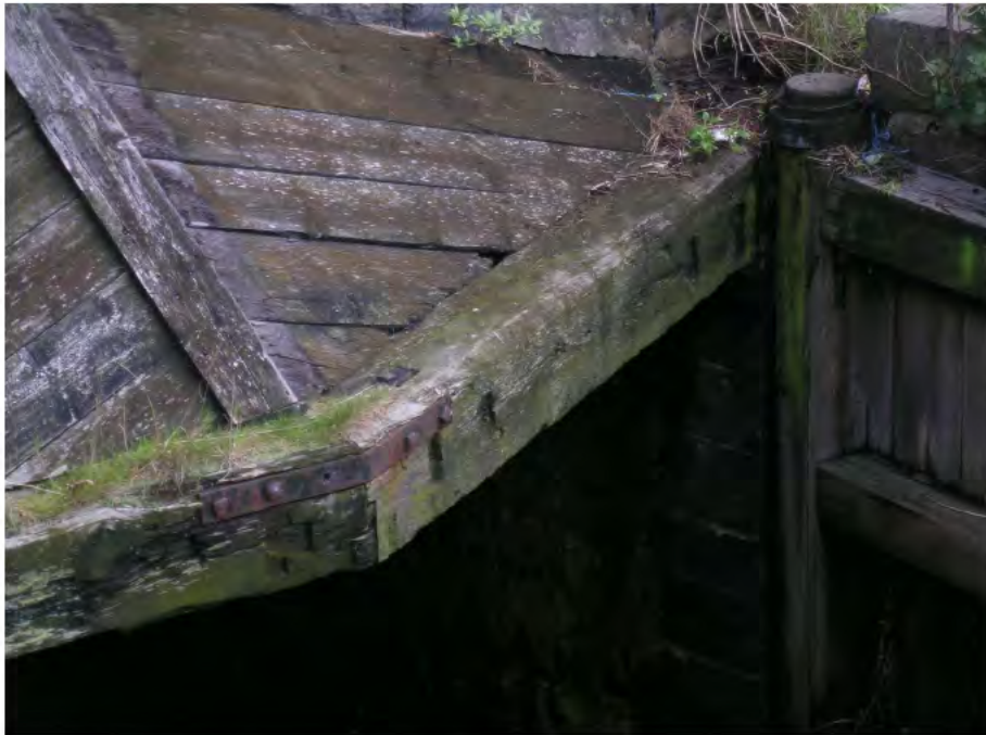
Plate 5: Close-up of Reused Oak Timber on Gate A
