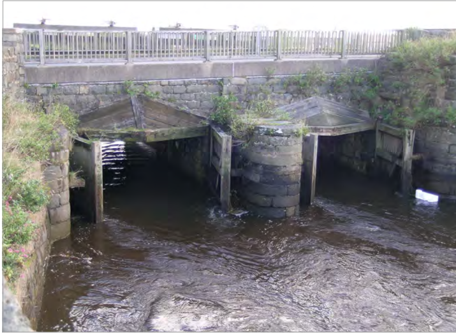
Plate 3: Close-up of Tidal Gates Open (View from Northwest)
