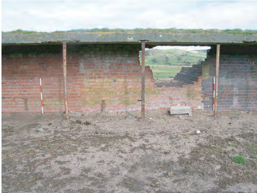
Fig. 14 Rifle Range butts. The central part of the covered walkway from the west showing the blocking between phases 1 and 2. Scales 1m long with 20cm divisions and 5m apart.
