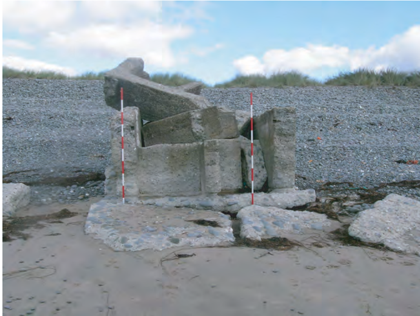
Fig. 20 Pillbox 270340. West side showing exposed interior and foundation plinth. Scales 2m long with 20cm divisions and 2m apart.
