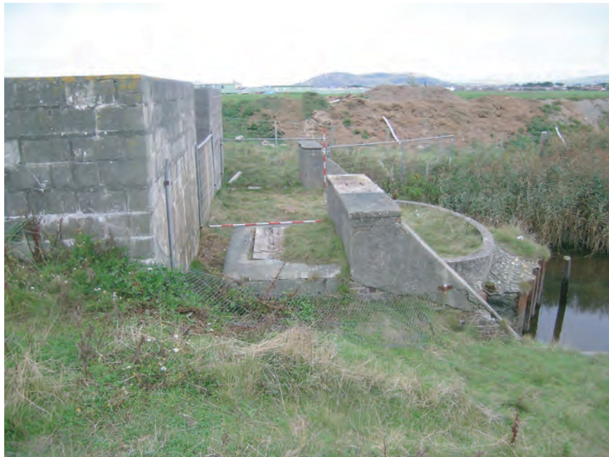
Fig. 5 Afon Dyffryn Gwyn tidal gate. The apron and access hatch of the 19th century tidal gate entrance. From the south. Scales 2m long with 20cm divisions.
