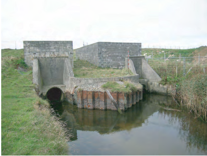
Fig. 4 Afon Dyffryn Gwyn tidal gate. The entrance to the outfall, the 19th century pipe inlet on the left. From the east. Scales 2m long with 20cm divisions.
