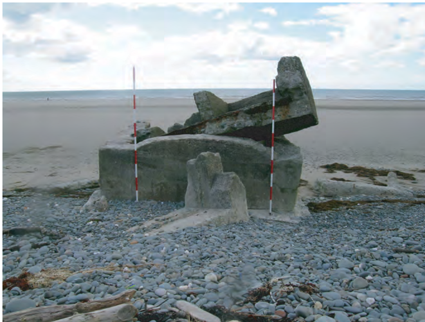
Fig. 21 Pillbox 270340. East side showing rear firing aperture (in fallen wall fragment) and exposed steel plate reinforcement for roof. Scales 2m long with 20cm divisions and 2m apart.
