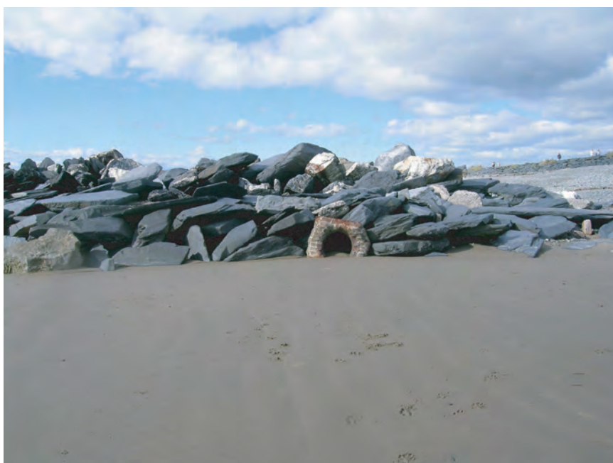
Fig. 7 Afon Dyffryn Gwyn beach outfall from the south. Remains of old outfall pipe incorporated in the rubble breakwater.
