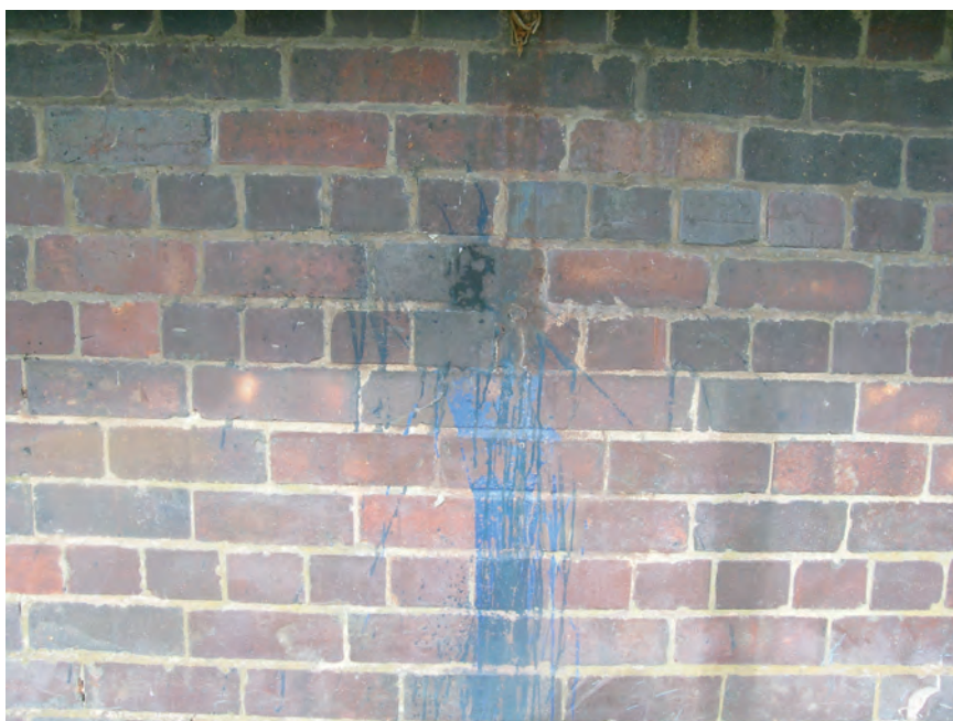
Fig. 12 Rifle Range butts. Bolt ends and stain of cast iron bracket on the rear wall of the Phase 1 part of the butts within the covered walkway.
