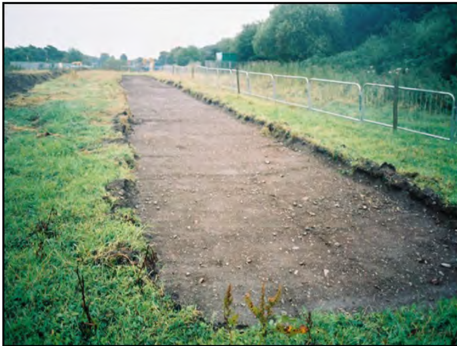
Plate 5: Topsoil Strip of Water Supply Pipe Route (Looking Southeast Towards the Compound)
