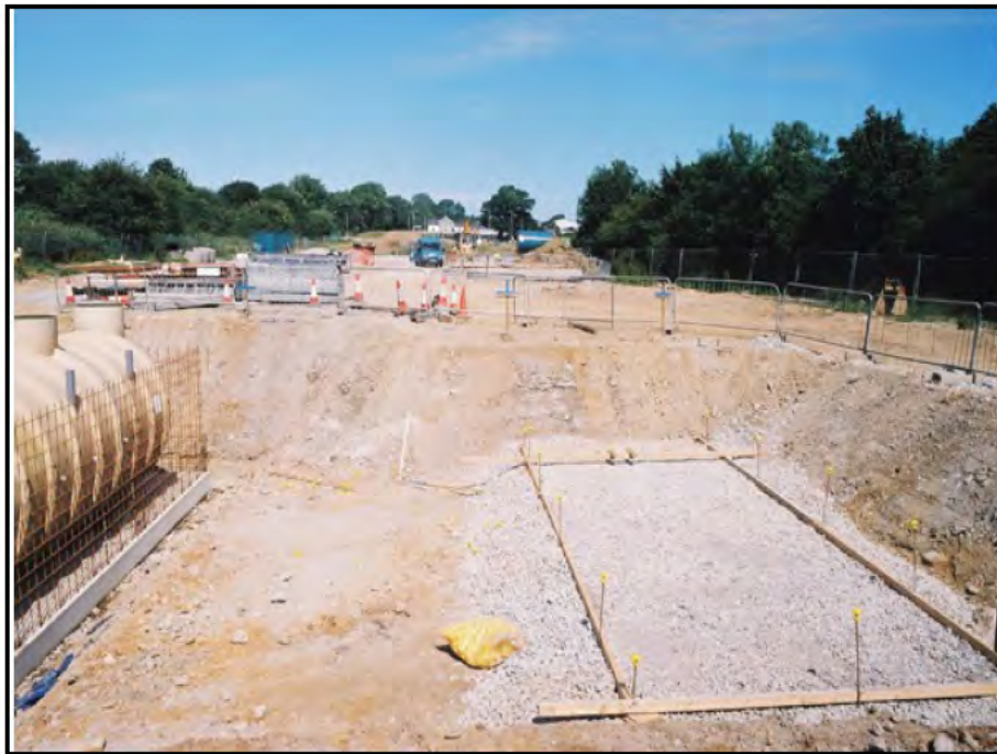
Plate 3: Odour Control Manhole Area Excavated
