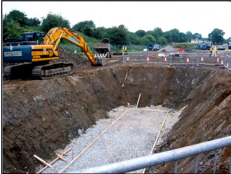
Plate 1: Excavation of Primary Settlement Tank
