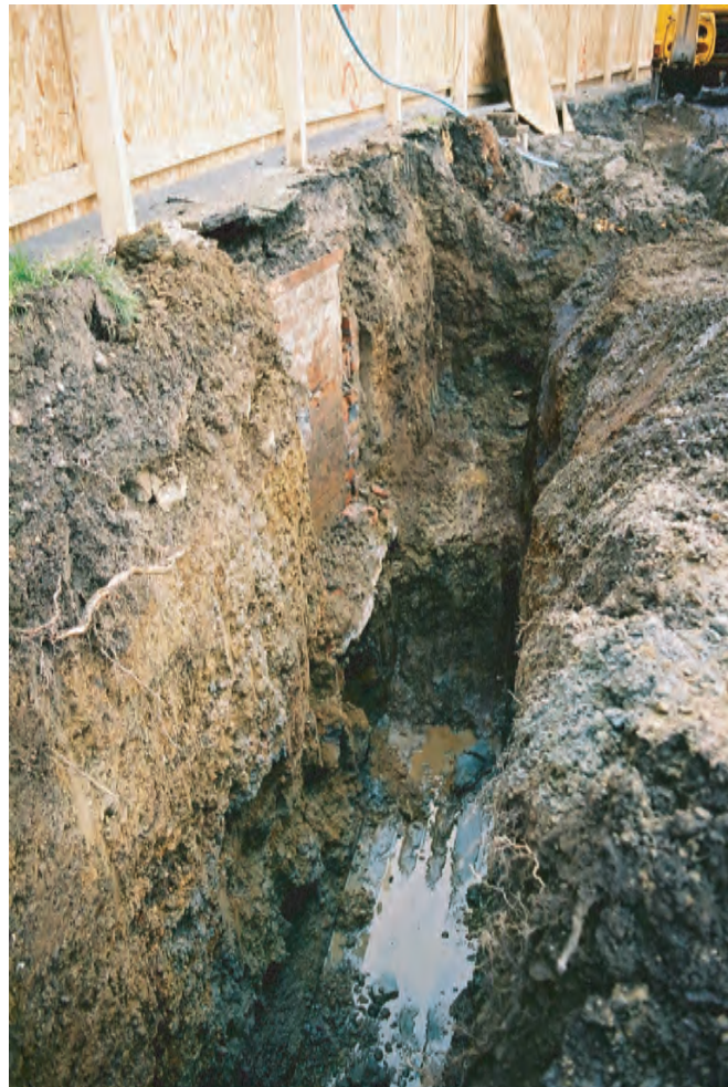
Bangor Bishop's Palace Archaeological Watching brief Fig. 4 Early 20th C sewer-cut beneath brick-built inspection chamber at the east edge of the site. From the north-west.
