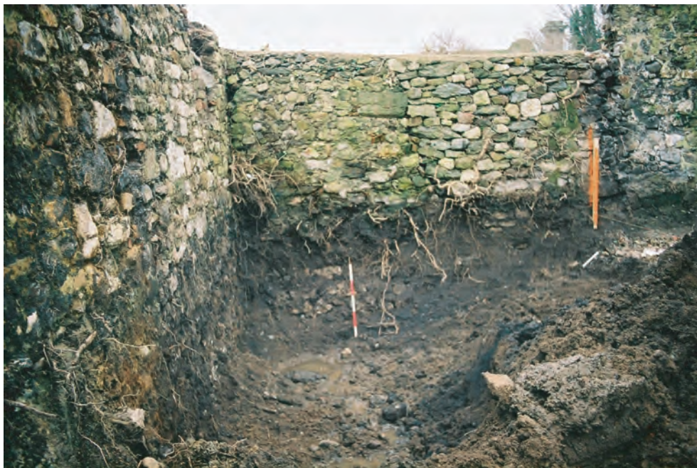
Regent House, Beaumaris Fig. 7 Blocked gap in west yard wall during excavation for sub-floor void. 1m scale
