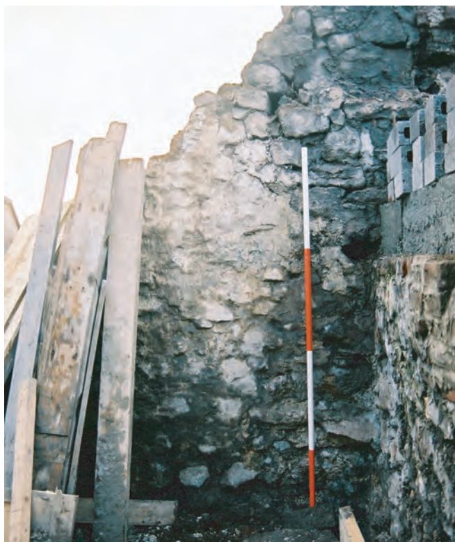
Regent House, Beaumaris Fig. 13 Interior gable of stable at west side after collapse of gable wall showing an earlier roof line of a single storey building. From the north-east. 1m scale.
