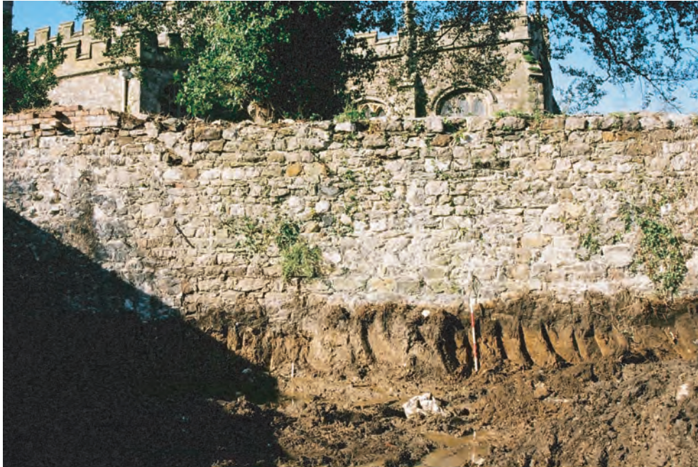
Regent House, Beaumaris Fig. 10 Churchyard retaining wall after excavation for new building footings showing exposed subsoil beneath base of wall. From the south-east. 1m scale.
