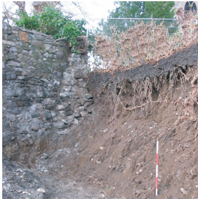
Regent House, Beaumaris Fig. 9 North-west corner of the yard after collapse of the churchyard wall, showing the bonded junction of the house yard and churchyard walls. From the east. 1m scale.
