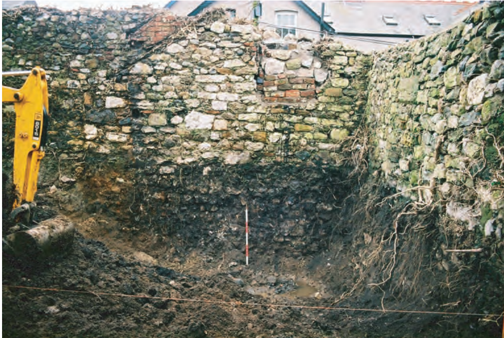
Regent House, Beaumaris Fig. 6 Outline of Smithy/Boilerhouse in south yard wall during excavation for sub-floor void. 1m scale
