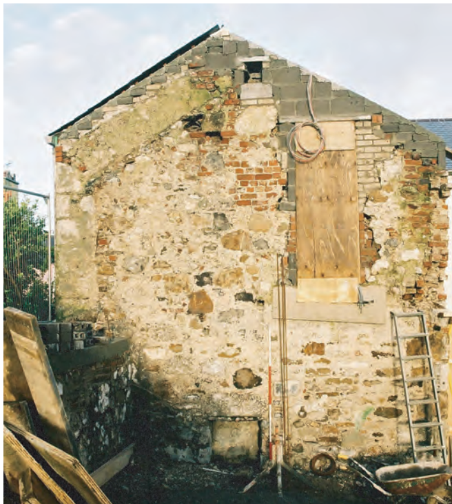
Regent House, Beaumaris Fig. 12 Interior of stable at east side showing blocked fireplace, line of removed roof and bonding with house wall. From the south-west. 1m scale.
